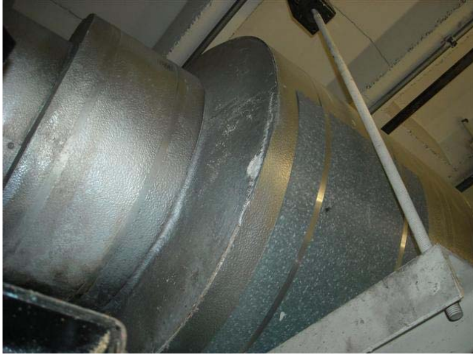
Building 1 Sample 58 - Generator Insulation Wrap
