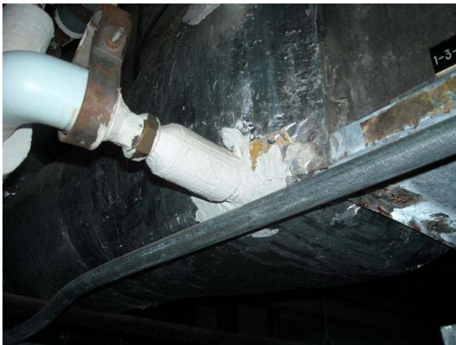
Building 1 Sample 165 – White Duct Mastic
