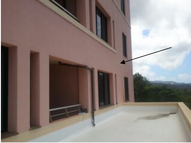
Exterior Wall – RACM - Cementitious Plaster
