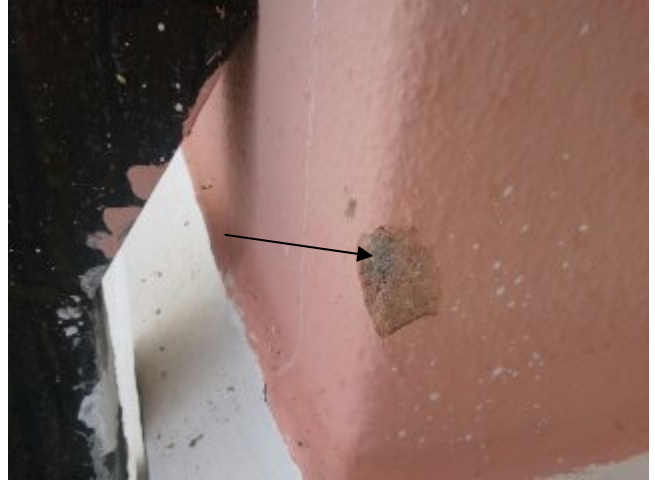
Exterior Wall – RACM - Cementitious Plaster
