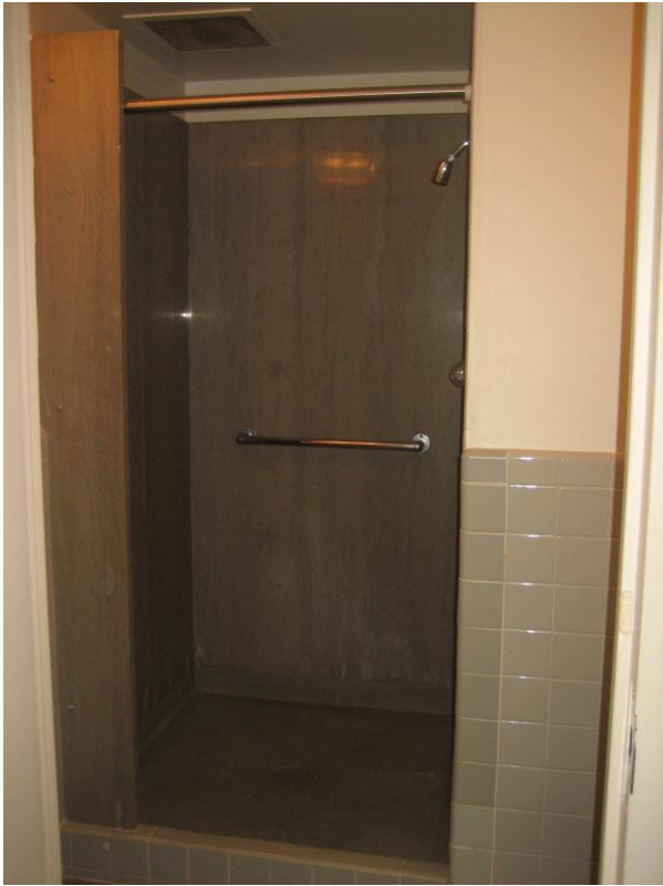
6B114 Remove shower, approx. 40 feet of pipe to T, hot and cold.
