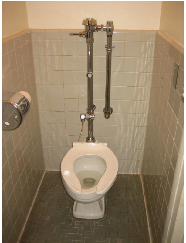
6B114 Remove toilet, approx. 30 feet of pipe to T
