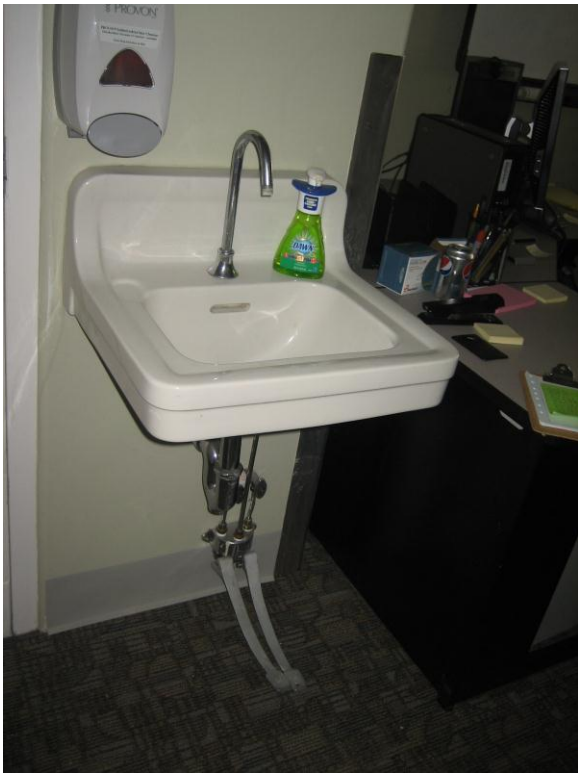
8C135 Remove sink, approx. 30 feet of pipe to T, hot and cold.
