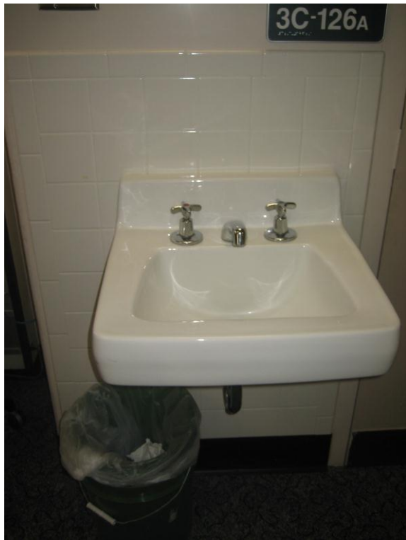
3C126 Remove sink #1, approx. 20 feet of pipe to T, hot and cold.
