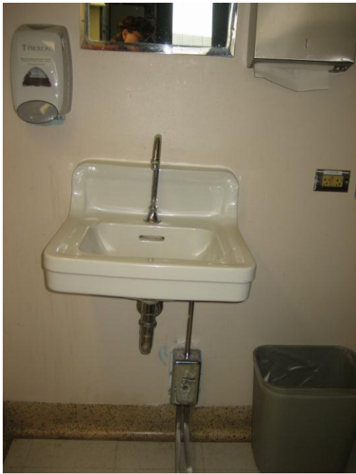
7B106 Remove sink, approx. 20 feet of pipe to T, hot and cold.
