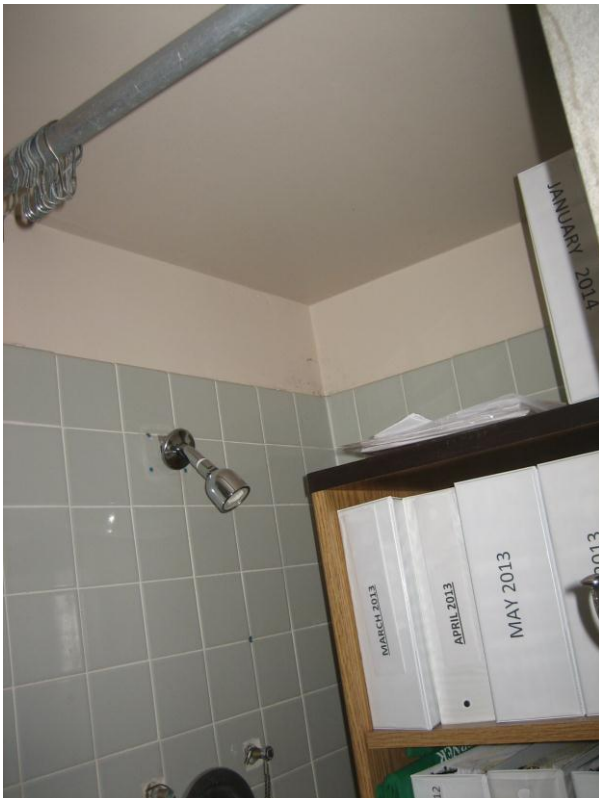
7B106A Remove shower, approx. 30 feet of pipe to T, hot and cold.
