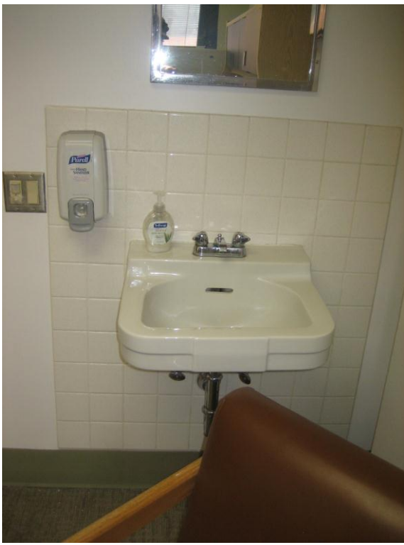
8C125 Remove sink, approx. 20 feet of pipe to T, hot and cold.
