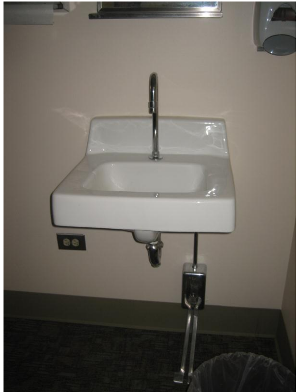
2D114 Remove sink, approx. 20 feet of pipe to T, hot and cold.
