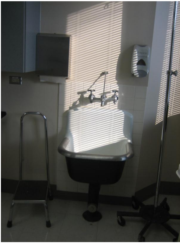
2D104A Remove sink, approx. 40 feet of pipe to T, hot and cold.
