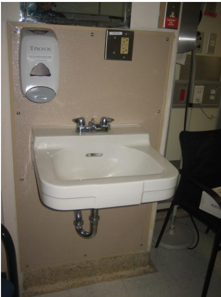
6C124 Remove sink, approx. 20 feet of pipe to T, hot and cold.
