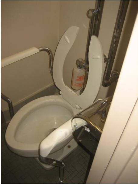
6B106 Remove toilet, approx. 20 feet of pipe to T
