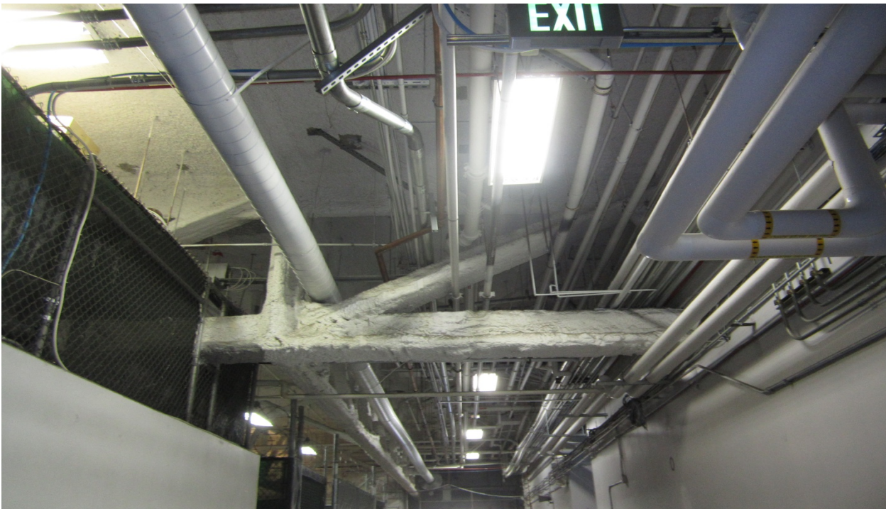
PHOTO 1: Fireproofing on structural beams and decking. Wrapped pipe insulation. Concrete floors and walls.
