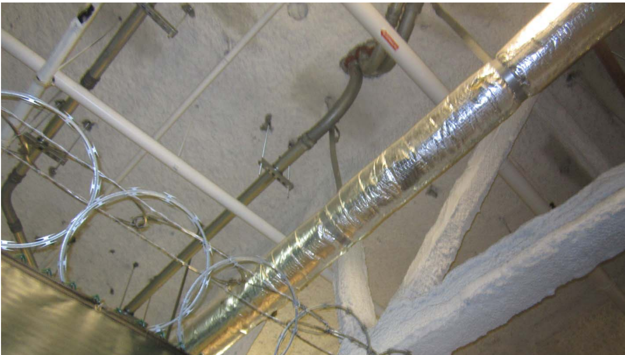
PHOTO 2: Fireproofing on structural beams and decking. Wrapped pipe insulation. Concrete floors and walls.
