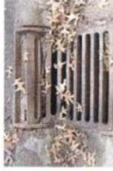
Sewer Inlet Deterioration 004
