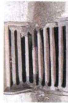
Sewer Inlet Deterioration 012
