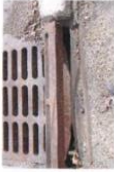
Sewer Inlet Deterioration 002
