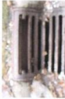
Sewer Inlet Deterioration 007
