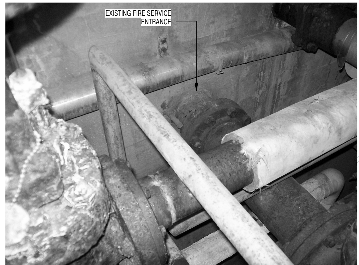
1 EXISTING FIRE SERVICE ENTRANCE Scale: NOT TO SCALE
