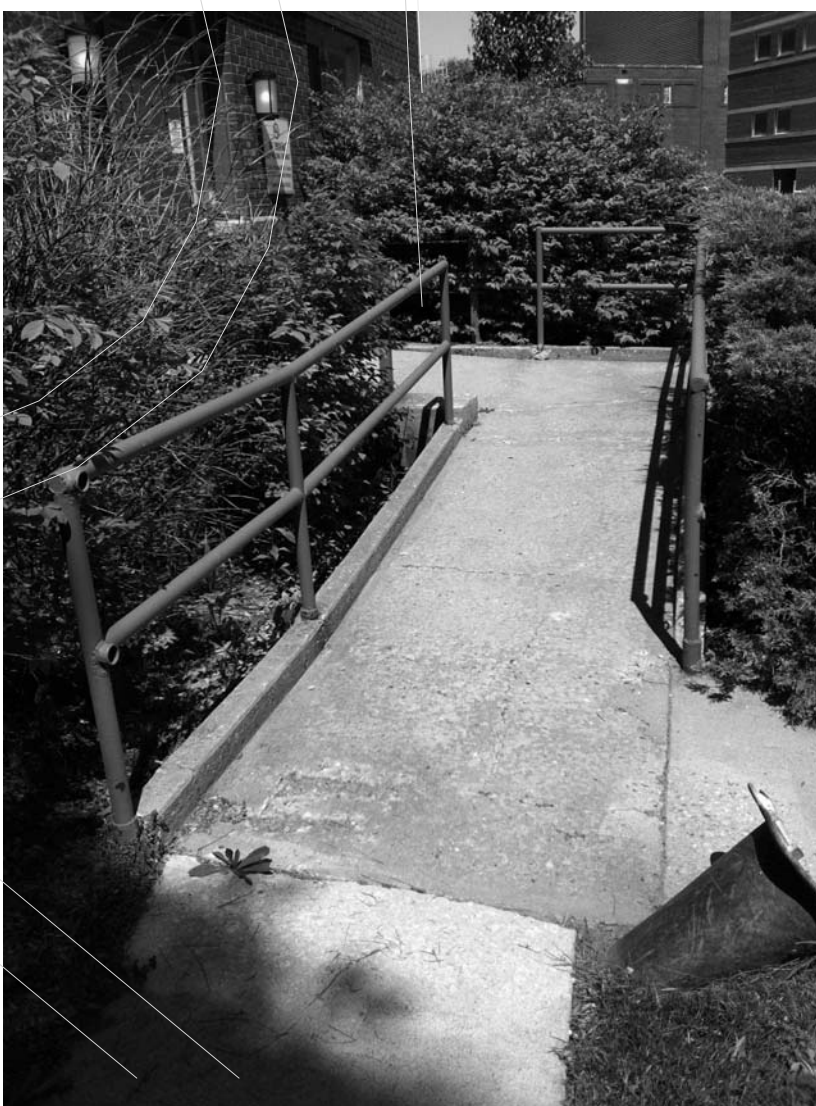
CONCRETE RAMP TO BE REMOVED. REF.: DEMOLITION NOTE D.10 AND 1/D010
