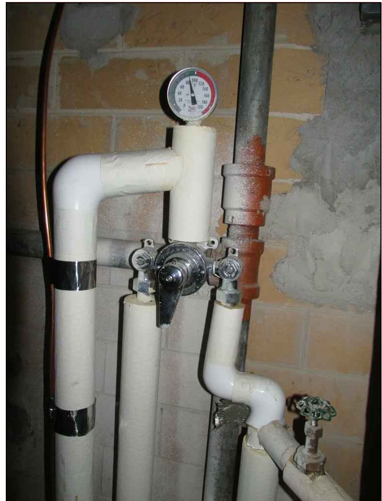
TYPICAL MIXING VALVE DISCONNECT AND REMOVE VALVE. DISCONTINUE COLD WATER FEED BACK TO MAIN FEED PIPE. REMOVE TEE FROM MAIN FEED PIPING AND INSTALL COUPLING. DISCONNECT HOT WATER SUPPLY TO VALVE AND WARM WATER SUPPLY TO FIXTURES AND INSTALL 1/4 TURN BALL VALVE AND CONNECT THE TWO PIPES SO THAT HOT WATER IS SUPPLIED TO THE FIXTURES.
