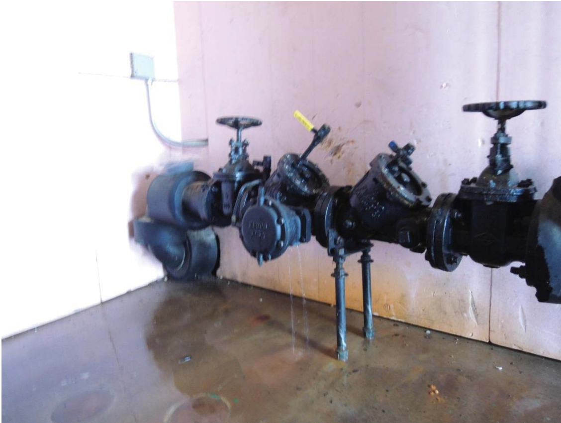
Backflow Preventer to be removed and replaced
