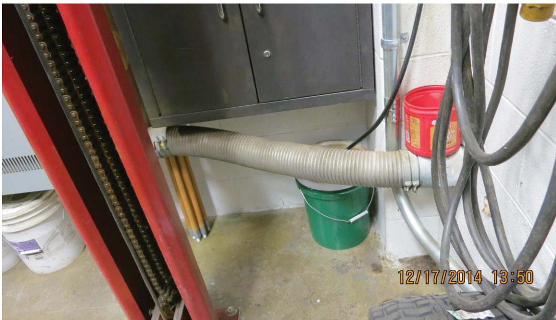
Plastic Flex Conduit to be removed and replaced with EMT
