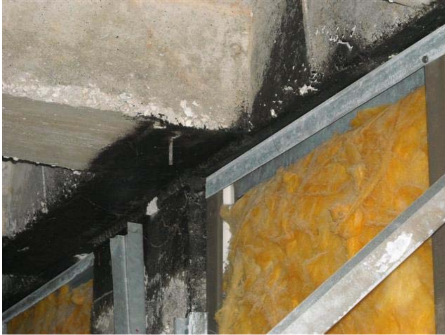
Building 1 Sample 76 - Black Waterproofing – Exterior Walls
