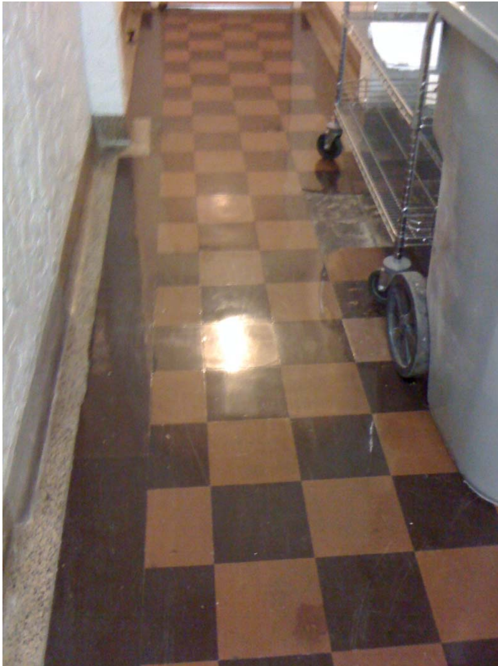
Building 20 Sample 44 Floor - 9" x 9" Burgundy Floor Tile Sample 47 - 9" x 9" Tan Floor Tile and Mastic
