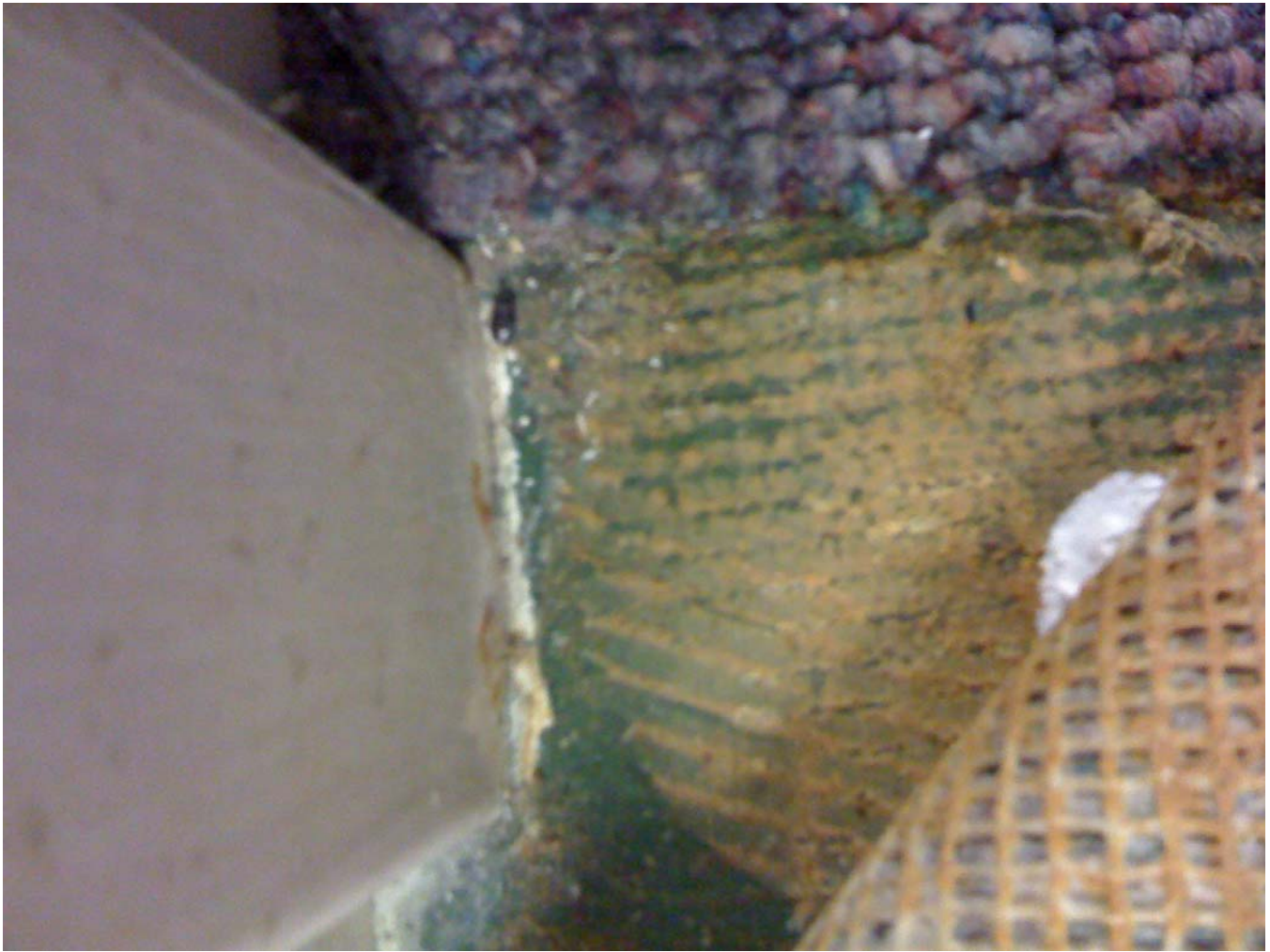
Building 20 Sample 50 Floor - 9" x 9" Green Floor Tile
