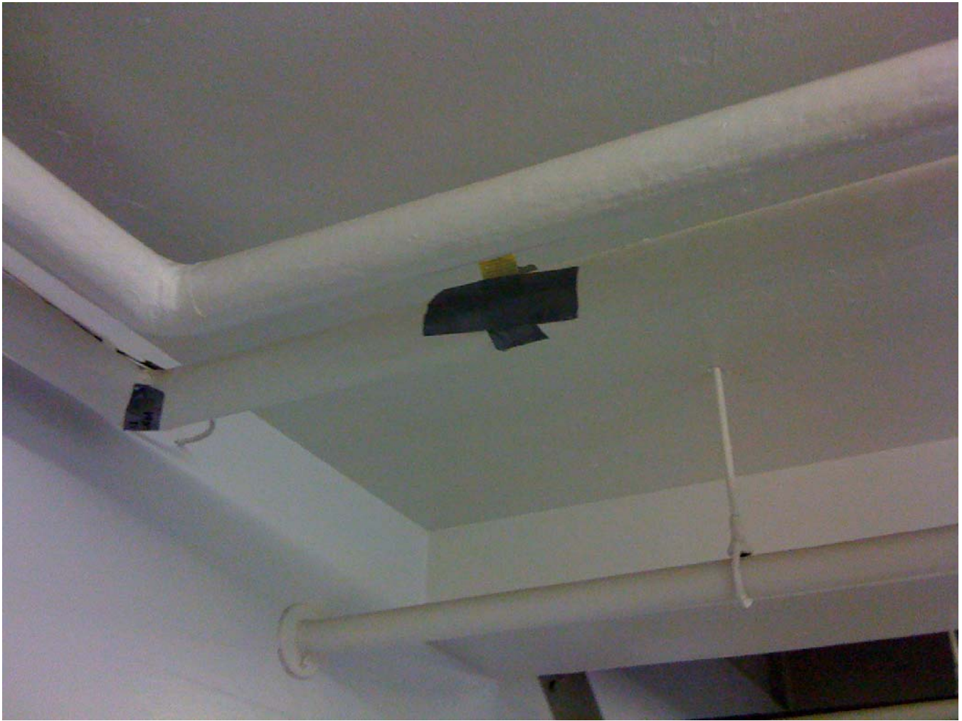
Building 20 Sample 72 – Pipefitting Insulation Sample 75 – Pipe Insulation
