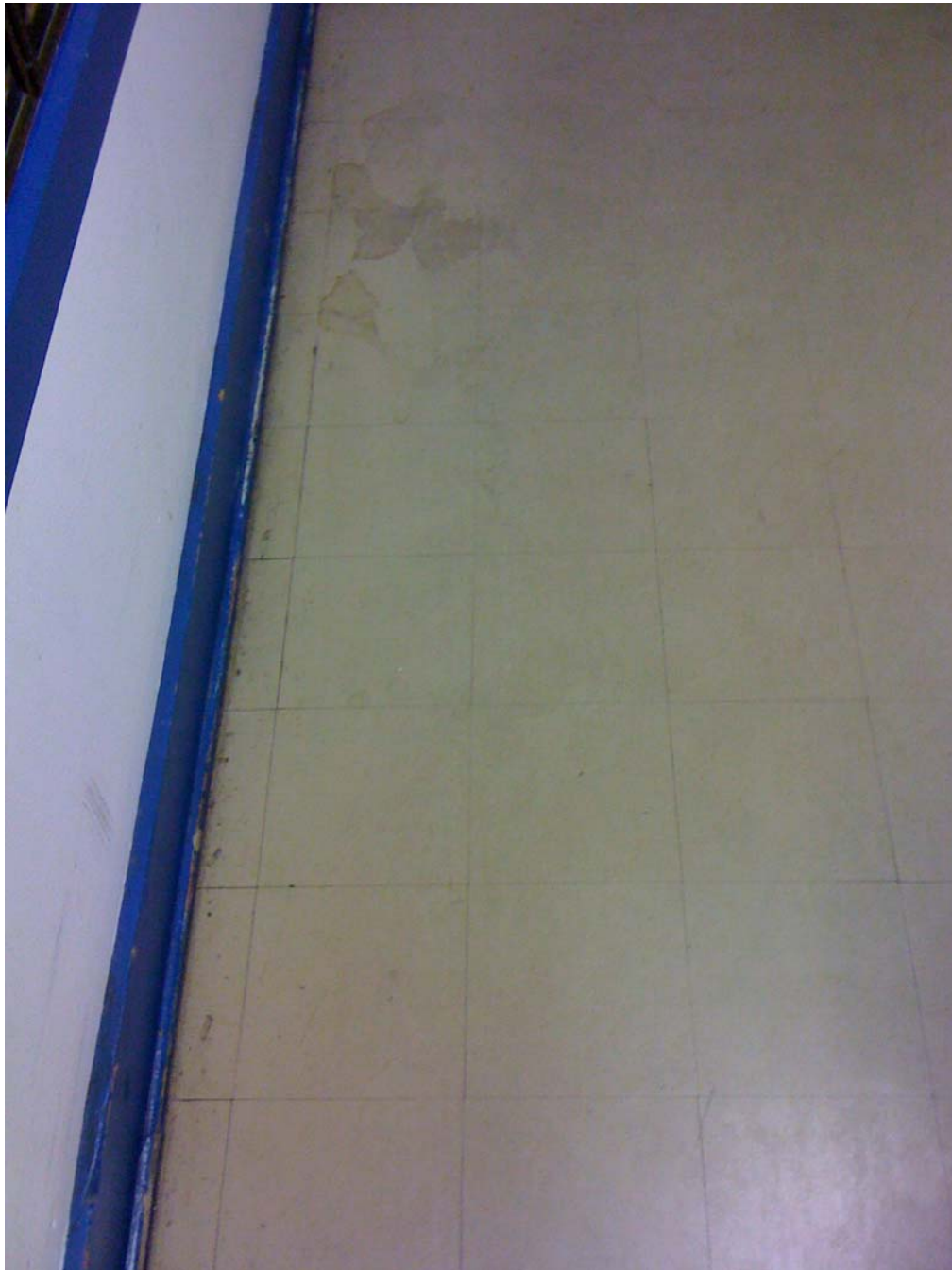
Building 20 Sample 32 Floor – 9" x 9" Light Brown Floor Tile and Mastic
