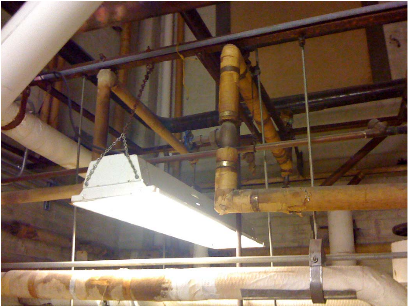
Building 37 Sample 137 - Air Cell-Like Pipe Insulation
