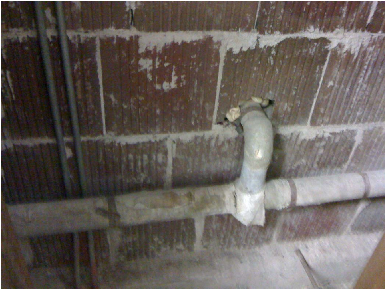
Building 37 Sample 110 - Pipefitting Insulation
