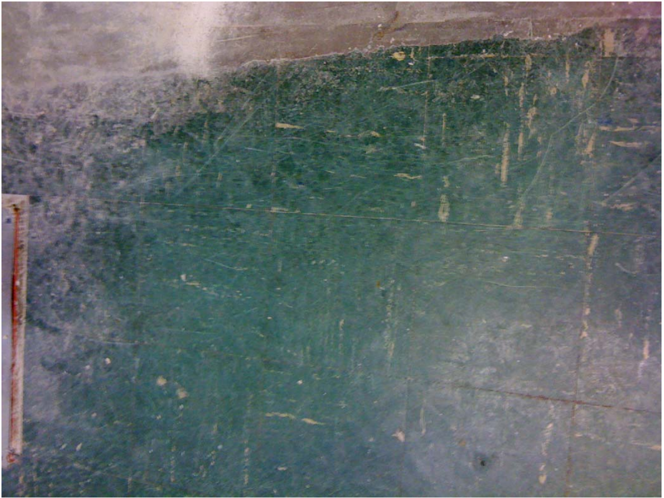
Building 37 Sample 131 Floor - 9"x9" Green Floor Tile Sample 132 Mastic - Black Mastic
