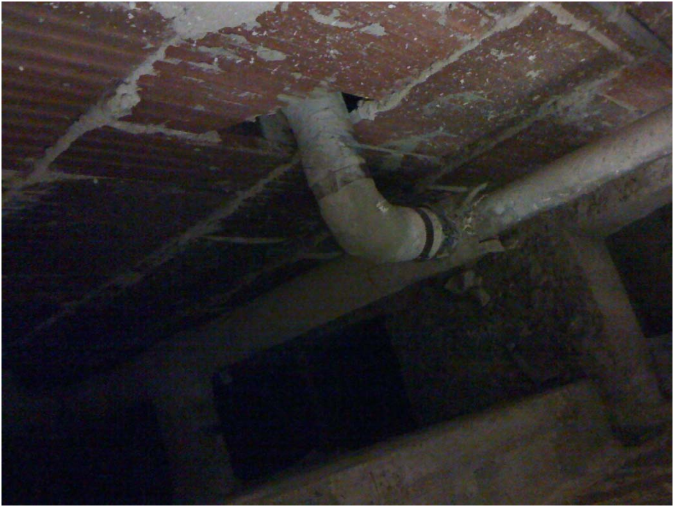
Building 37 Sample 107 – Pipe Insulation
