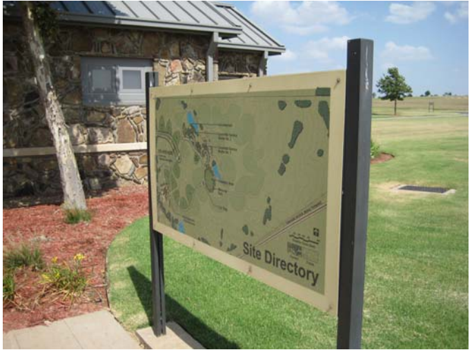
Figure 8: Existing site directory sign to be salvaged, posts repainted, and reinstalled
