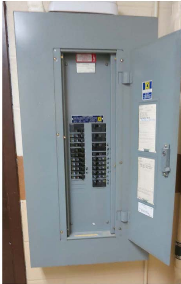
Lower Level Control Panel – Panel Installed Upside Down
