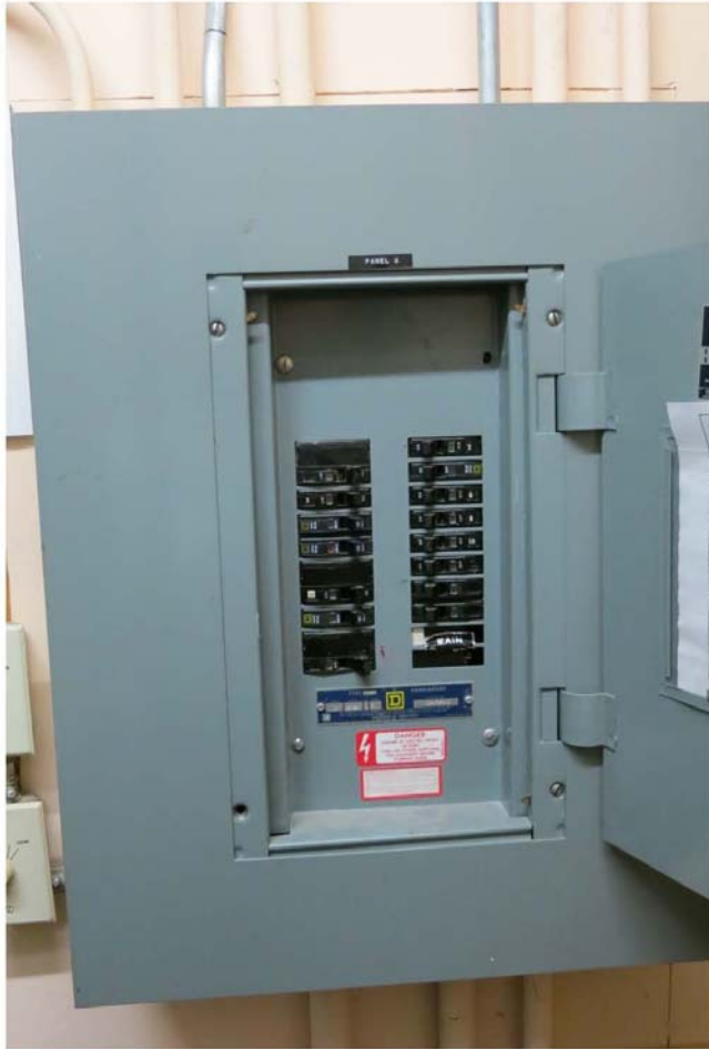
Main Level Control Panel – Main Switch Improperly Placed
