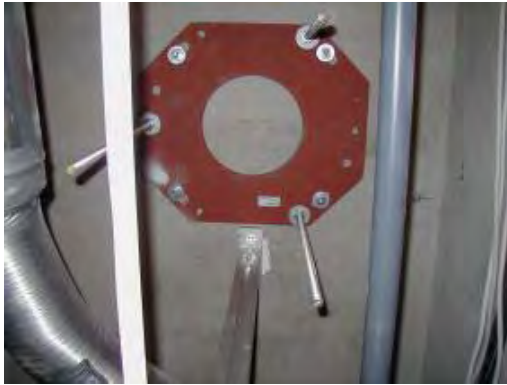
Figure 3-49 Ceiling Plate with Installed Threaded Bolts
