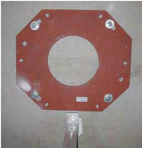
Figure 3-48 Ceiling Plate Installed
