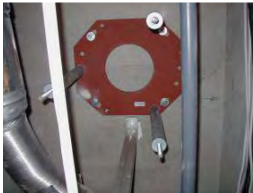
Figure 3-50 Ceiling Plate with Installed Tubes
