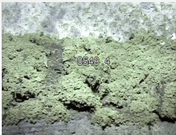
Top of 8" Liner
