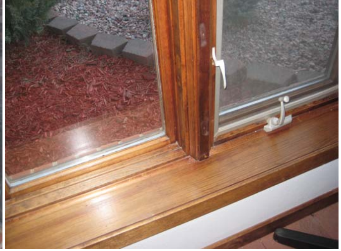
Figure 16: Casement window (typical), interior view
