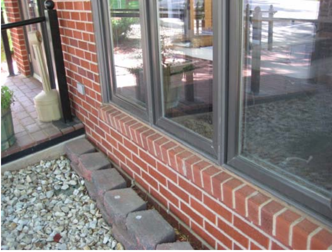
Figure 15: Admin casement window (typical), exterior view
