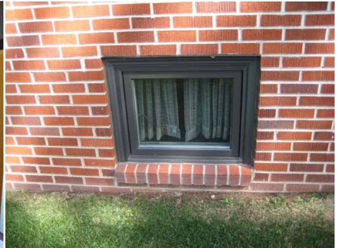
Figure 18: Basement casement window (typical)
