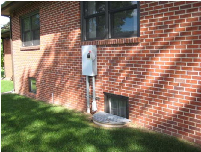
Figure 19: Basement window for new window well
