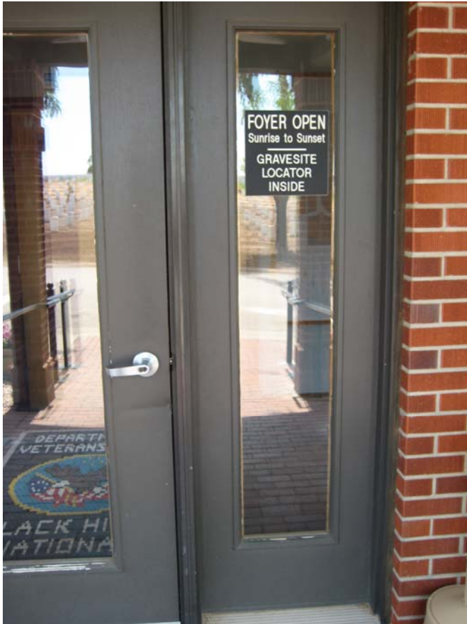
Figure 11: Admin front entrance door and sidelite
