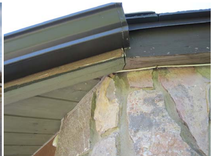
Figure 10: Shelter gutter, beginning of run; and soffit
