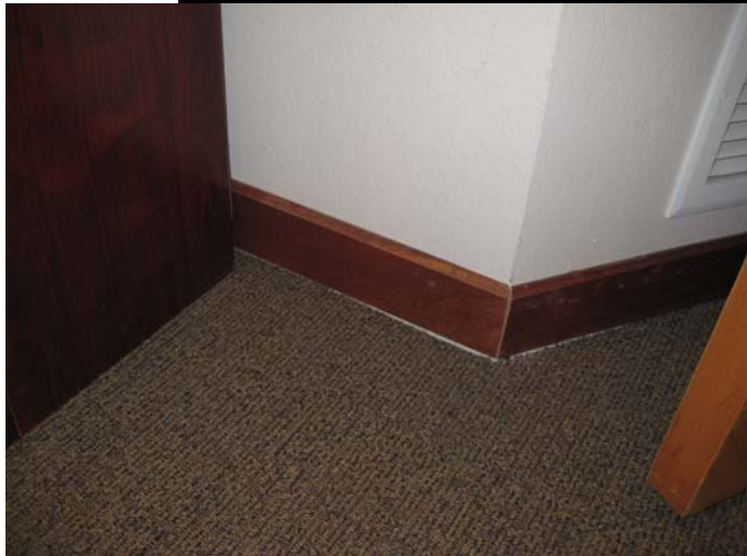
Figure 21: Baseboards and interior painting (typical)
