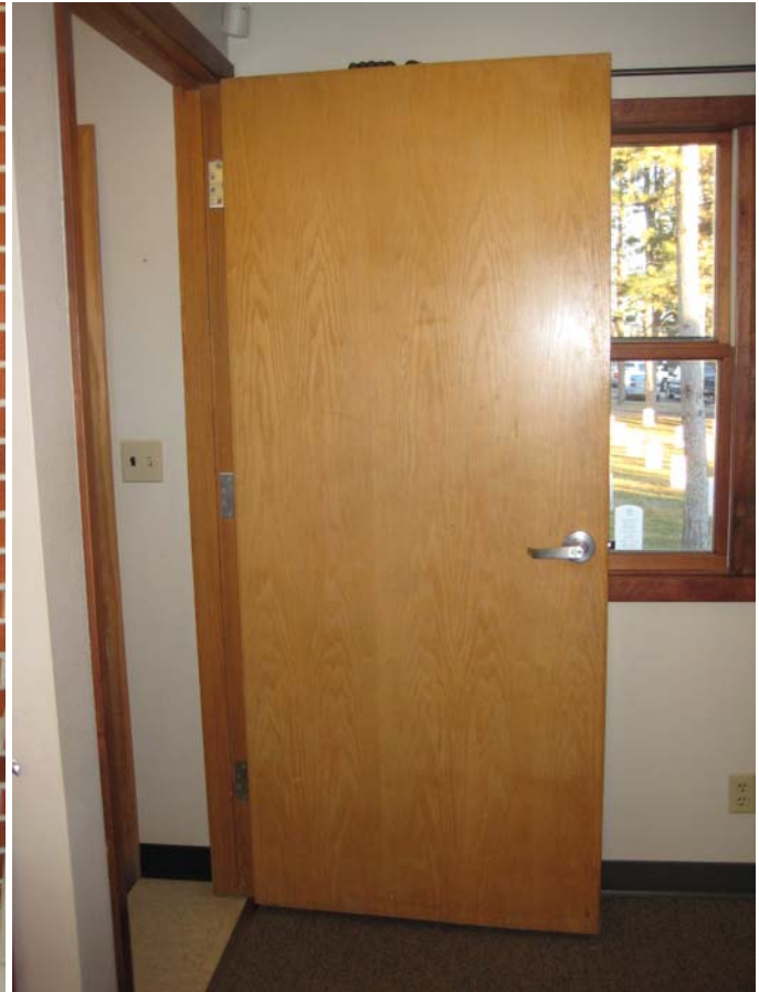
Figure 12: Interior wood door (typical)
