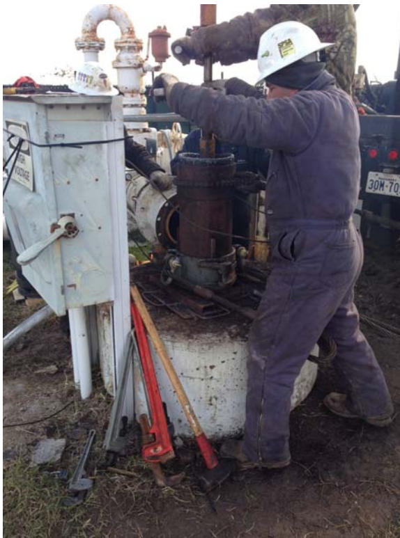
Figure 2: Pulling the pump
