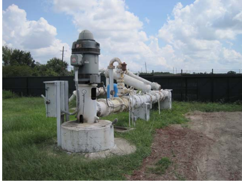
Figure 1: Well head and pump motor
