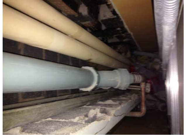
Figure 2: Representative view of pipe enclosure in area previously abated, indicating that in renovated areas, ACM pipe insulation was also abated within the enclosures.
