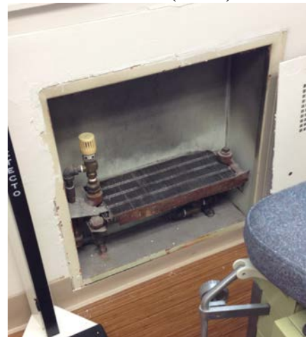
Figure 4: Representative view of recessed radiator enclosure with asbestos containing transite backing board with asbestos caulking. Metal cover plate does not contain lead paint in excess of 1.0 mg/cm 2 .
