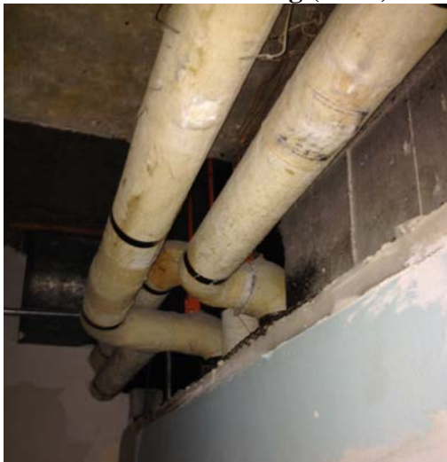
Figure 3: Representative view of asbestos containing pipe insulation above drop ceiling.
