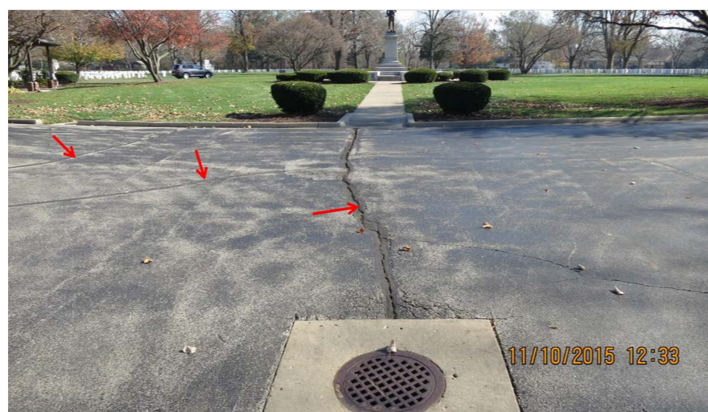
EXAMPLE OF A PAVEMENT CRACKS TO BE REPAIRED/PATCHED
