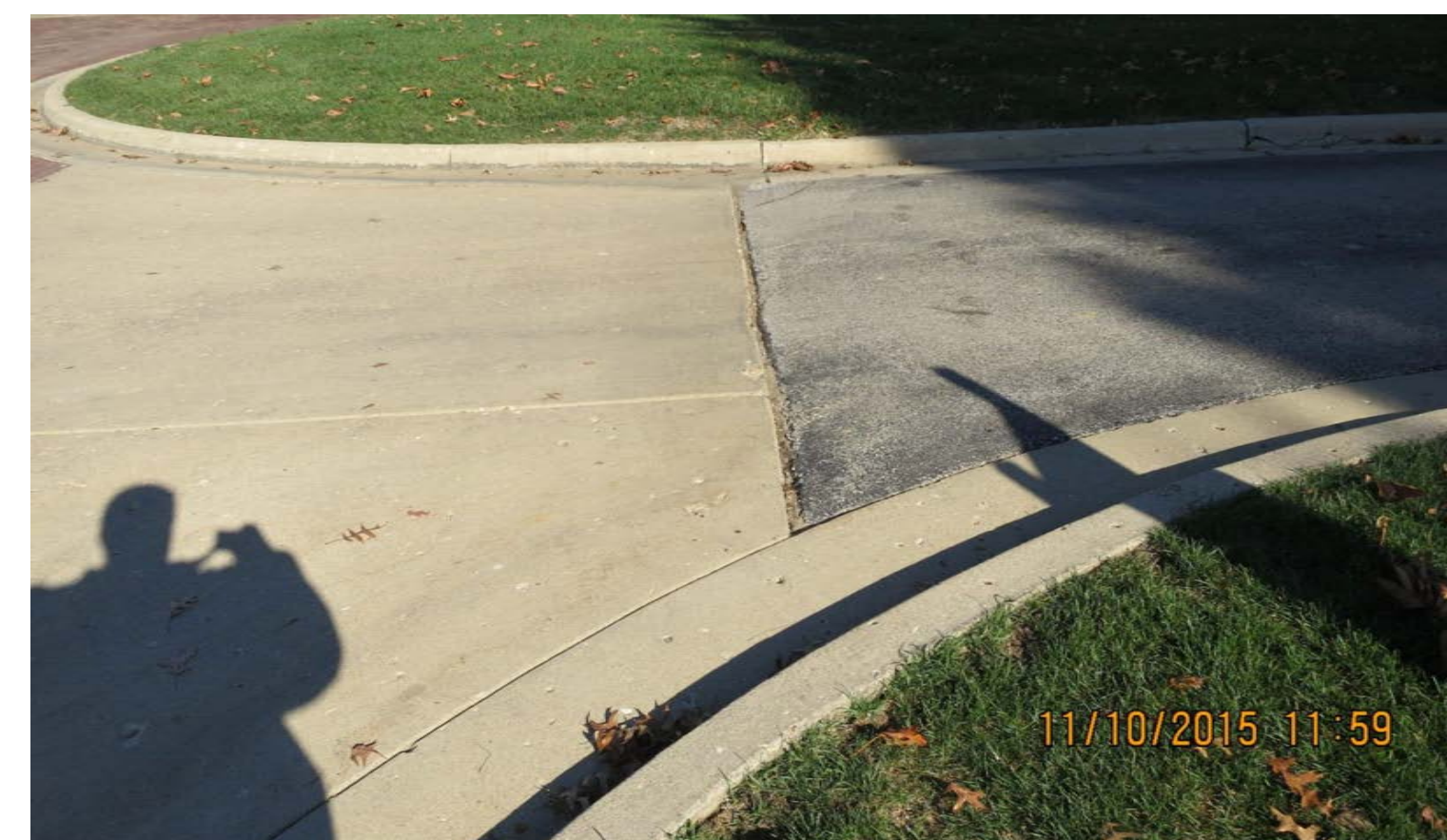
EXAMPLE OF A PAVEMENT SEAM BUTTING CONCRETE TO BE REPAIRED/PATCHED (CONCRETE TO REMAIN UNTOUCHED)
