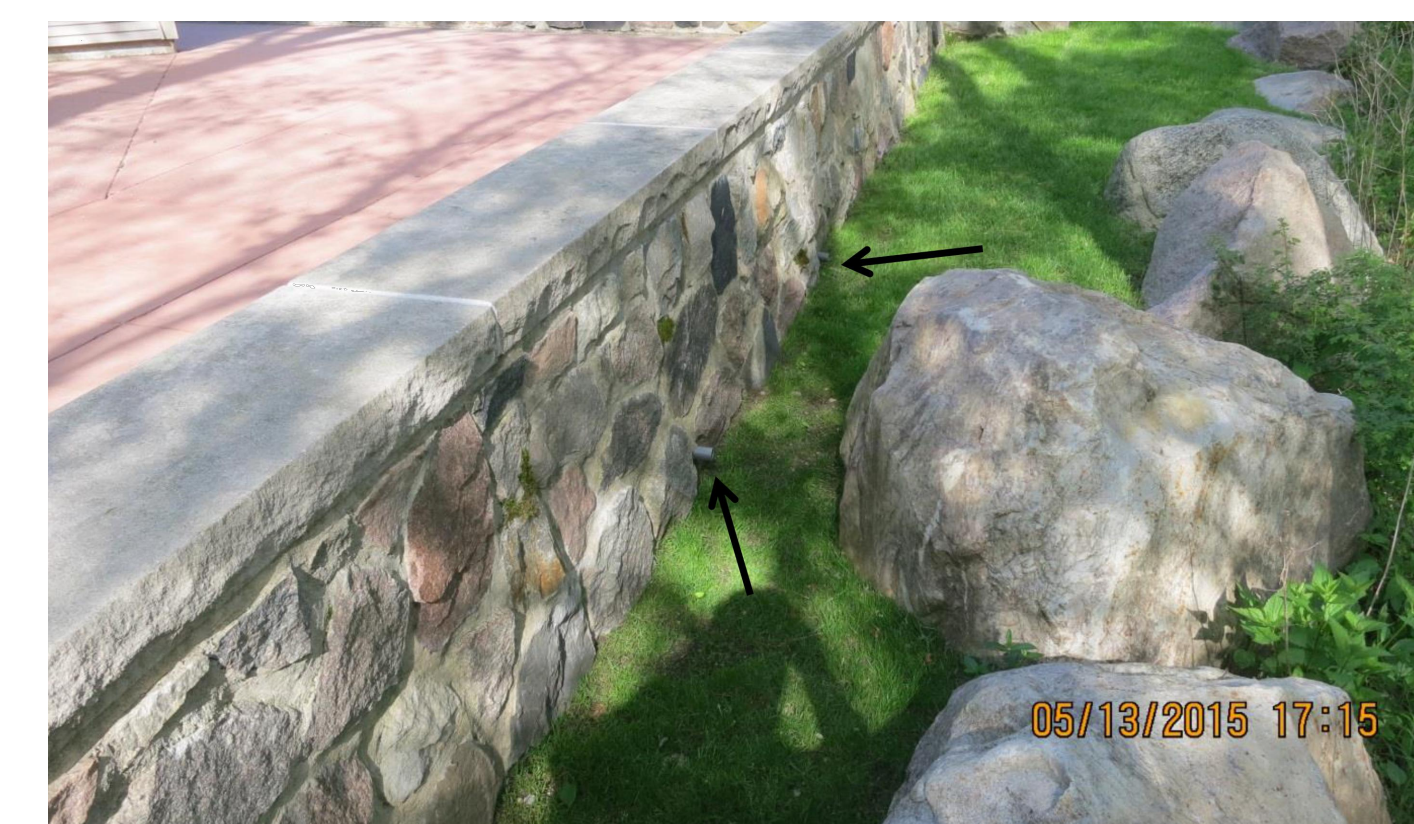
EXAMPLE OF WEEP HOLES TO BE REPLACED WITH 4" PVC PIPE
