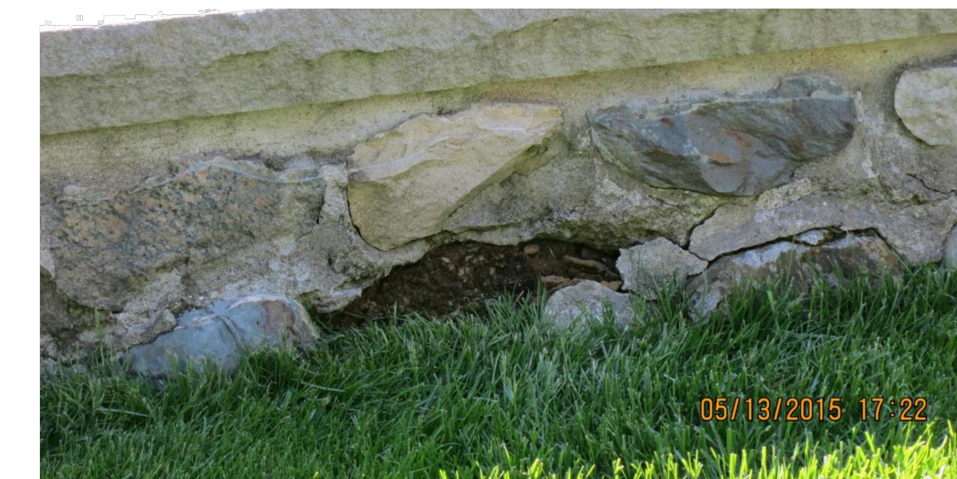
EXAMPLE OF MISSING STONES NEEDING REPLACED AND LOOSE/CRACKED MORTAR JOINT REQUIRE TUCKPOINTING
