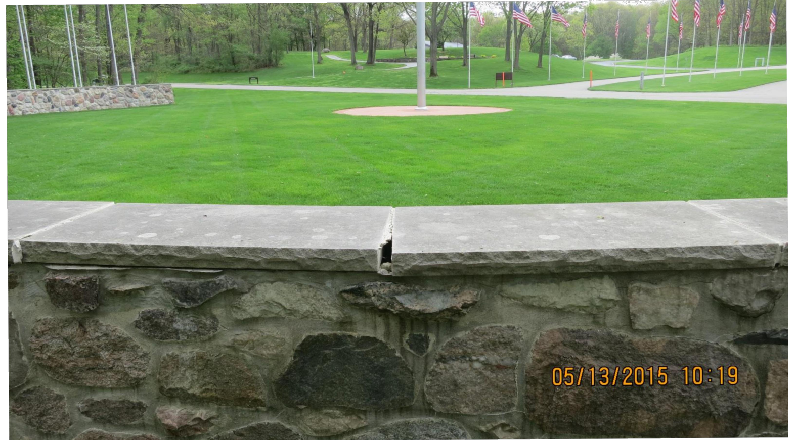
EXAMPLE OF LIMESTONE CAP REQUIRE RESETTING AND JOINT RESEALING (REMOVE OLD SEALANT)
