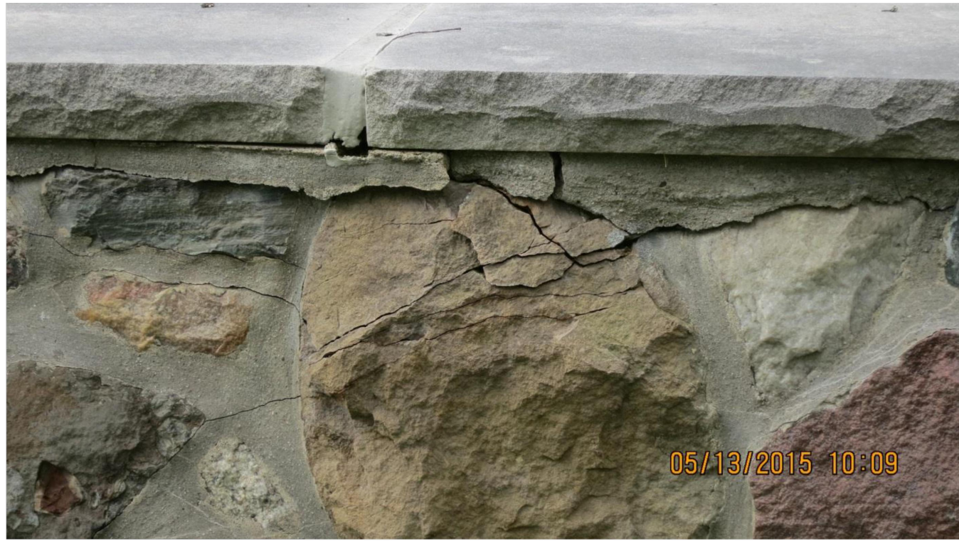
EXAMPLE OF BROKEN STONE TO BE REPLACED, LIMESTONE CAP TO BE RESET AND JOINT TO BE RESEALED (REMOVE OLD SEALANT)
