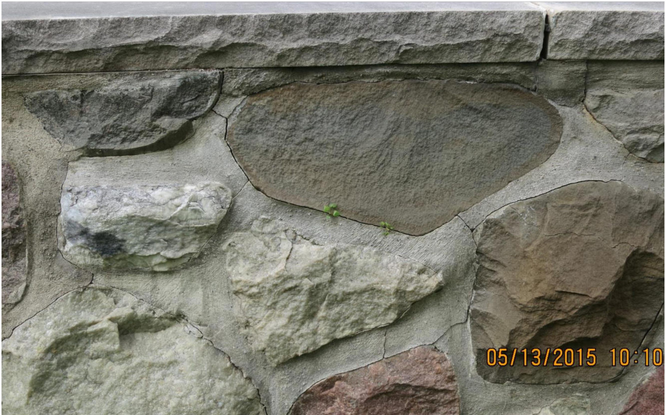
EXAMPLES OF CRACKED MORTAR JOINT REQUIRE TUCK POINTING AND LIMESTONE CAP REQUIRE JOINT RESEALING (REMOVE OLD SEALANT)
