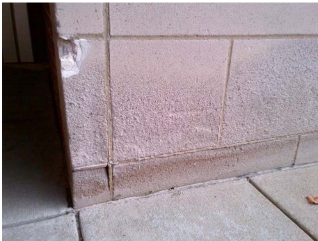
Figure 1.12 Building 1 Elevation 49 Cast Stone Façade Salt Damage
