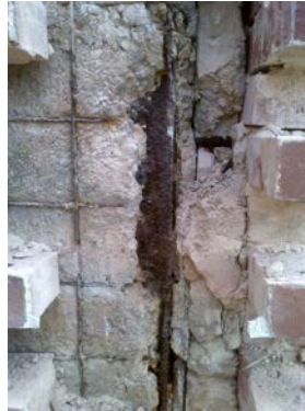
Figure 1.12 Building 1 Elevation 49 Cast Stone Façade Salt Damage
