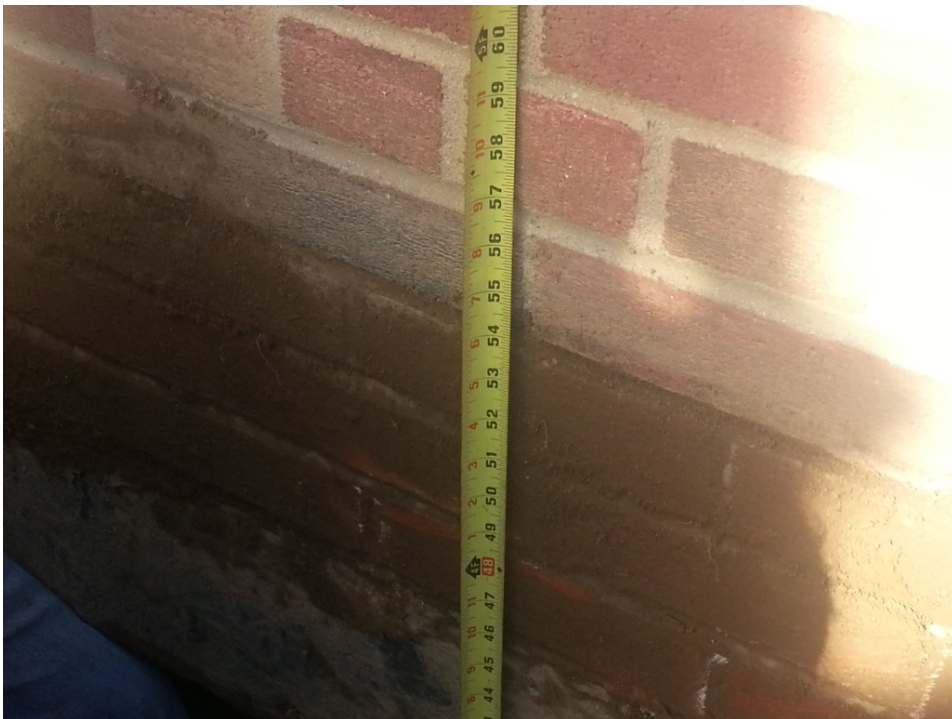
TP-1: Top of Foundation and Soil Line
