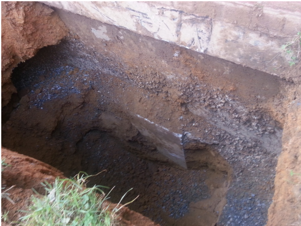
TP-3: Concrete Foundation with Concrete Encountered Below Prevailing Foundation
