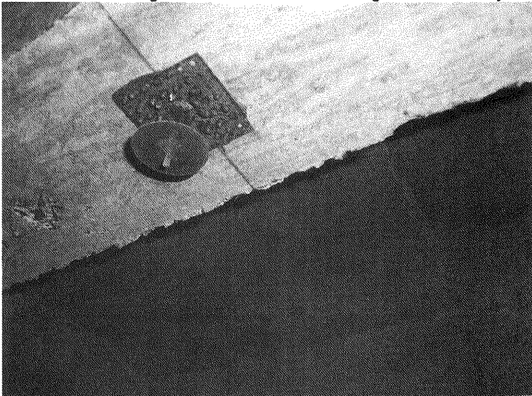
Glue for spike hangers attached to concrete ceiling – 3% Chrysotile
