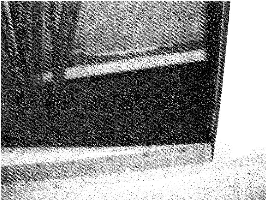
Glue Pucks on Ceiling associated with 1'x1' Ceiling Tiles – 3% Chrysotile
