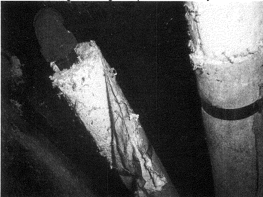
Significantly Damaged MAG Pipe Insulation above drop ceilings – Chrysotile 35%
