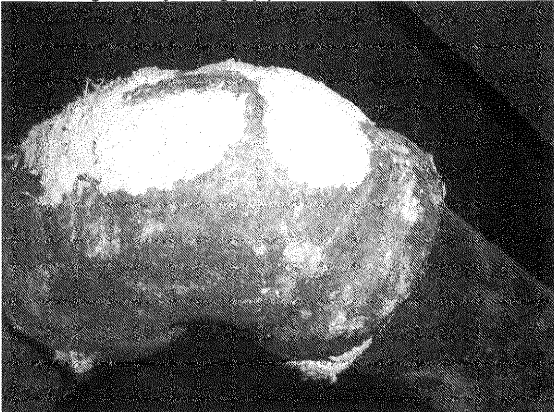
Room 118A – Poorly abated pipe insulation fittings
