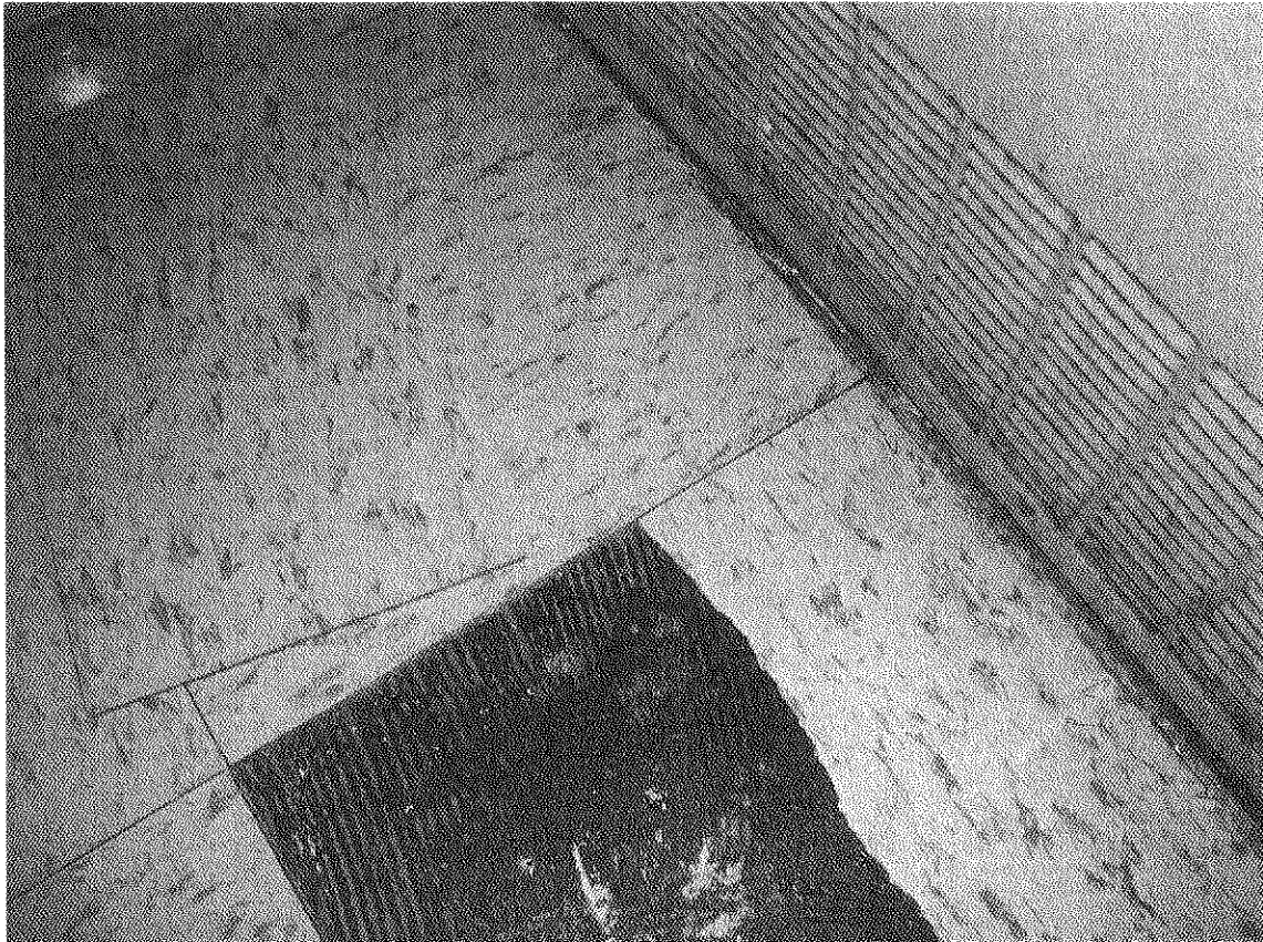
Room 227A – 12"x12" white w/ gold floor tile and mastic
