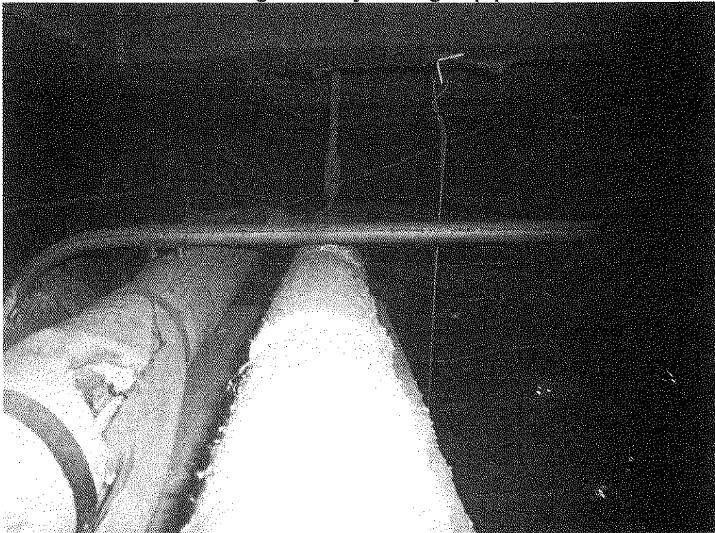
Room 130 – Asbestos Pipe Insulation significantly damaged
