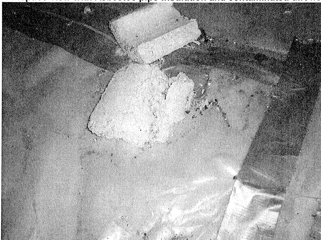
Crawlspace – asbestos pipe insulation debris on poly covering parts of the dirt floor – 35% asbestos
