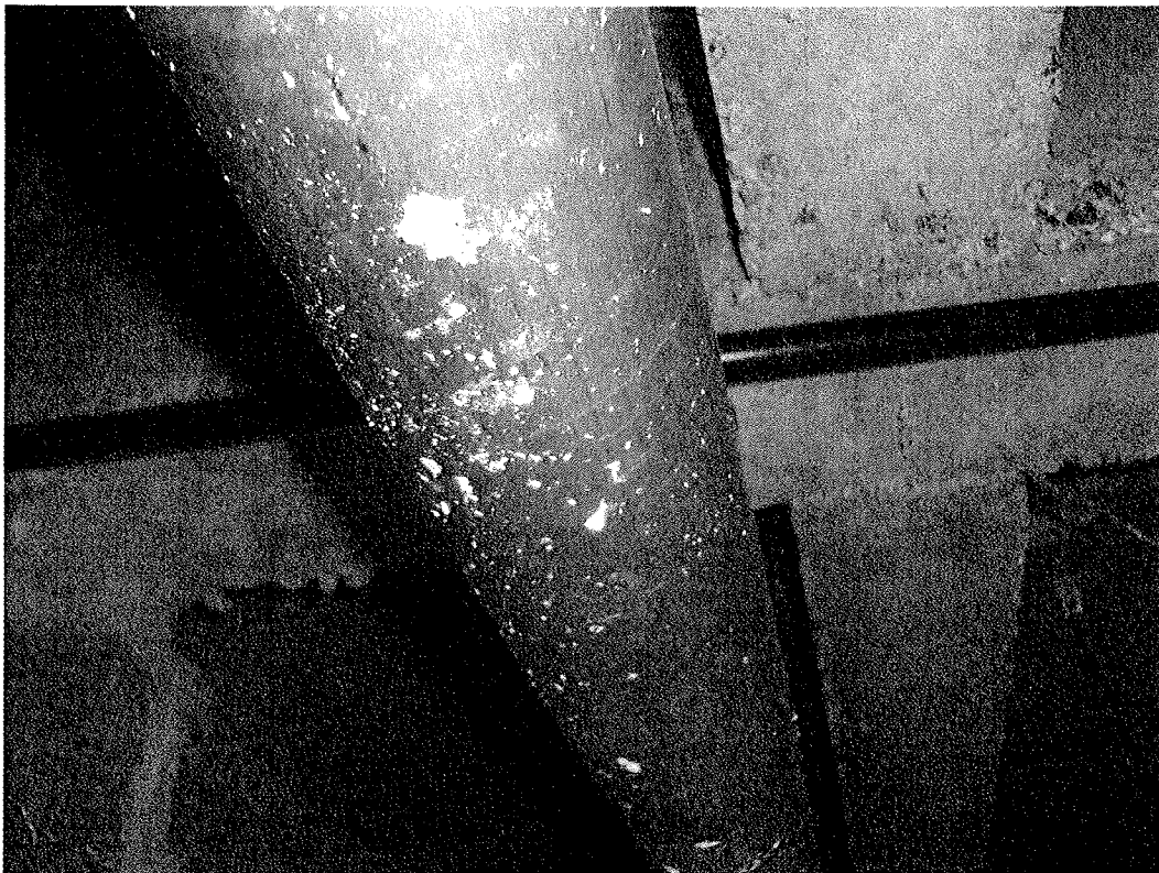
Room 123 – Asbestos Pipe Insulation residue/debris on abated pipe
