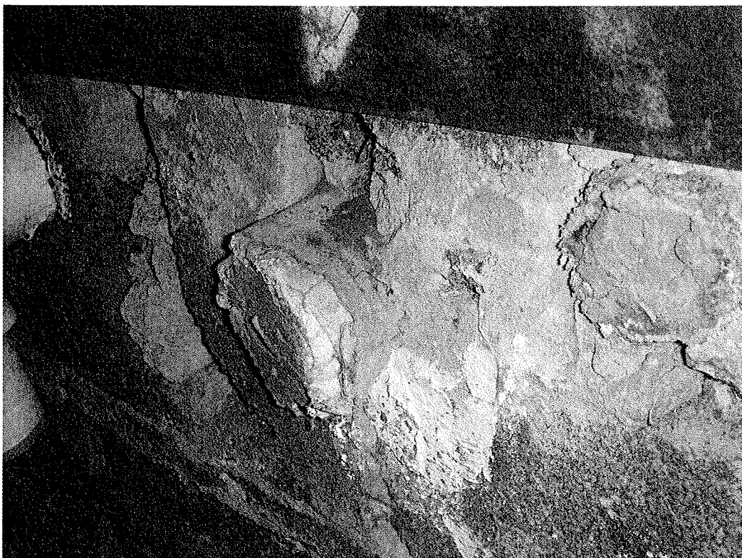
Chase 125E - Asbestos Pipe Insulation with exposed and mortared ends
