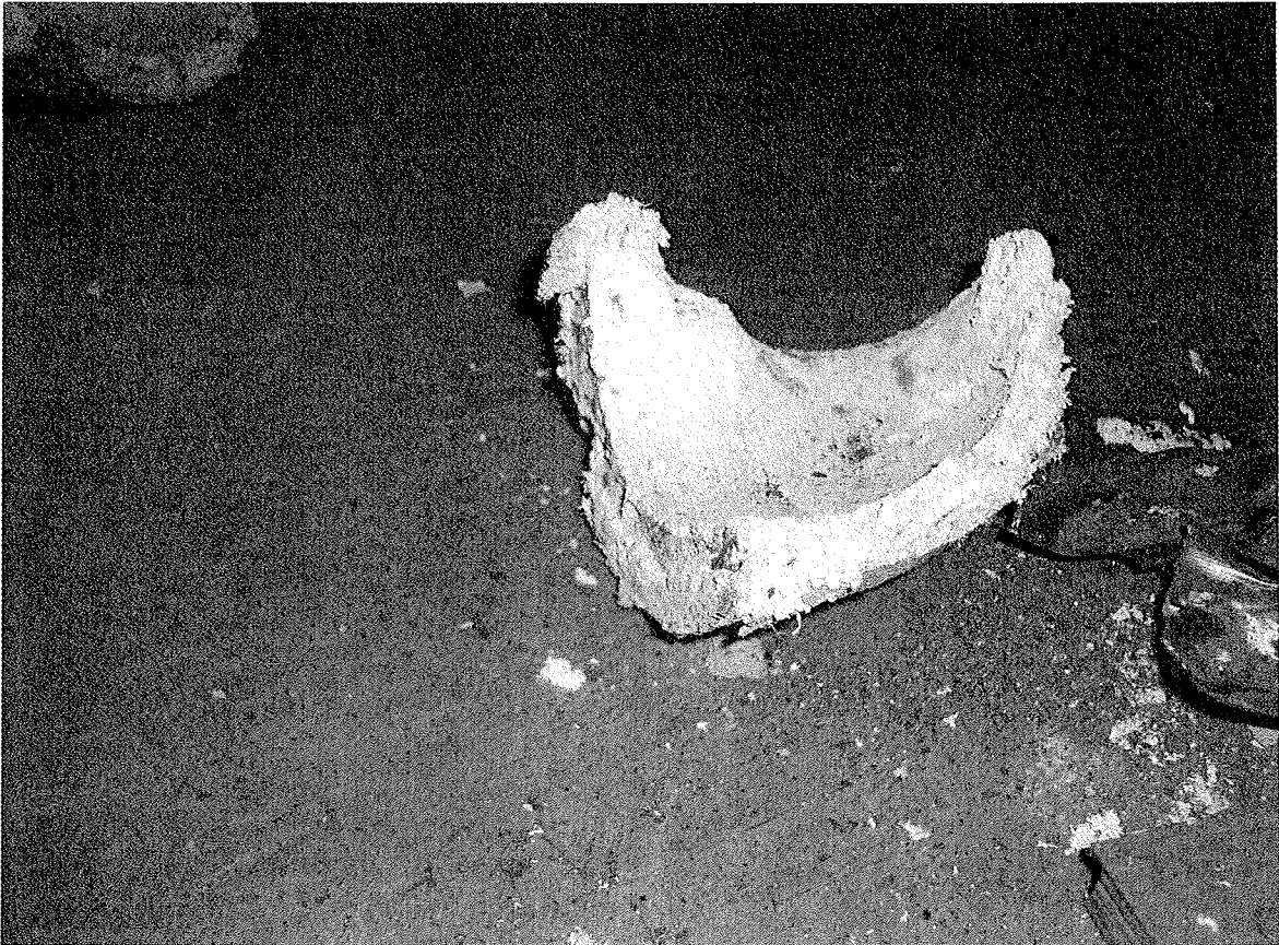
Crawlspace – asbestos pipe insulation contaminating the space
