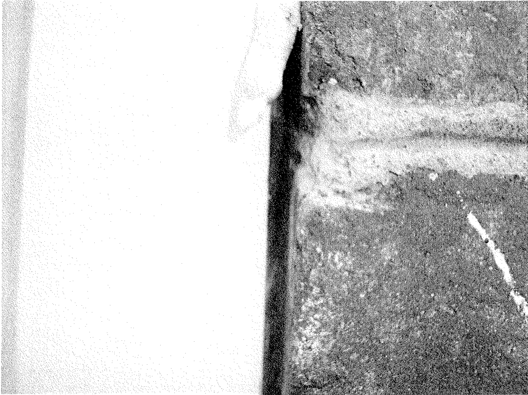
Old window caulking underneath new caulking
