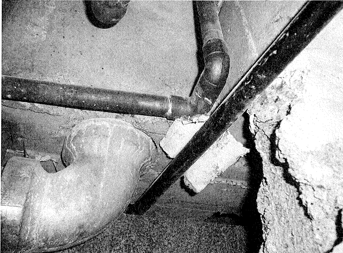
Room 123 – Piece of asbestos pipe insulation missed during abatement
