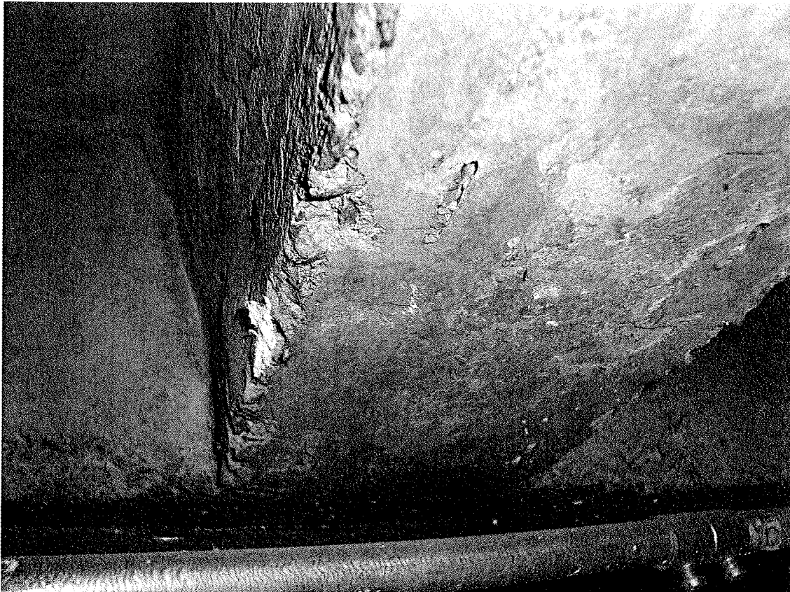
Room 122 – Pipe insulation residue/debris on concrete ceiling and electrical lines
