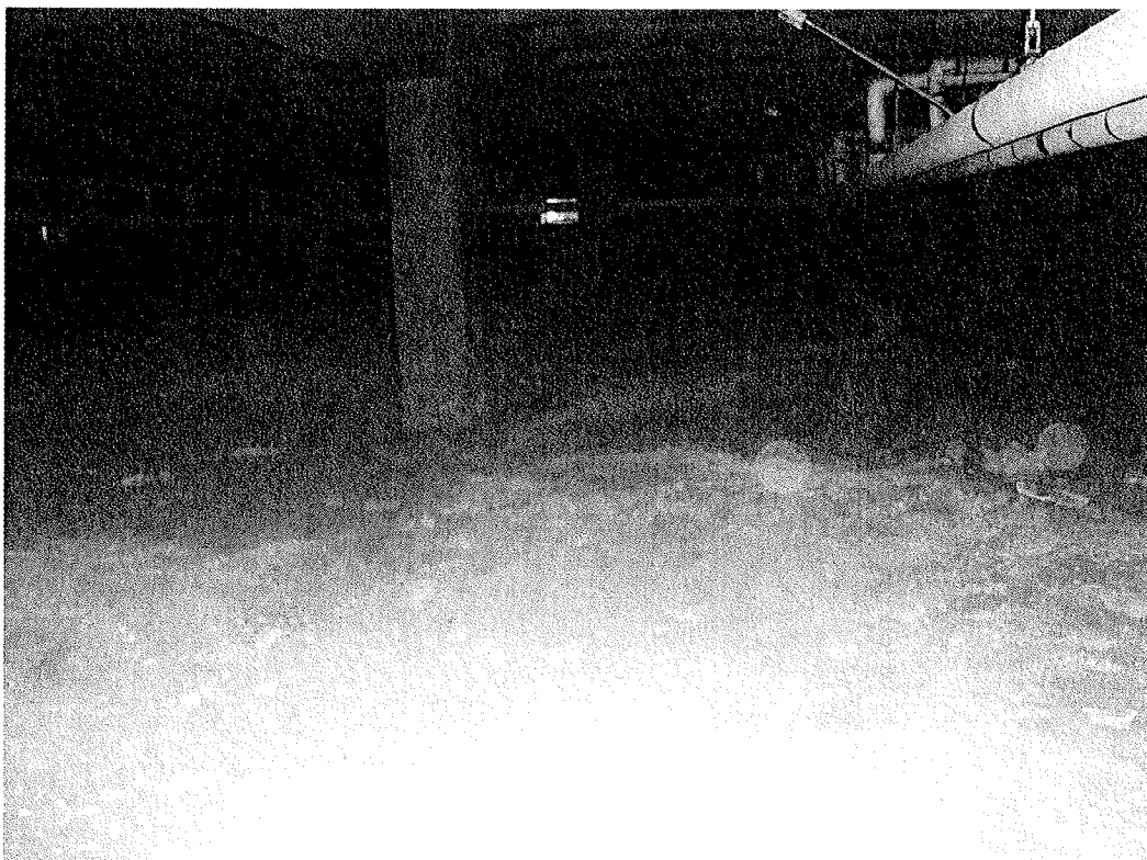
Crawlspace view with Asbestos pipe insulation and contaminated dirt floor
