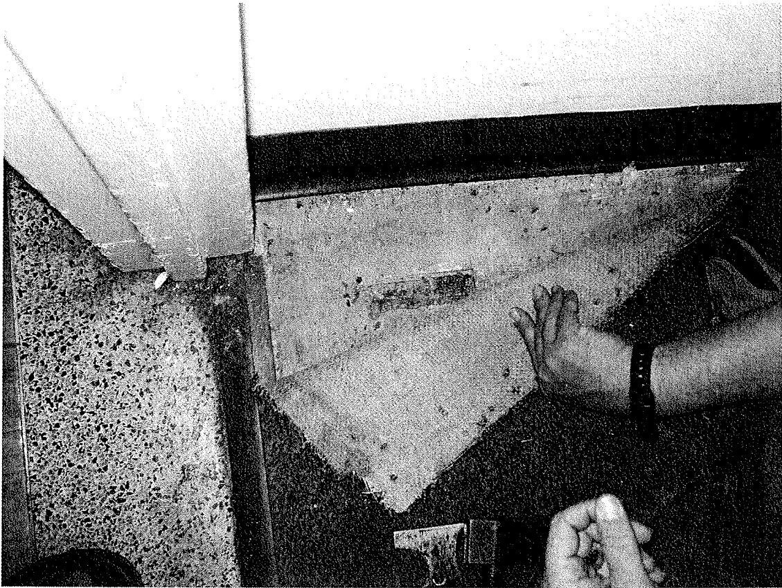
9x9 Red Floor Tile and Mastic under Carpet
