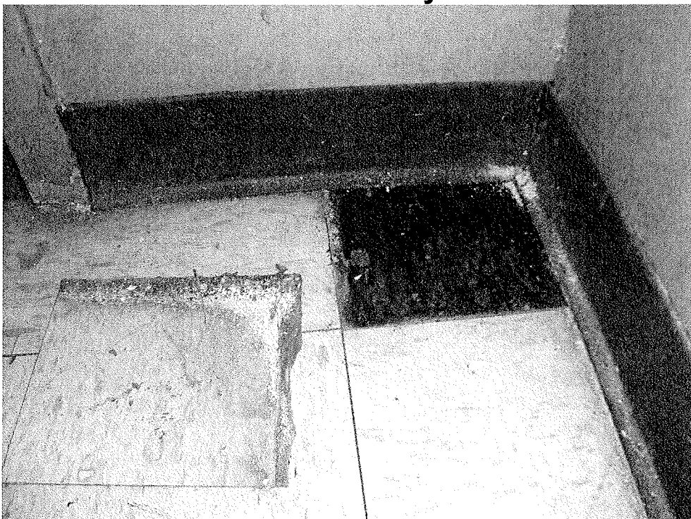
12"x12" Cream w/ Tan mottle floor tile and mastic – Chrysotile 2% and 4% respectively
