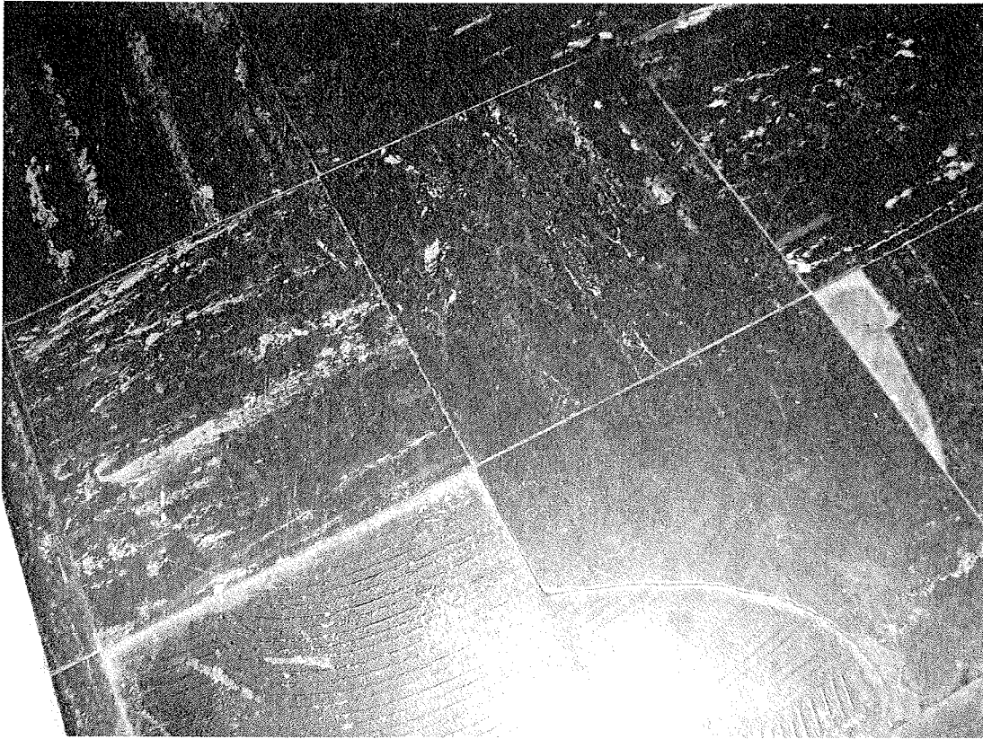
Brownish Red 9"x9" Floor Tile and Mastic – 15% and 5% Chrysotile (respectively)
