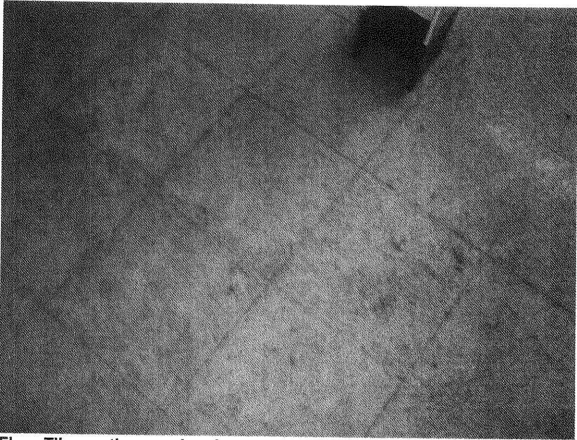
Floor Tile mastic associated with 12"x12" white floor tiles – 8% Chrysotile
