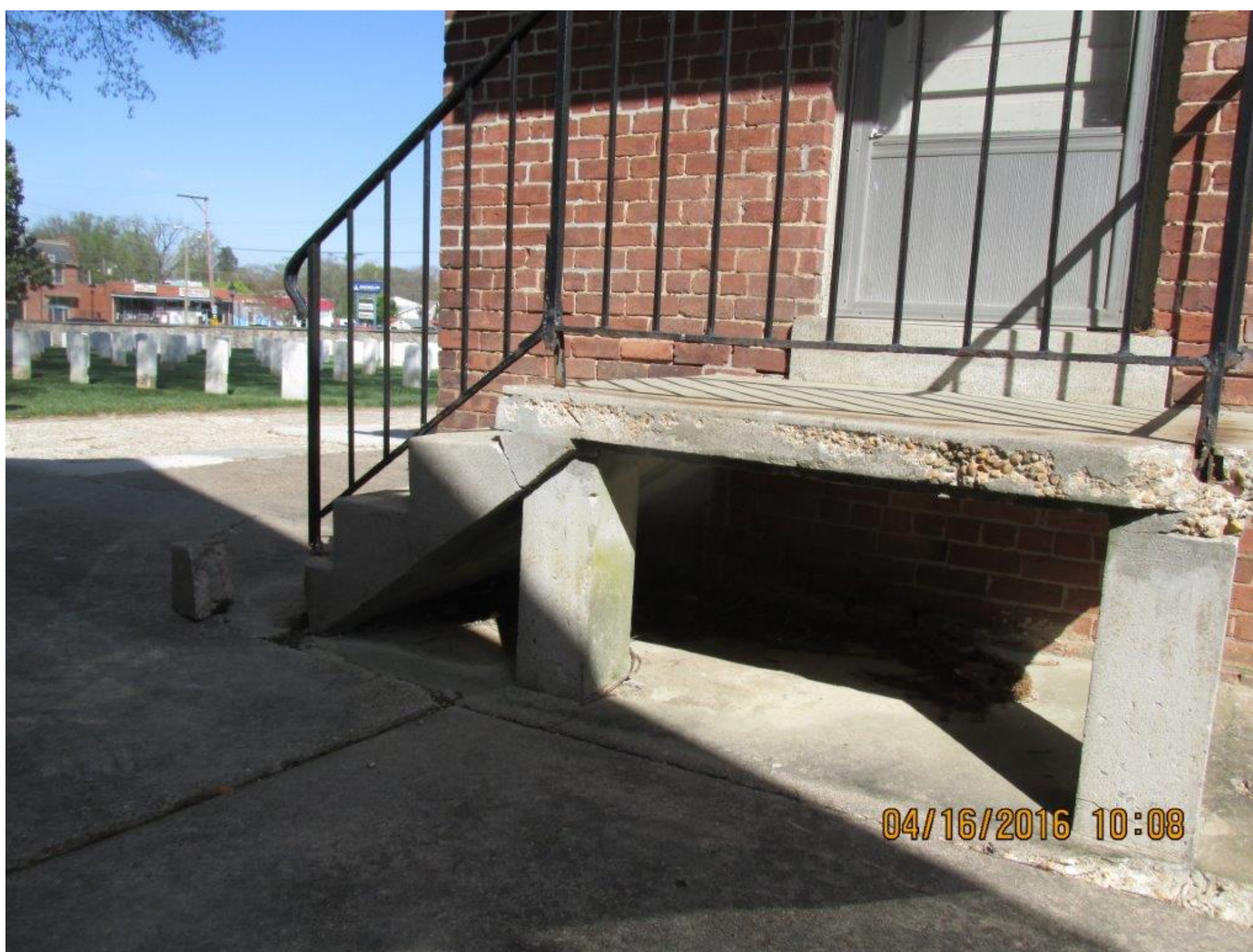
Detail 4: Demolish stairs, landing, and metal railing. Reuse existing columns. Design build a structural detail which matches existing dimensions of the stair, landing, and railings which are to be installed new. Tie structure into existing building and slab using epoxied rebar, or other design build solution. See specifications.
