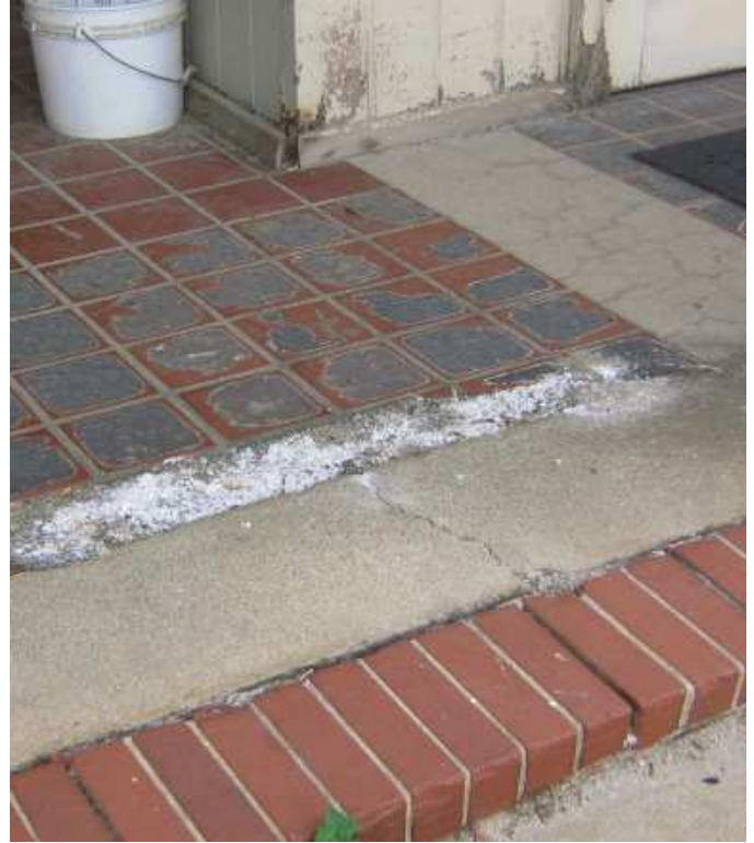
Photo 6: Cracking & Deterioration of Existing Concrete/Brick Patio Floor Slab.
