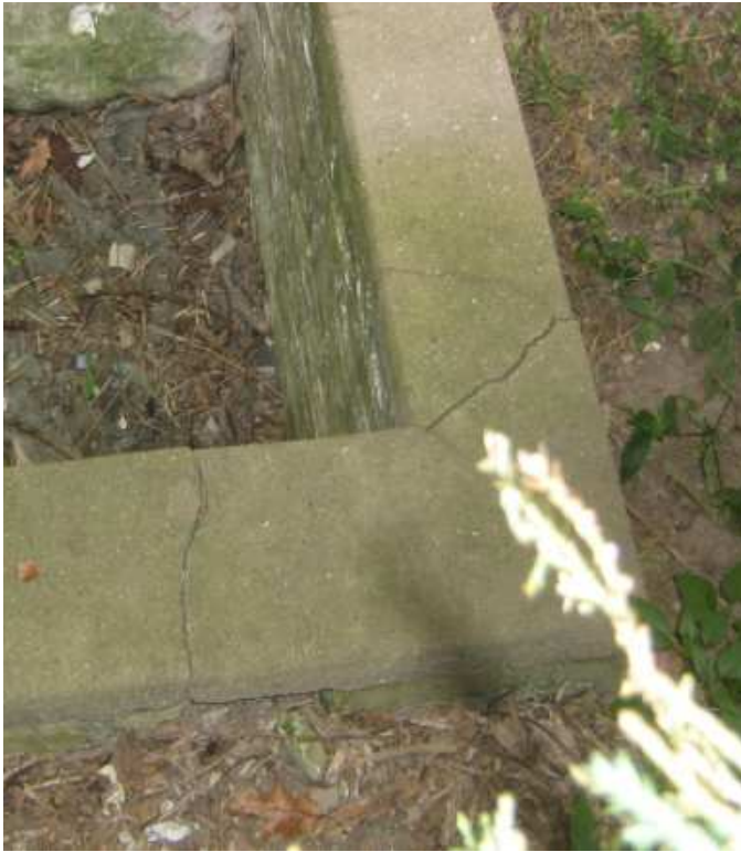
Photo 1: Deterioration & Cracking at Existing Area Well Walls.
