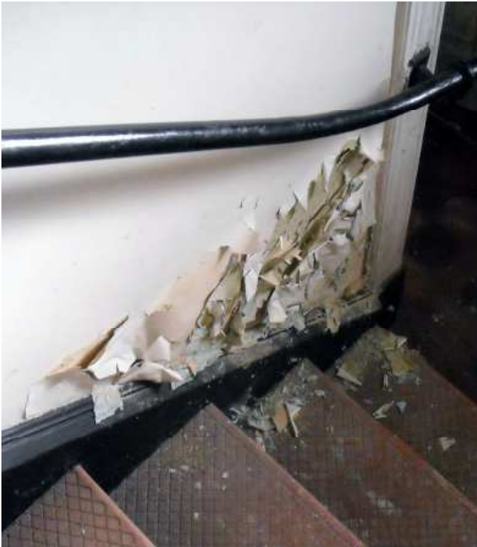
17 Paint peeling plaster wall from moisture damage.
