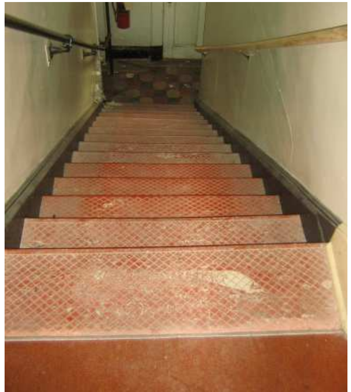
Photo 12: Warping of Existing Wood Stair.
