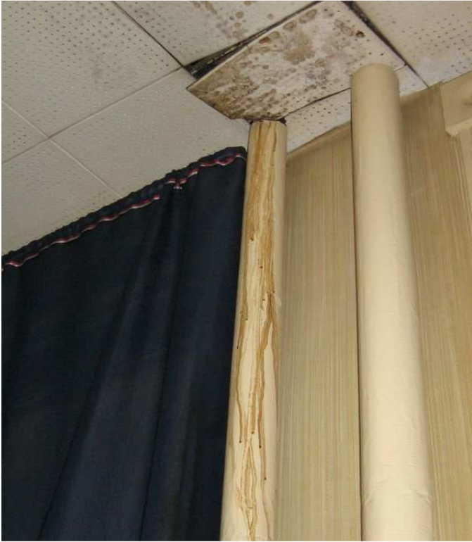
1 Water damaged ceiling tile.
