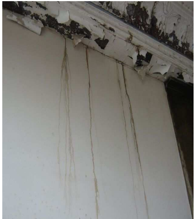
12 Water-stained material and peeling paint.
