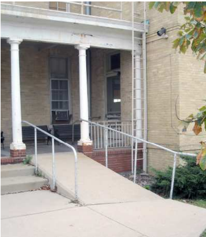
11 Non-compliant handicap ramp and railing.
