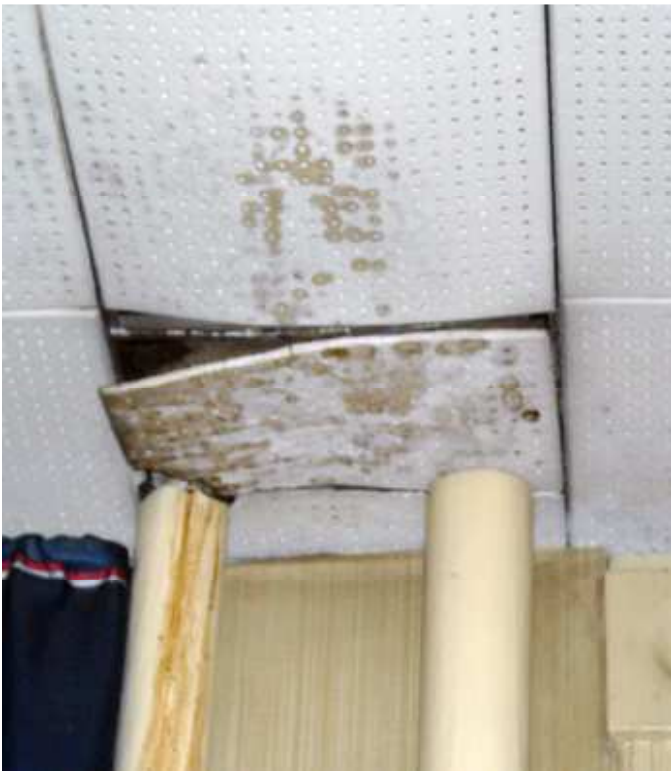
15 Water damaged acoustical ceiling tile.
