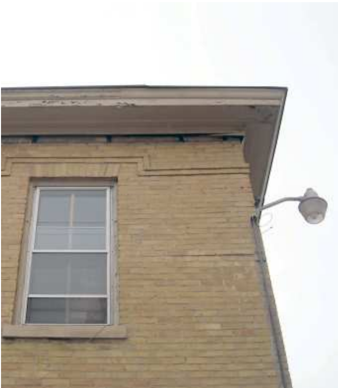
7 Deteriorating wood soffit, trim & inappropriate light fixture.
