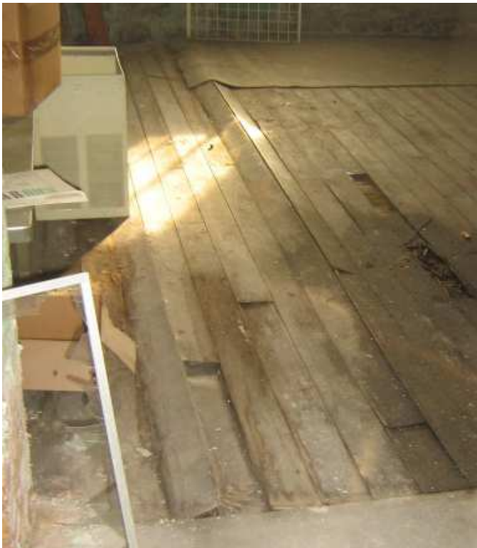
Photo 11: Heaving of Existing Basement Floor Boards.
