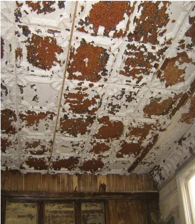
9 Peeling paint on ceiling.
