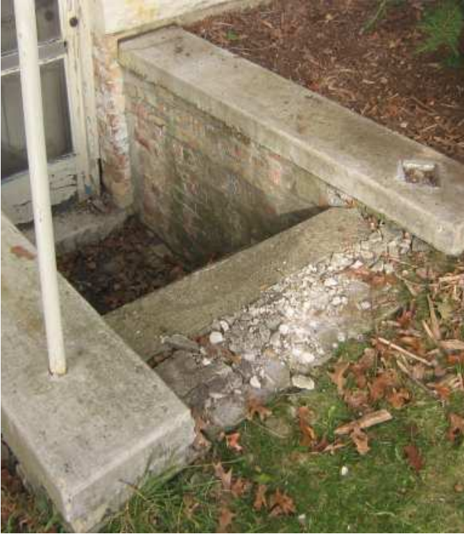
Photo 5: Cracking & Deterioration of Existing Concrete Stair.
