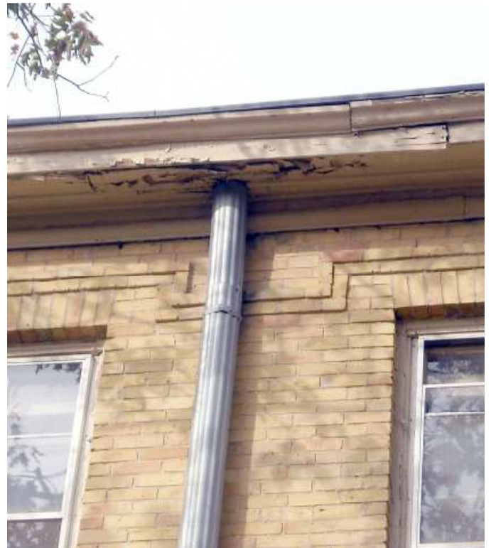
8 Peeling paint at fascia and soffits.
