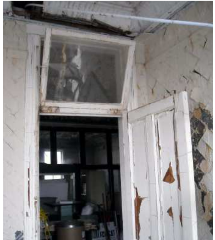
22 Paint peeling from door assembly and tin wall covering.
