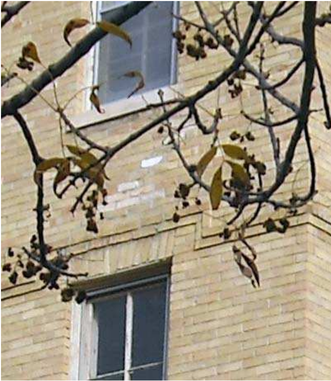
5 Brick repair does not match existing adjacent brick.
