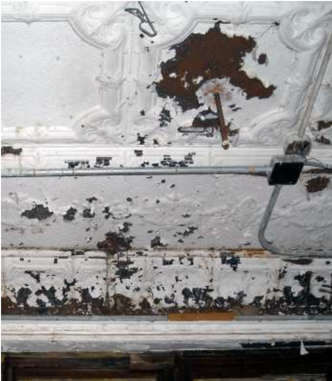
13 Paint peeling from tin ceiling.
