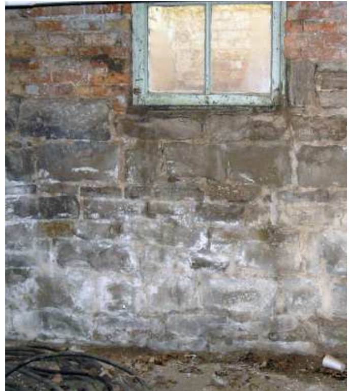
26 Dirt, pollutants and efflorescence on brick and stone wall.
