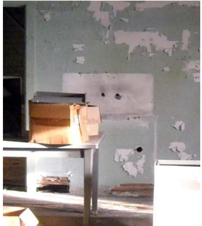
18 Damaged wall from old plumbing fixtures.
