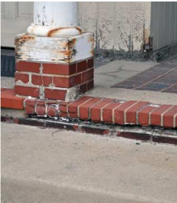
3 Deteriorating brick pavers.
