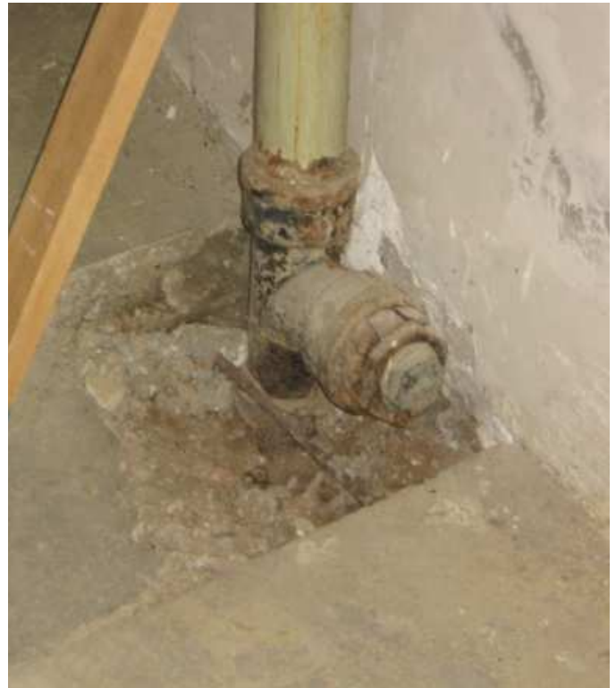
Photo 8: Missing Concrete Floor Slab.
