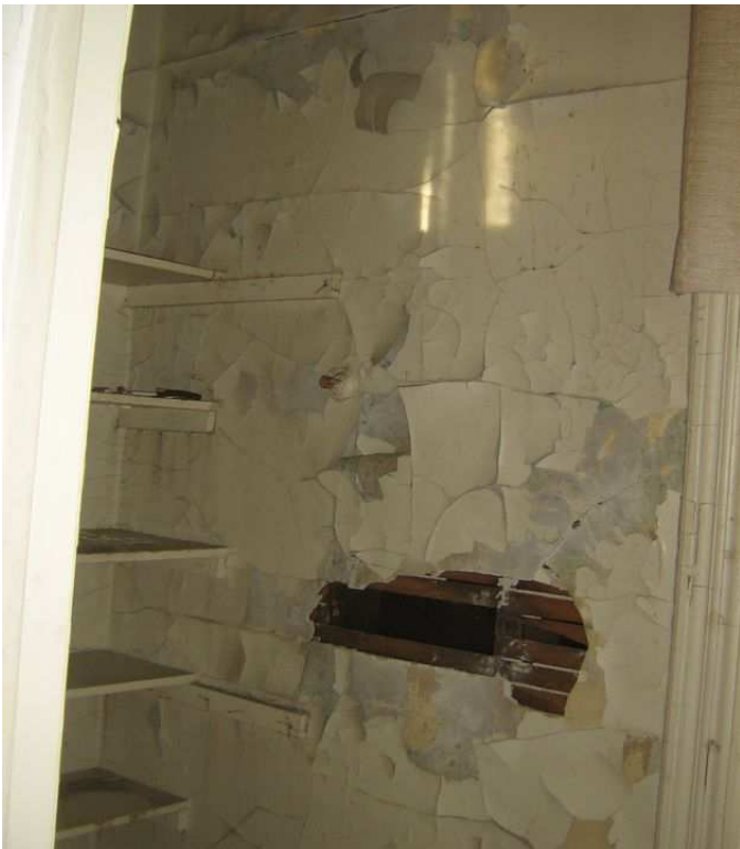
3 Damaged plaster.
