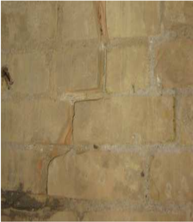
Photo 9: Cracking & Deterioration of Existing Masonry Foundation Walls.
