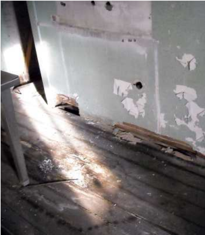
25 Dirt, pollutants and stained wood flooring.
