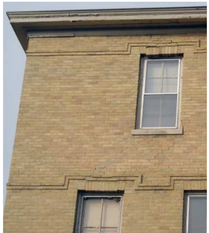
4 Cracked and loose bricks.
