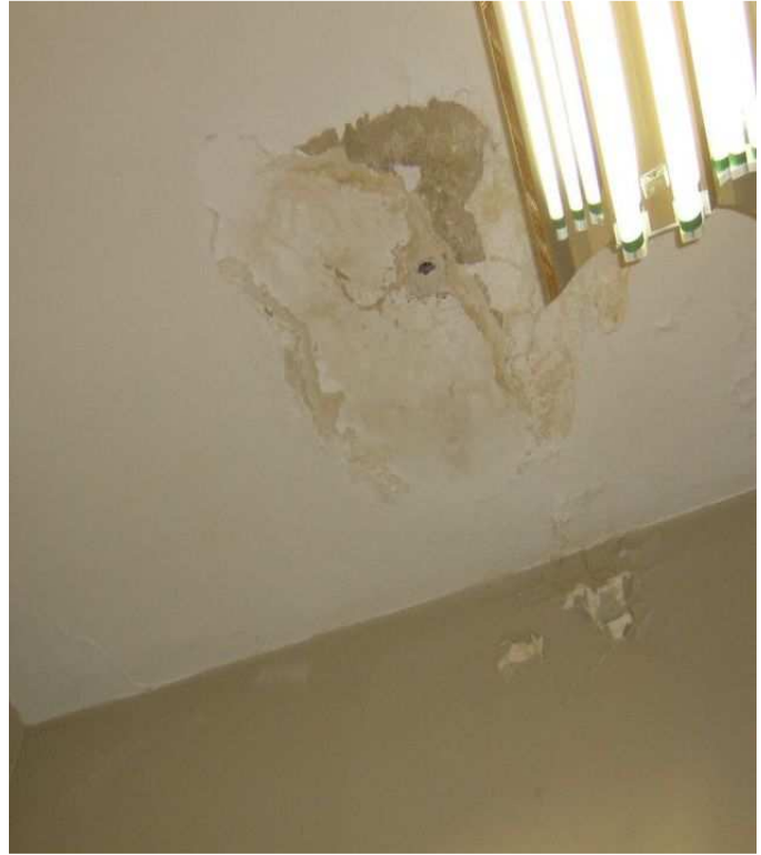
2 Damaged plaster ceiling and wall.
