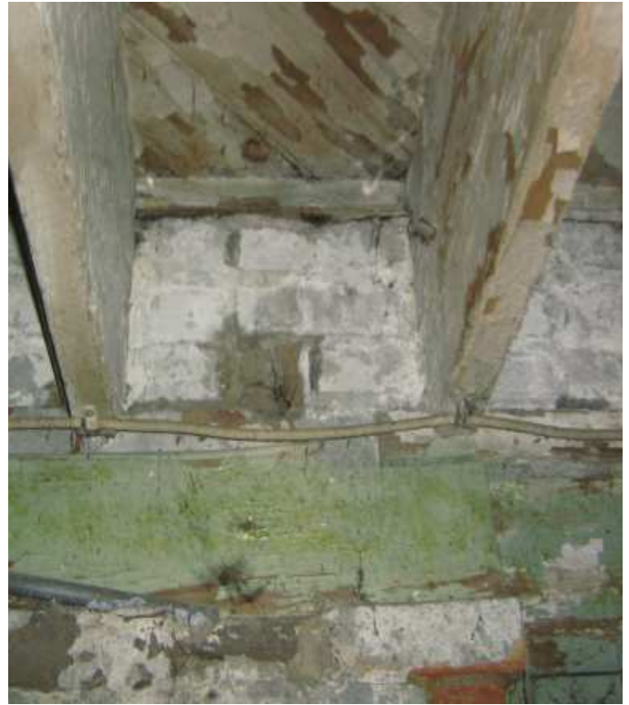
Photo 10: Deterioration of Existing Wood Floor Framing.
