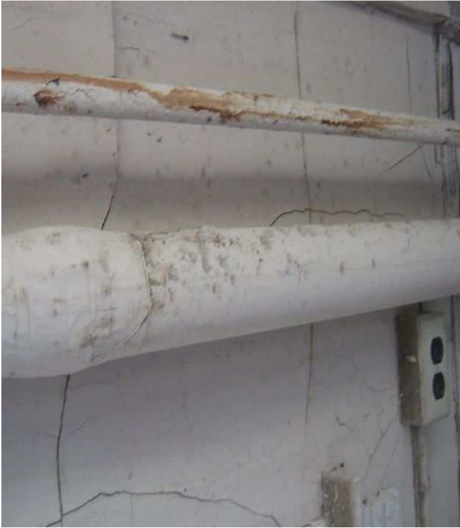
5 Damaged thermal insulation and suspect mold growth.
