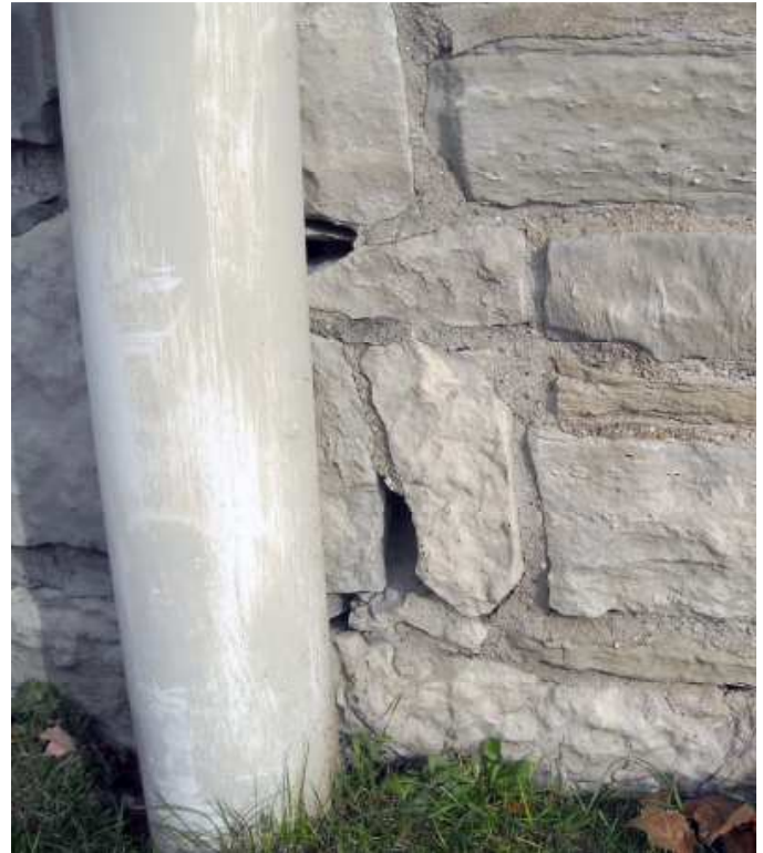
10 Stone mortar washed away at downspout area.
