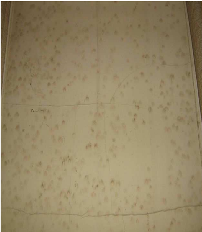
11 Suspect mold growth on wall.
