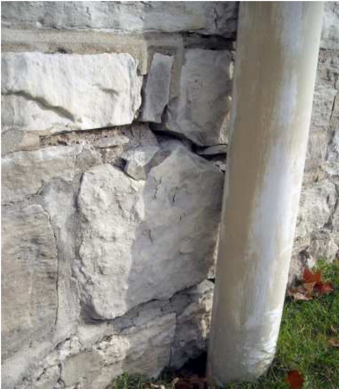
1 Missing mortar at stone foundation wall.
