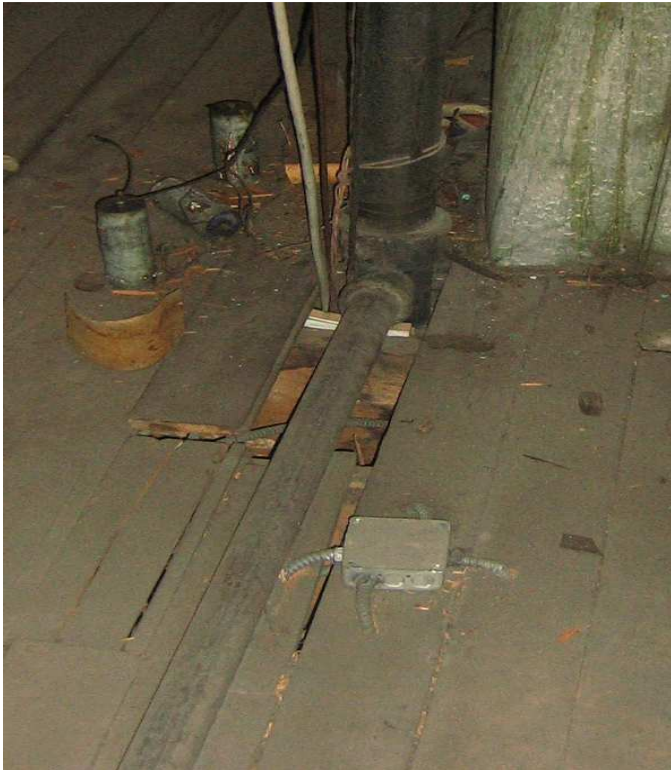
Photo 13: Damaged & Missing Roof Floor boards.
