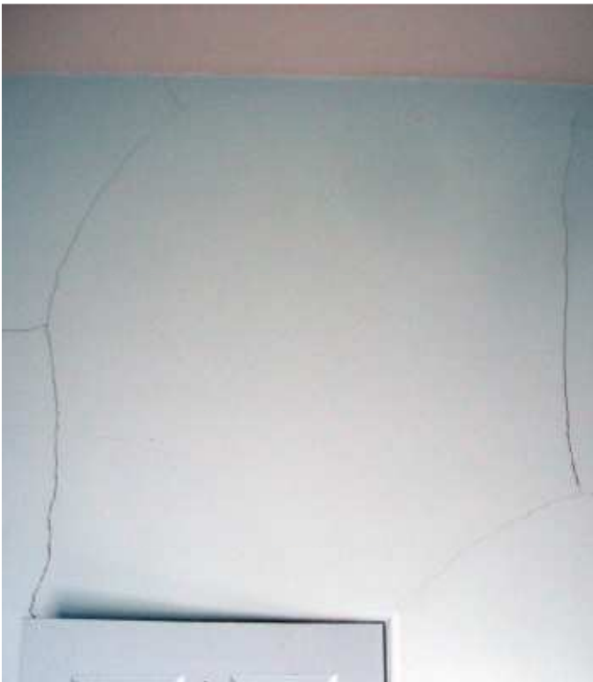
19 Cracked and damaged plaster walls.
