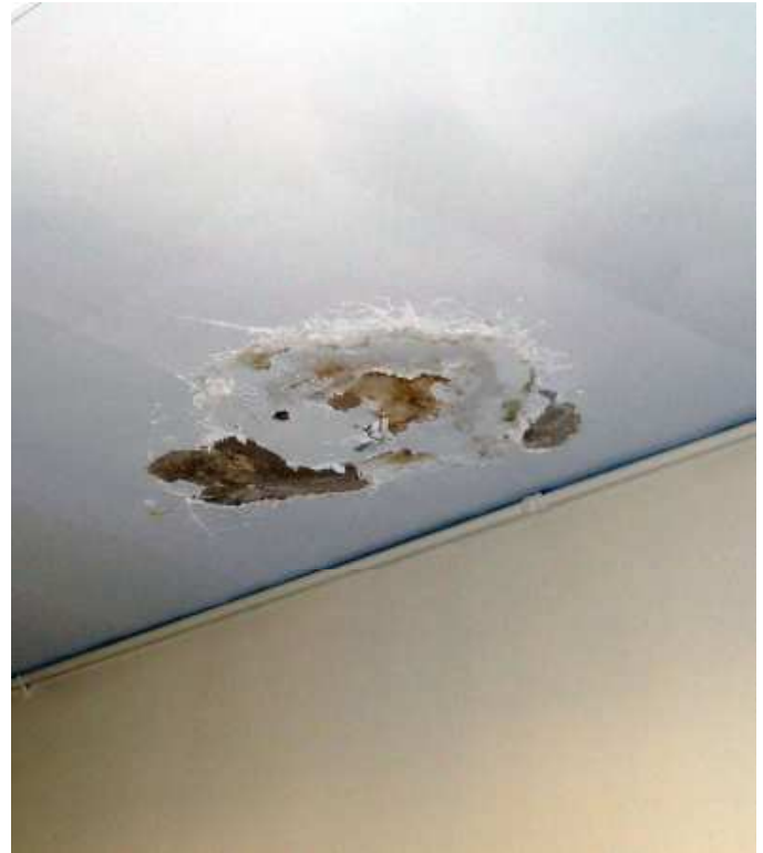
14 Water damage with paint peeling at plaster ceiling.
