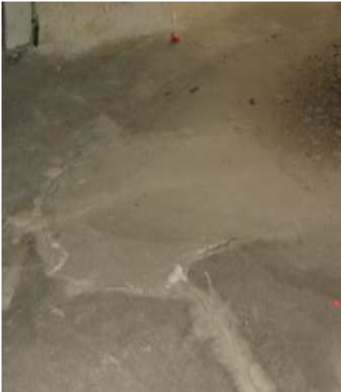
Photo 7: Cracking & Deterioration of Existing Concrete Floor Slab.
