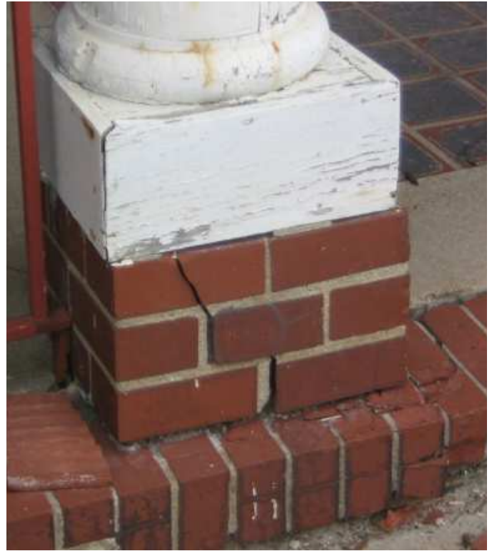
Photo 2: Deterioration & Cracking at Existing Column Base.
