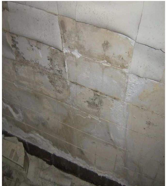
4 Damaged brick mortar and suspect mold growth on wall.
