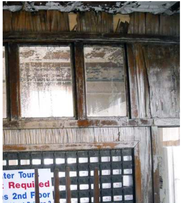
20 Deteriorating wood partition wall with extensive water damage.
