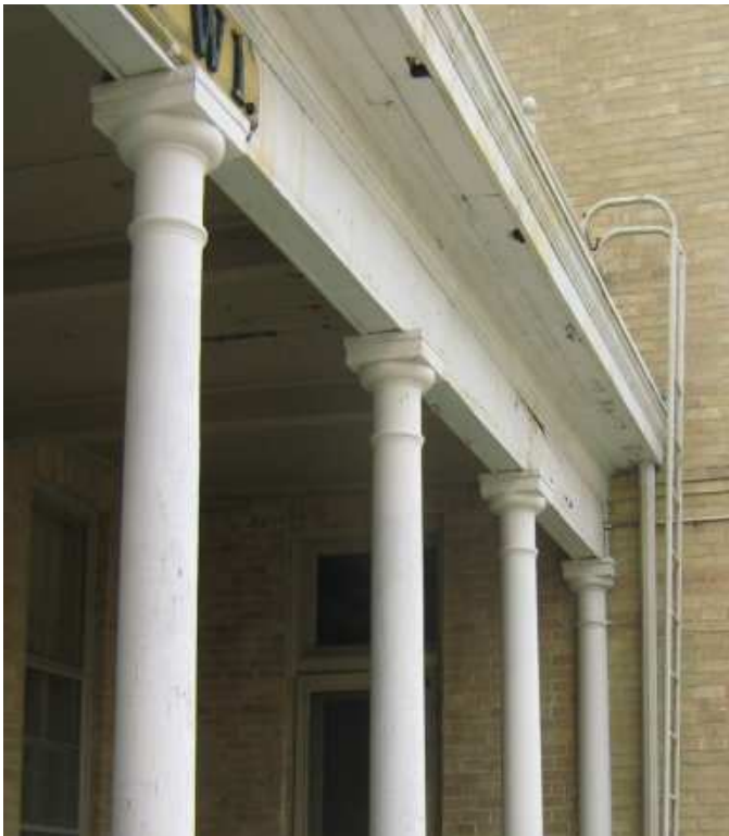
Photo 3: Deterioration of Existing Wood Porch Framing.
