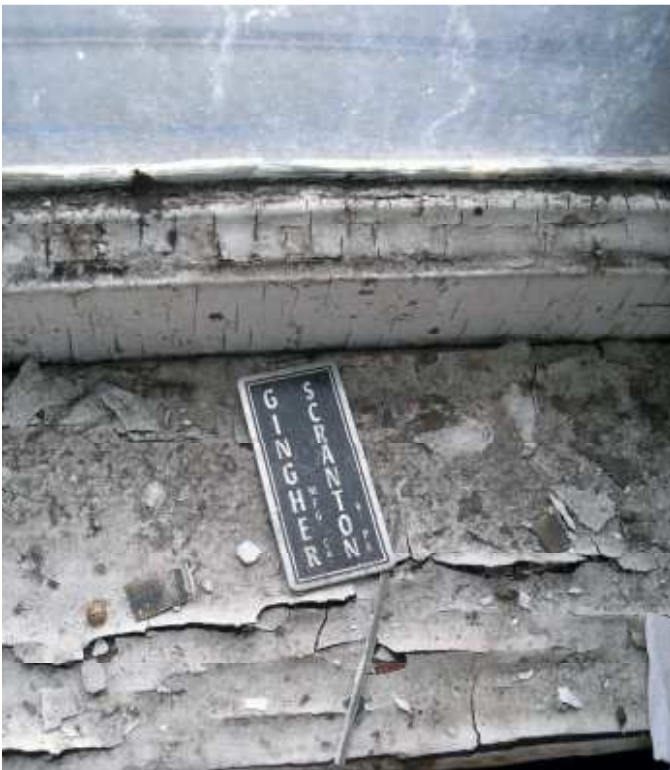
23 Dirt, pollutants and paint peeling from window assembly.
