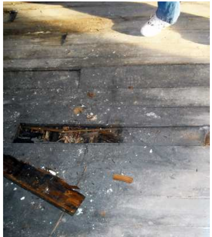
24 Loose and missing floor boards.
