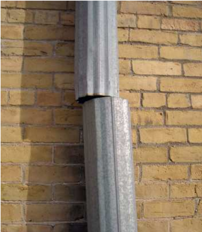
9 Leak at downspout.
