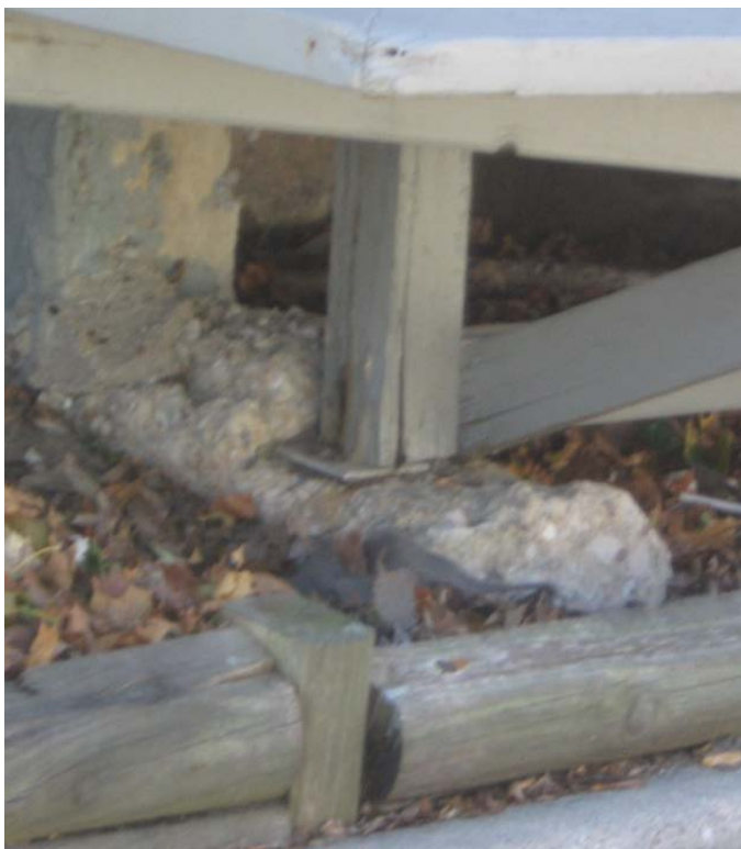
Photo 3: Deterioration & Cracking at Patio Stair Concrete Foundation Walls.
