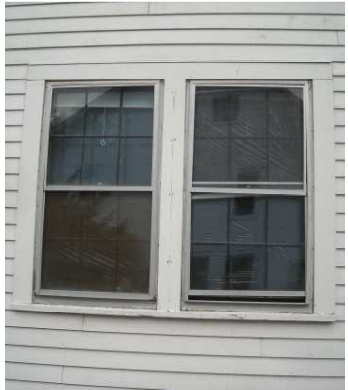
6 Inappropriate aluminum storm windows; deteriorating caulk.
