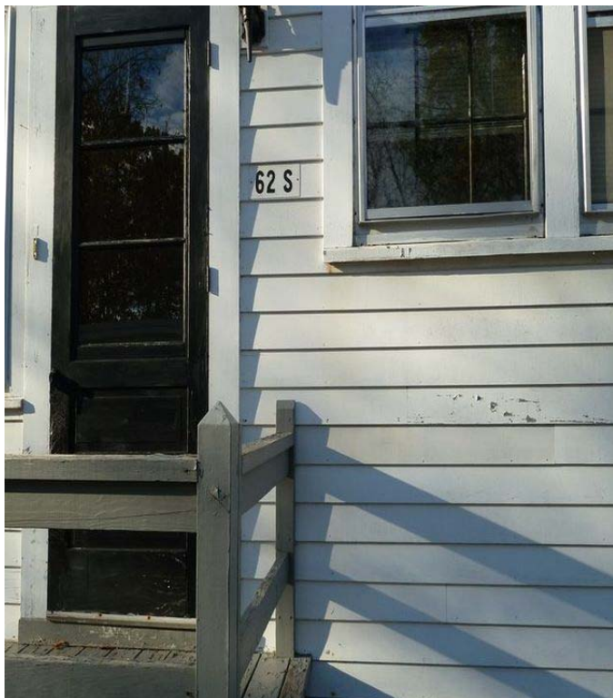
1 Peeling paint on wood clapboards, window frame, and stairs.
