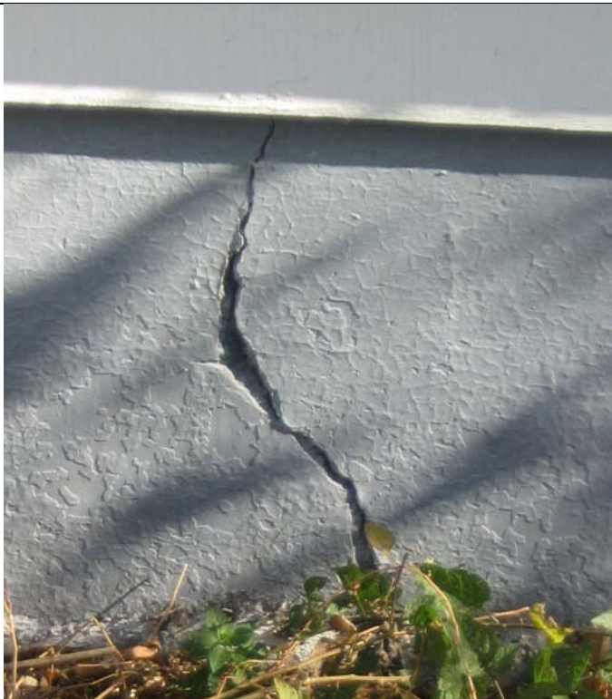
Photo 1: Deterioration & Cracking at Existing Concrete Foundation Walls.
