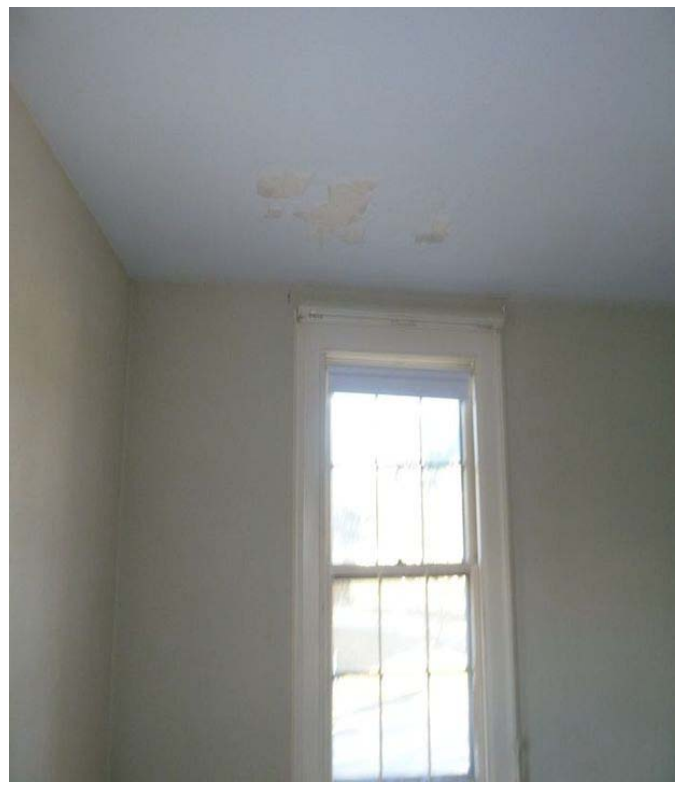
4 Peeling paint on ceiling.
