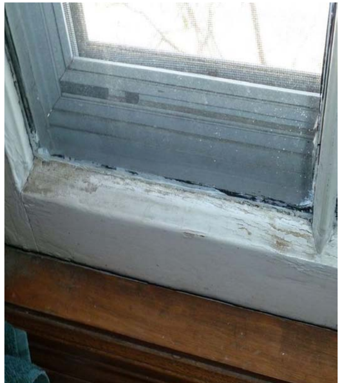
8 Suspect mold growth on window frame.
