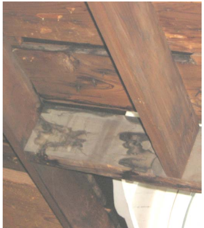
Photo 12: Deterioration of Existing Wood Roof Framing & Associated Roof Boards.
