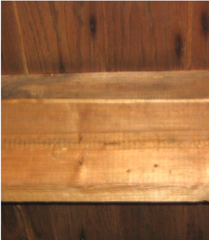
Photo 9: Deterioration & Splitting of Existing Wood Roof Truss.
