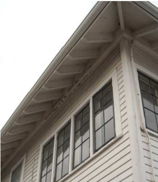
7 Peeling paint at soffits and fascia.
