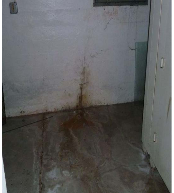
6 Discoloration on basement wall and floor.
