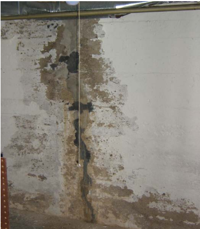
Photo 7: Deterioration & Cracking at Existing Concrete Foundation Walls.
