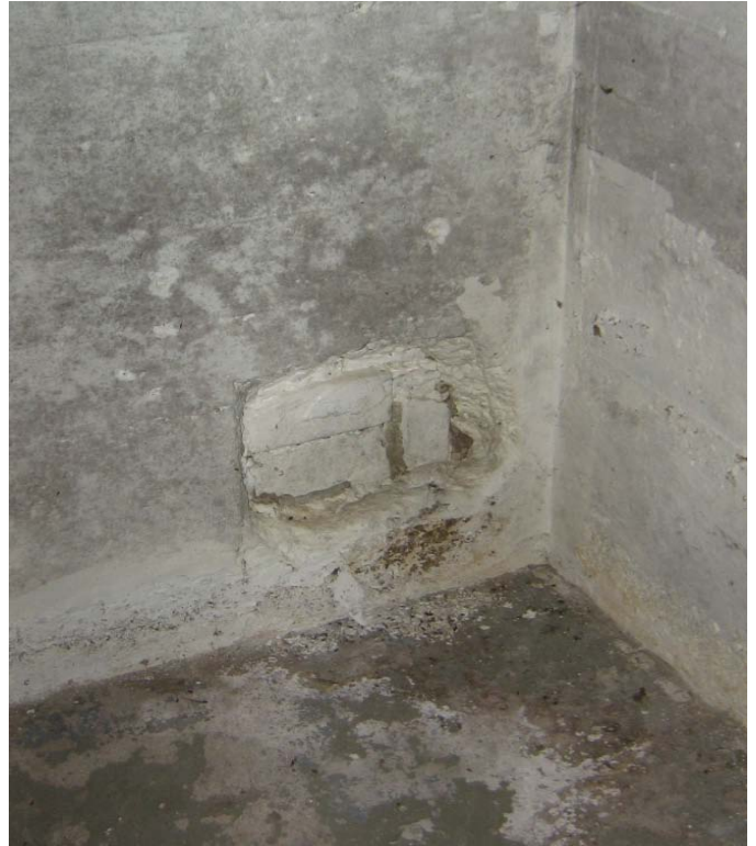
Photo 8: Deterioration & Cracking at Existing Concrete Foundation Walls.
