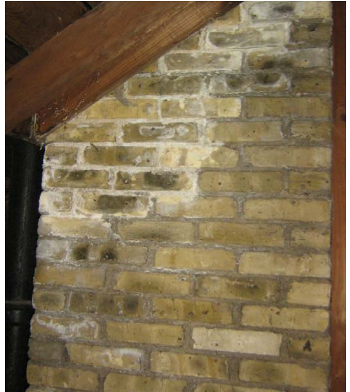
Photo 10: Deterioration of Existing Brick Chimney Stack.
