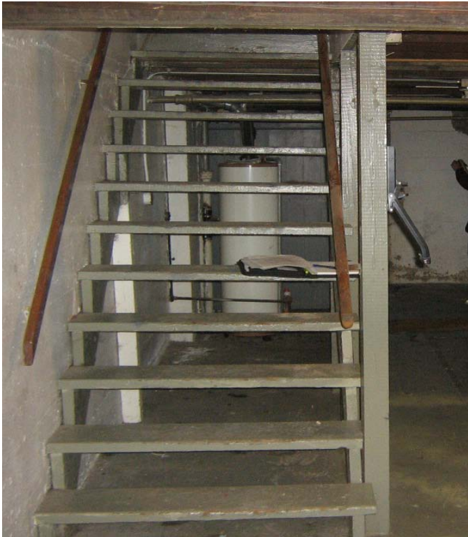
Photo 13: Deterioration & Warping of Existing Interior Wood Stair.
