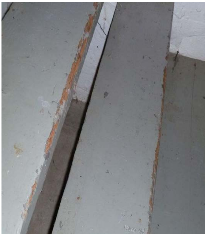
3 Peeling paint on basement stairs.
