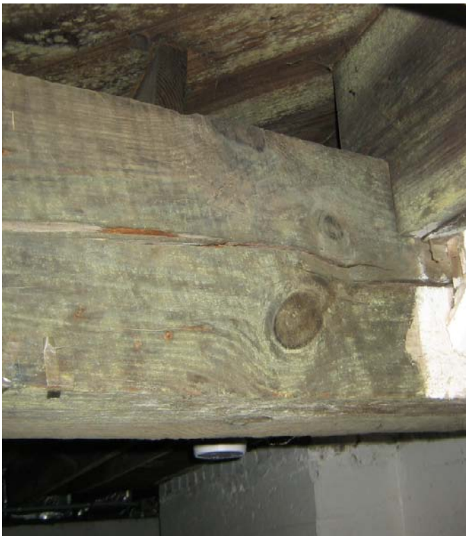
Photo 11: Deterioration of Existing Wood Floor Beam & Associated Floor Framing.
