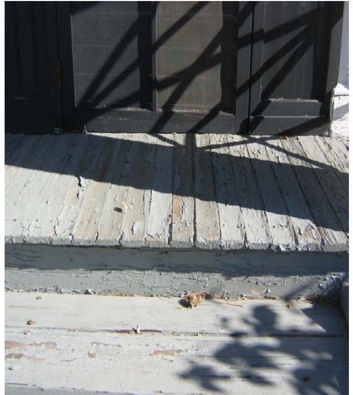
Photo 6: Deterioration of Exterior Wood Patio & Associated Wood Floor Boards.
