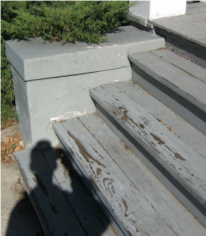
Photo 5: Deterioration of Exterior Wood Stair & Associated Framing.
