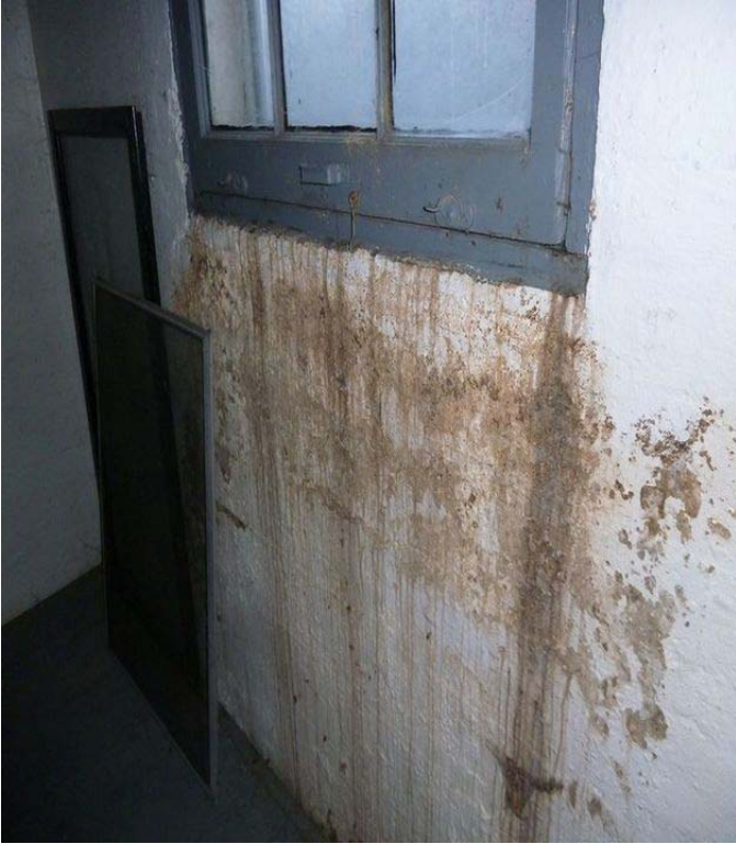
5 Discoloration on basement wall.
