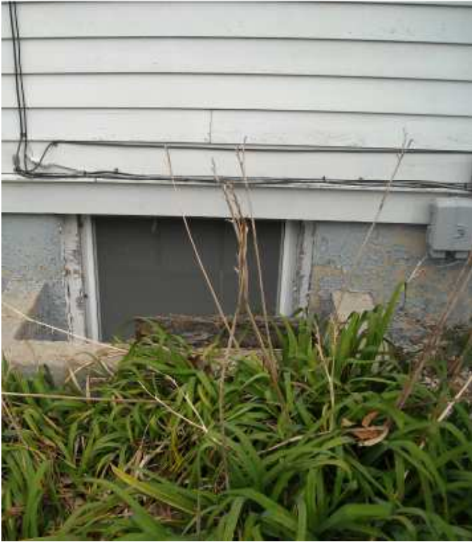
1 Peeling paint at concrete foundation and wood windows.
