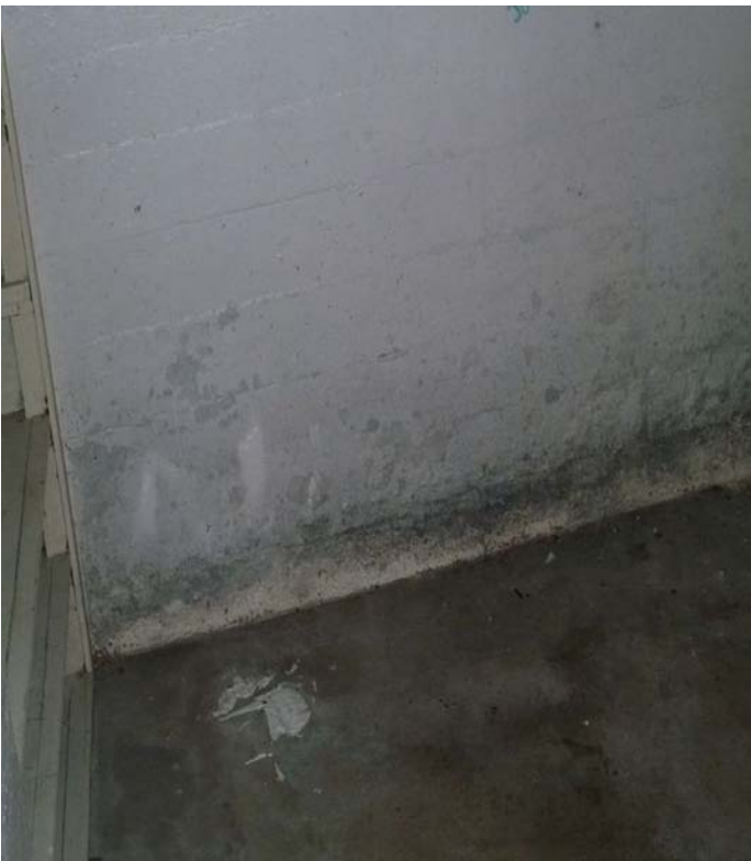
7 Suspect mold growth on basement wall.
