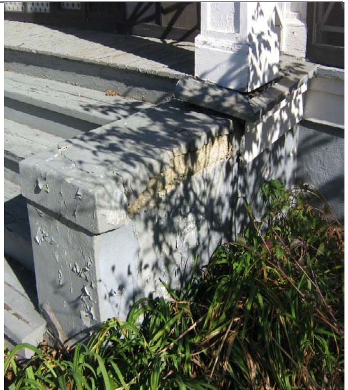
Photo 2: Deterioration & Cracking at Existing Concrete Foundation Walls.
