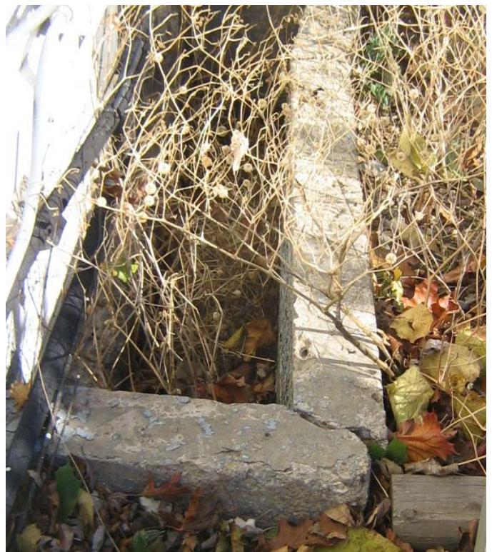
Photo 4: Deterioration & Cracking at Existing Area Well Concrete Foundation Walls.
