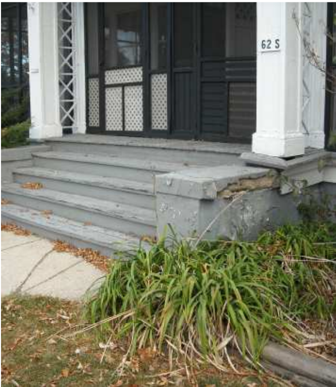
3 Damaged concrete trim; advanced structural deterioration at wood porch.
