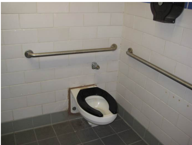
Figure 3: Water closet.
