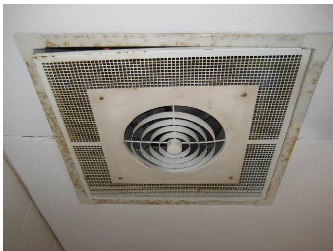
Figure 7: Electric heater register.
