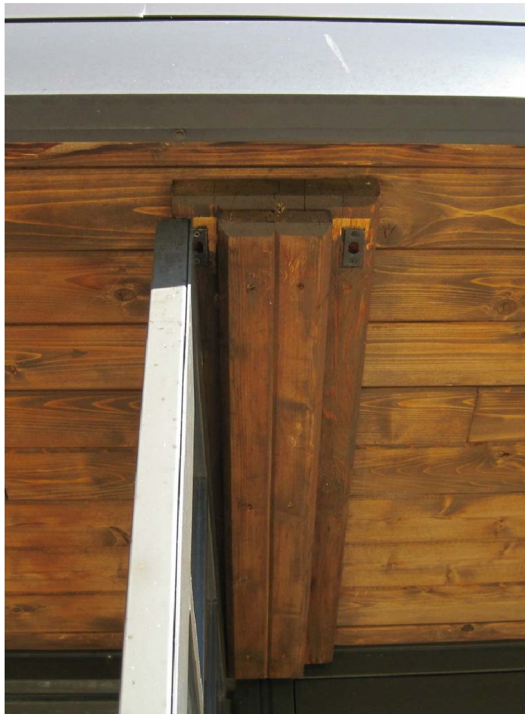
6E L-3 REFERENCE PHOTO EXISTING EAVE MOUNTED DOOR STOP
