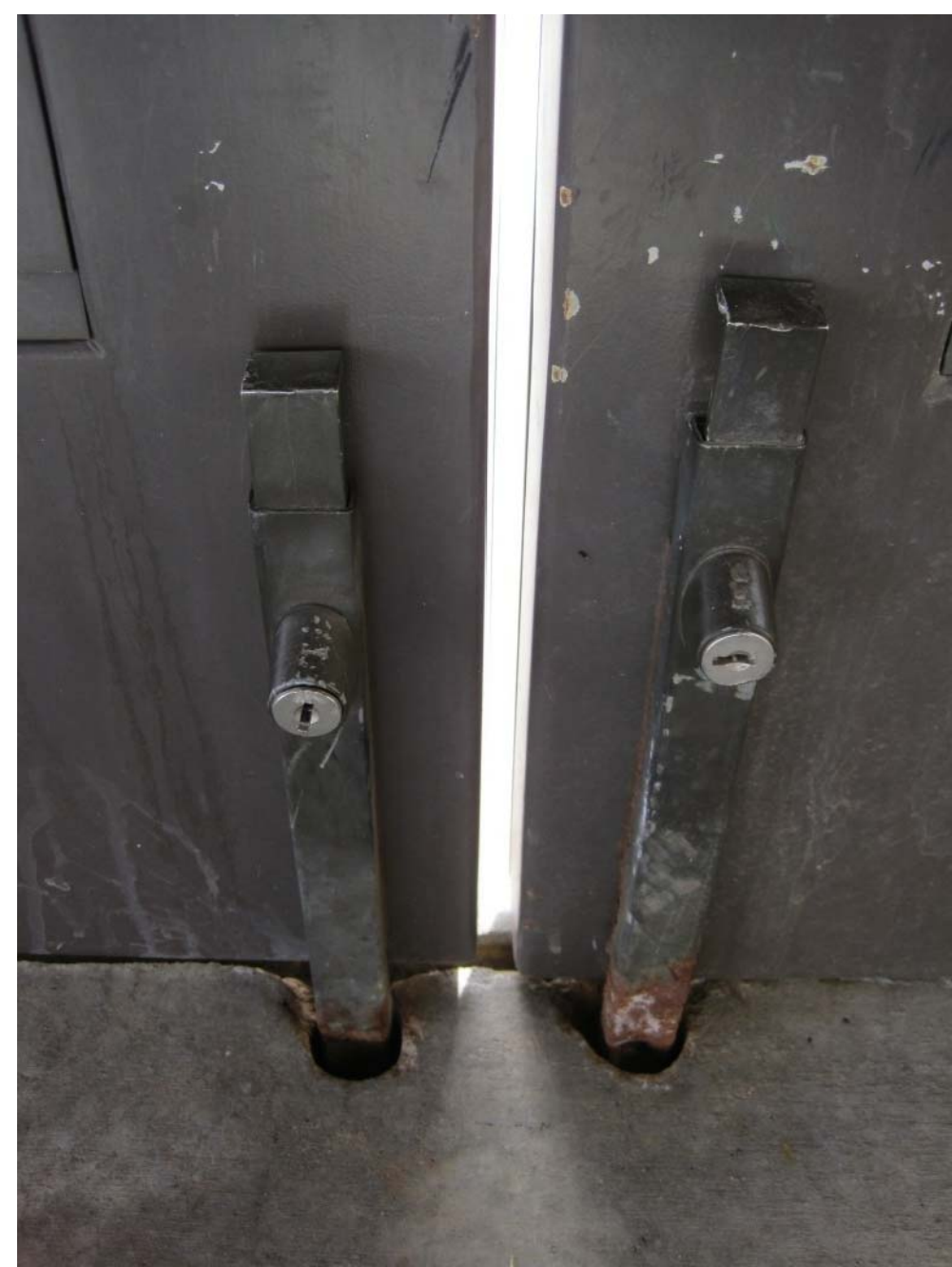
2G L-3 REFERENCE PHOTO EXISTING FLOOR SURFACE BOLT (DOOR IN OPEN POSITION)
