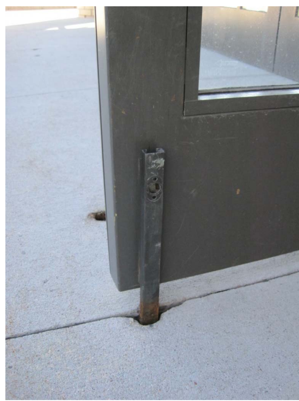
4G L-3 REFERENCE PHOTO EXISTING FLOOR SURFACE BOLT (DOOR IN OPEN POSITION)
