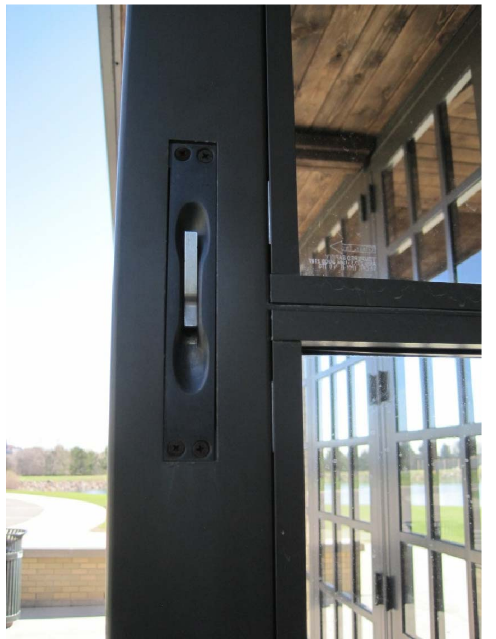
8E L-3 REFERENCE PHOTO EXISTING CONCEALED DOOR BOLT SYSTEM TO BE REMOVED AND OPENINGS COVERED
