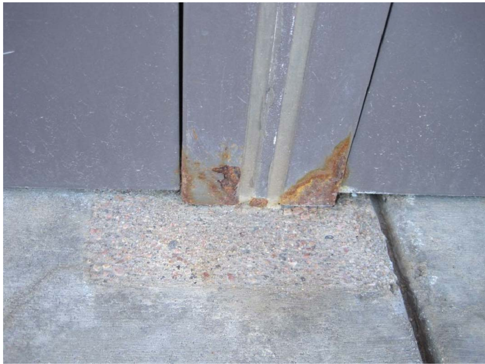
6C L-3 REFERENCE PHOTO EXISTING DOOR & DOOR FRAME CONDITIONS (RUST)
