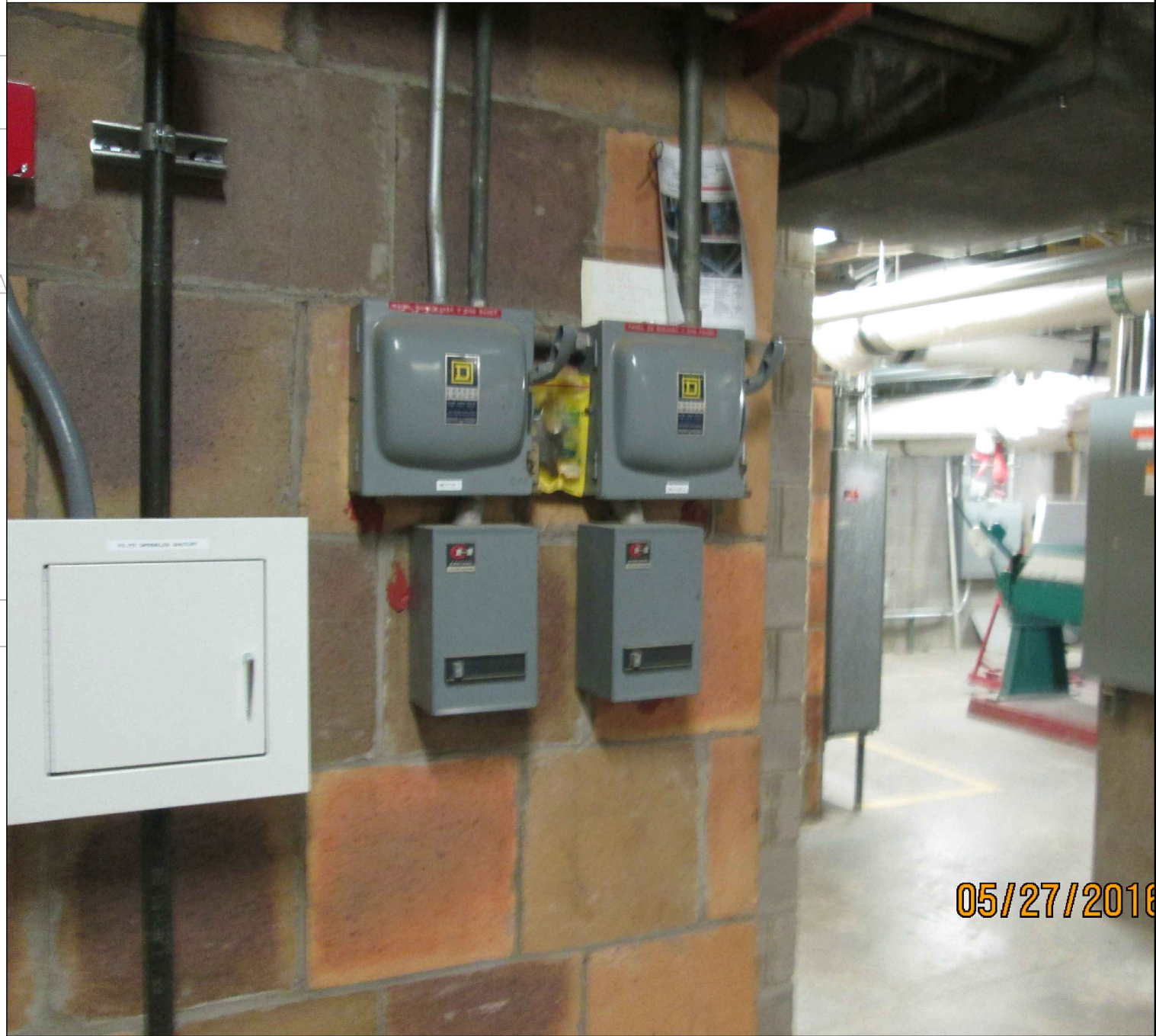
EXISTING PUMP DISCONNECT.
