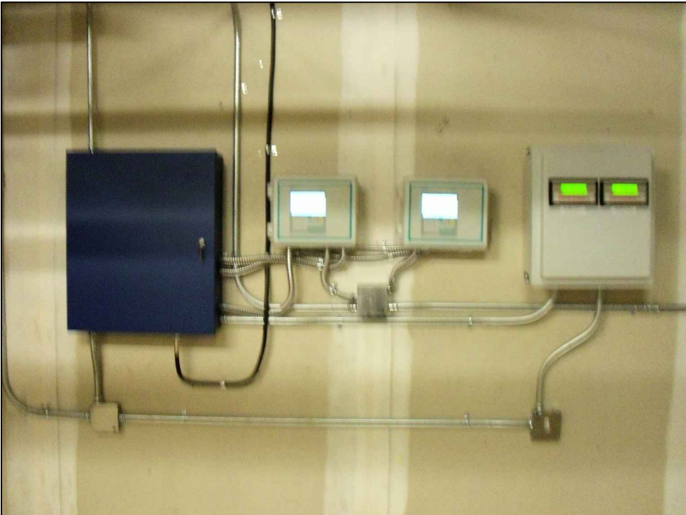
BLDG. 4 METER HEADS AND PANEL INSTALLED
