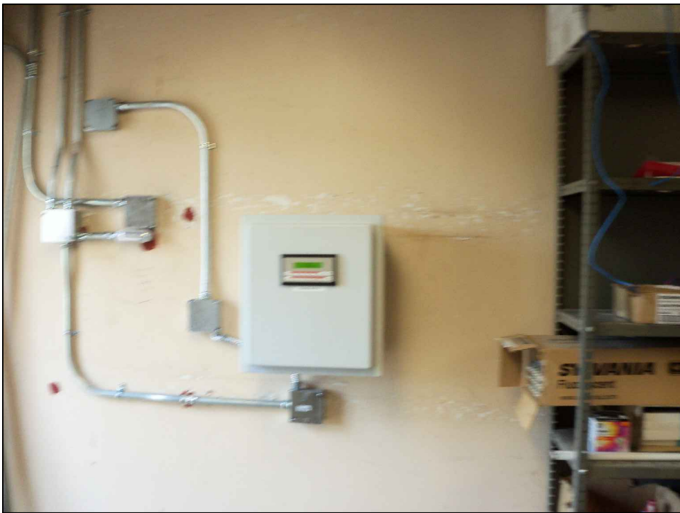
BLDG. 45 ST-1 METER HEAD INSTALLED
