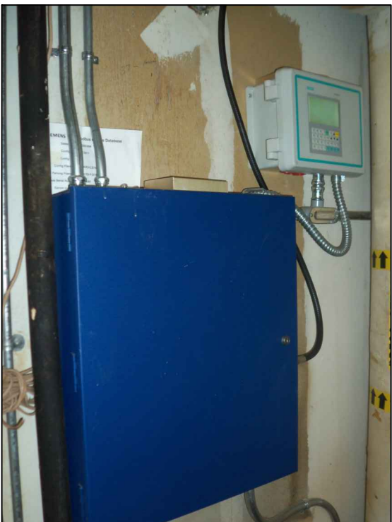
BLDG. 9 METER HEADS AND PANEL INSTALLED
