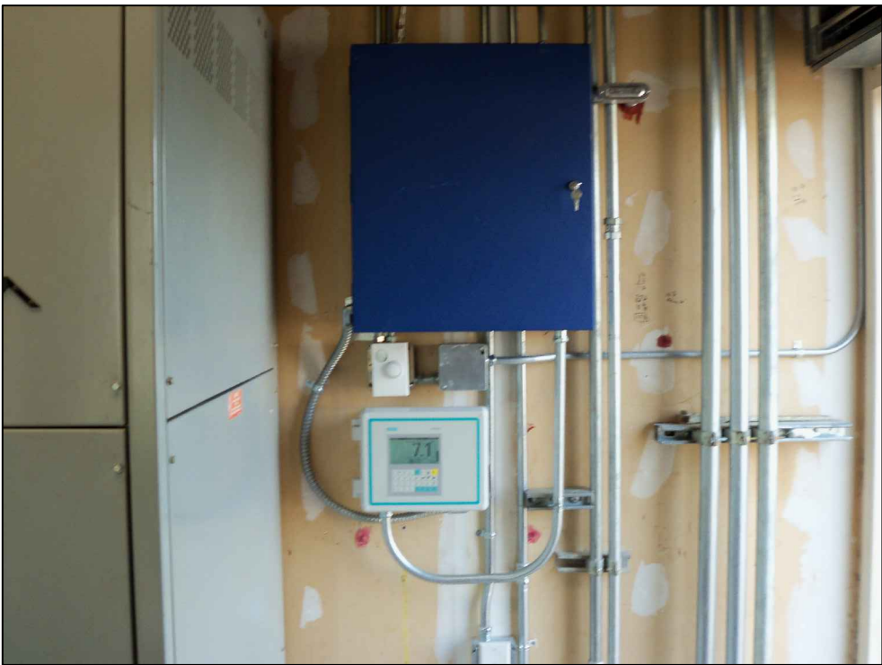
BLDG. 45 CHW-1 AND PW-1 METER HEADS AND PANEL INSTALLED
