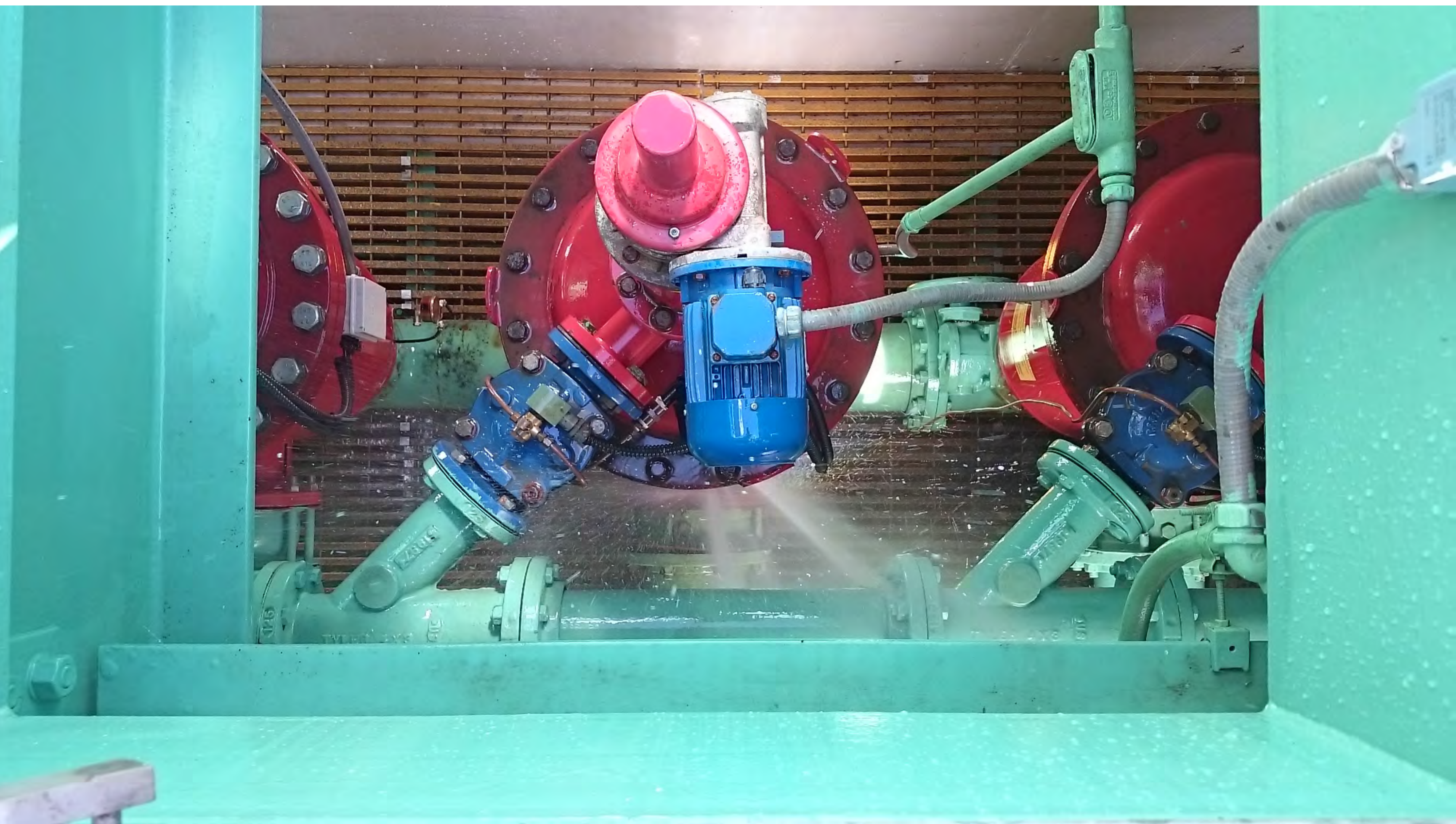
Details 1 and 2: Demolish and replace with new the filter in the above detail. Connect to existing valves and piping. The picture above and right shows the leaking filter (top view) to be replaced. Access is down a hatch and ladder.
