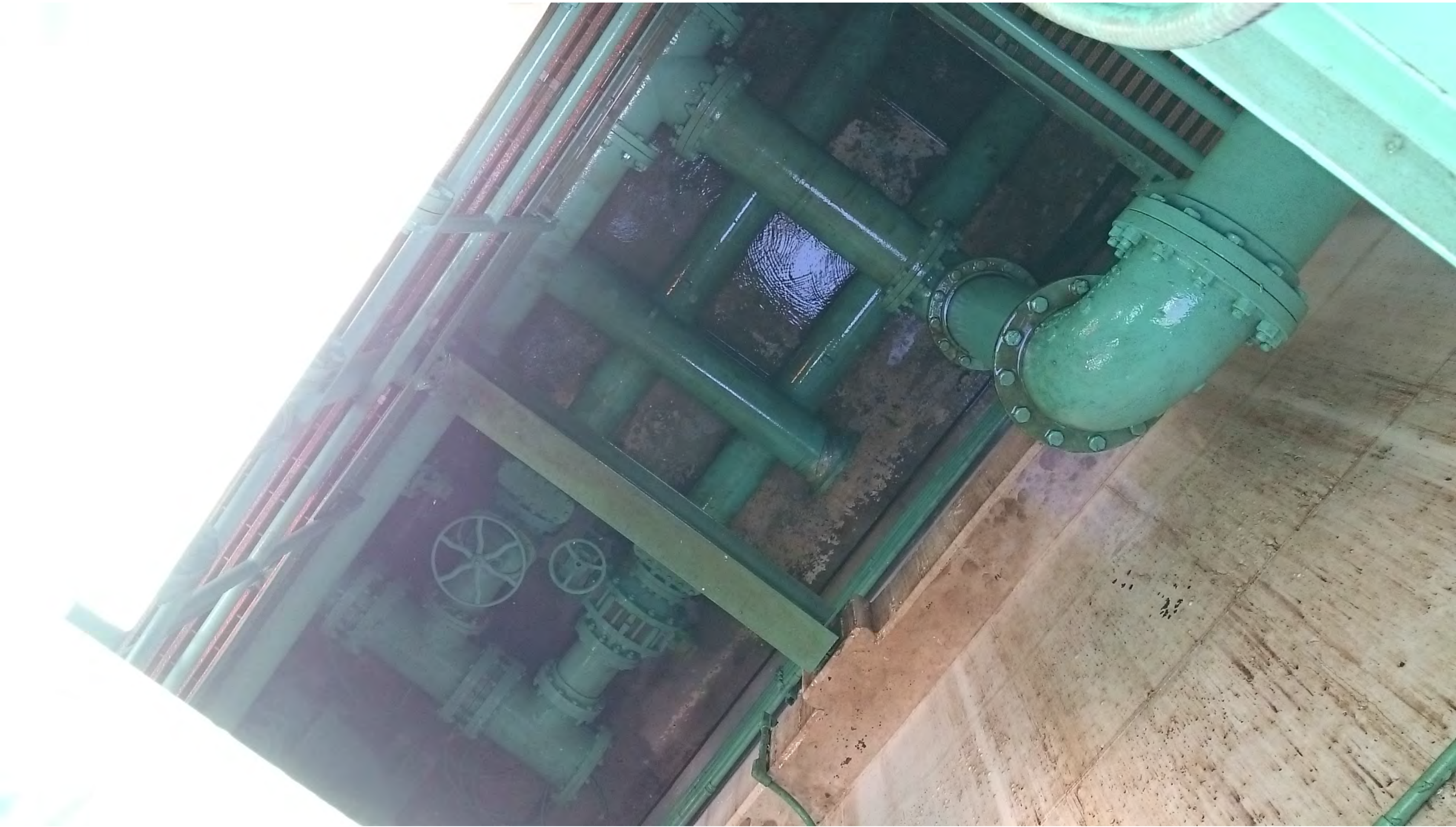
Details 1 and 2: Demolish and replace with new the filter in the above detail. Connect to existing valves and piping. The picture above and right shows the leaking filter (top view) to be replaced. Access is down a hatch and ladder.
