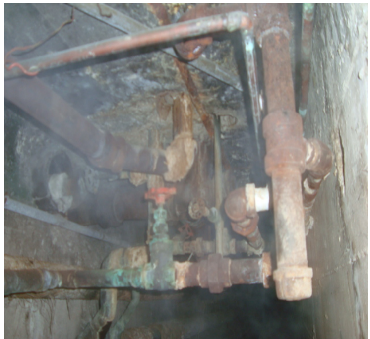
Typical Condensate Pipe connection to Take-off
