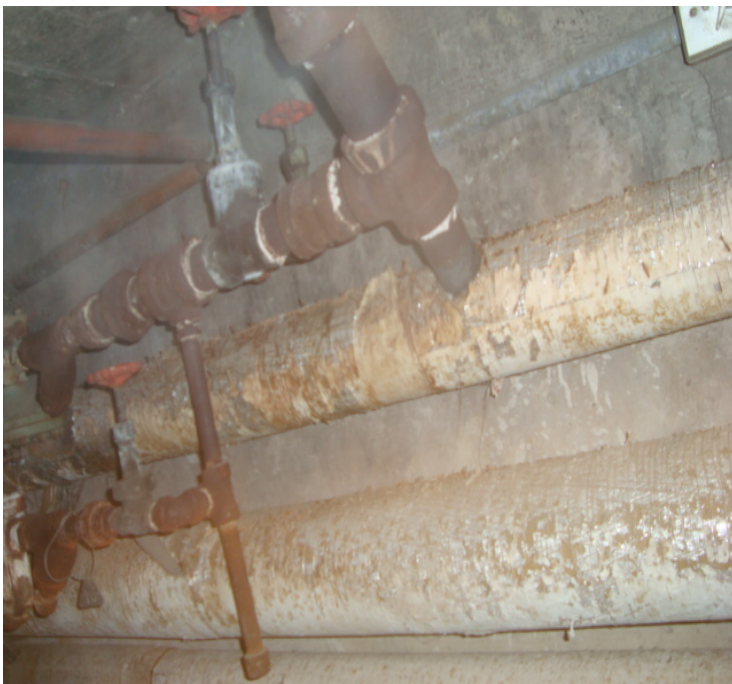
Typical Steam Pipe connection to Take-off
