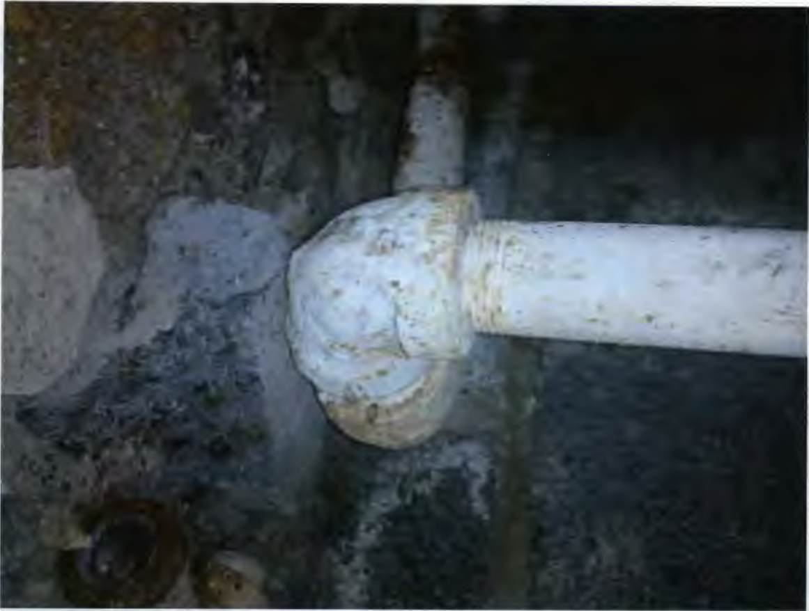
Residual asbestos joint packing on elbow
