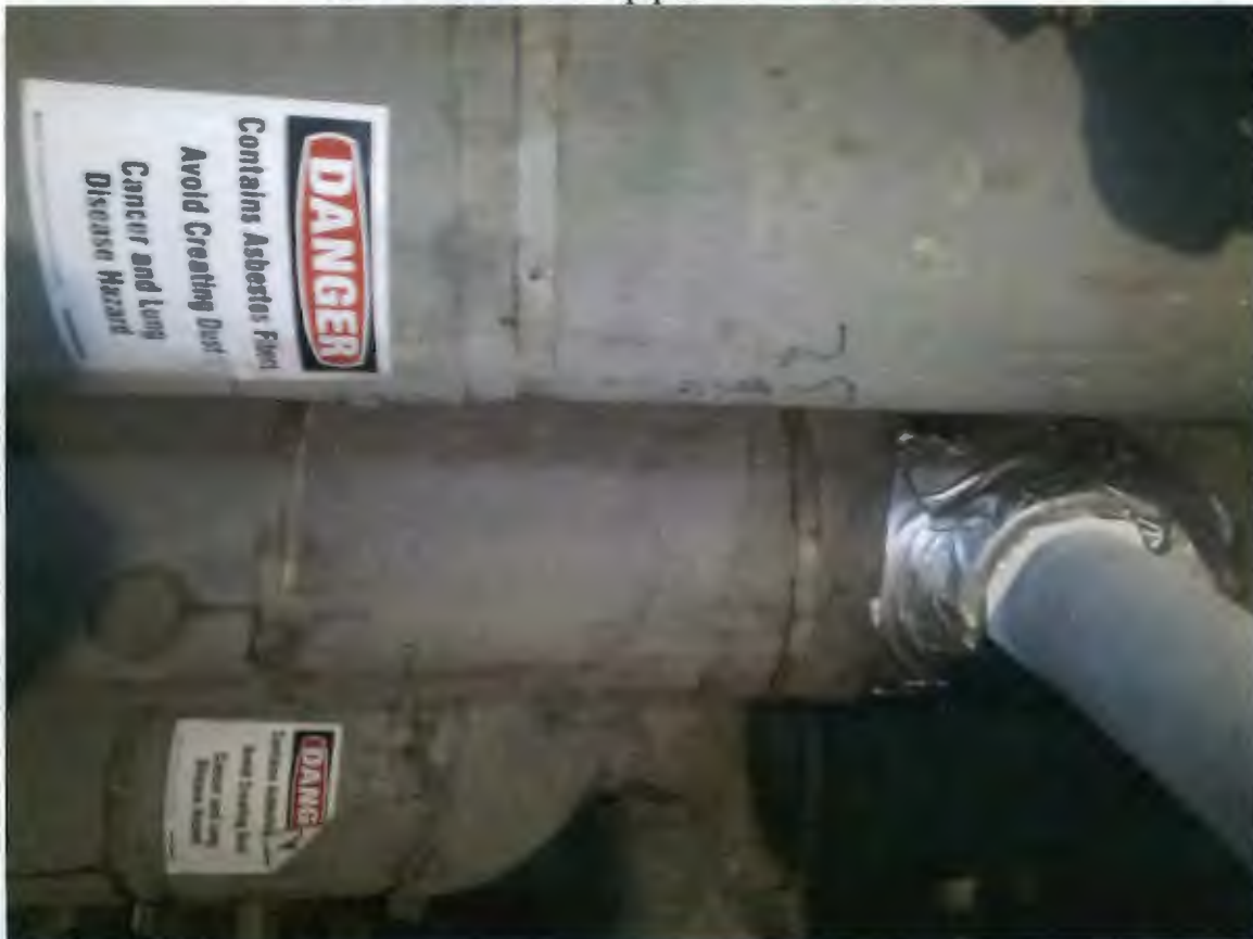
Improperly tied in pipe run in core pipe chase
