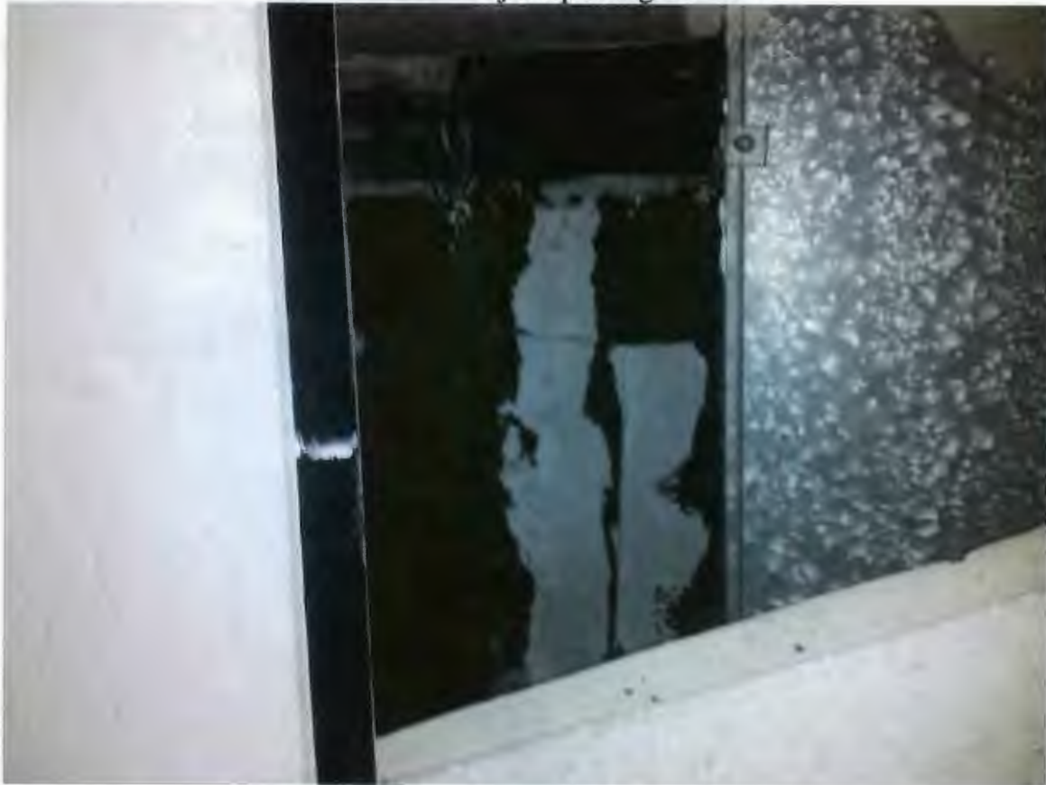
Asbestos containing seam patching on cork ductwork
