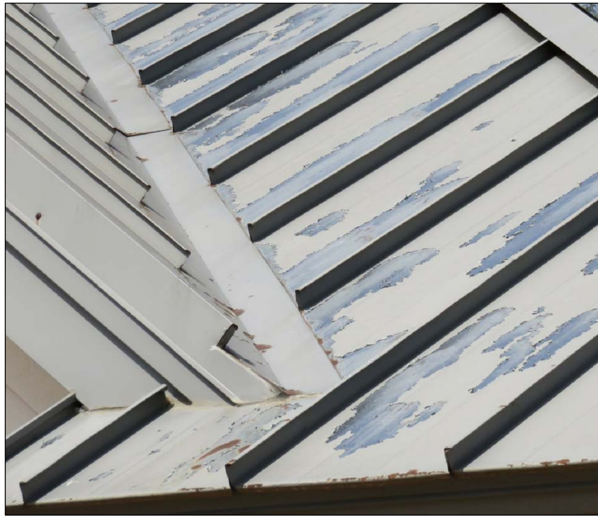
1D REFERENCE PHOTO L-2 EXISTING CONDITIONS - PEELING & FLAKING PAINT ON METAL ROOF PANELS
