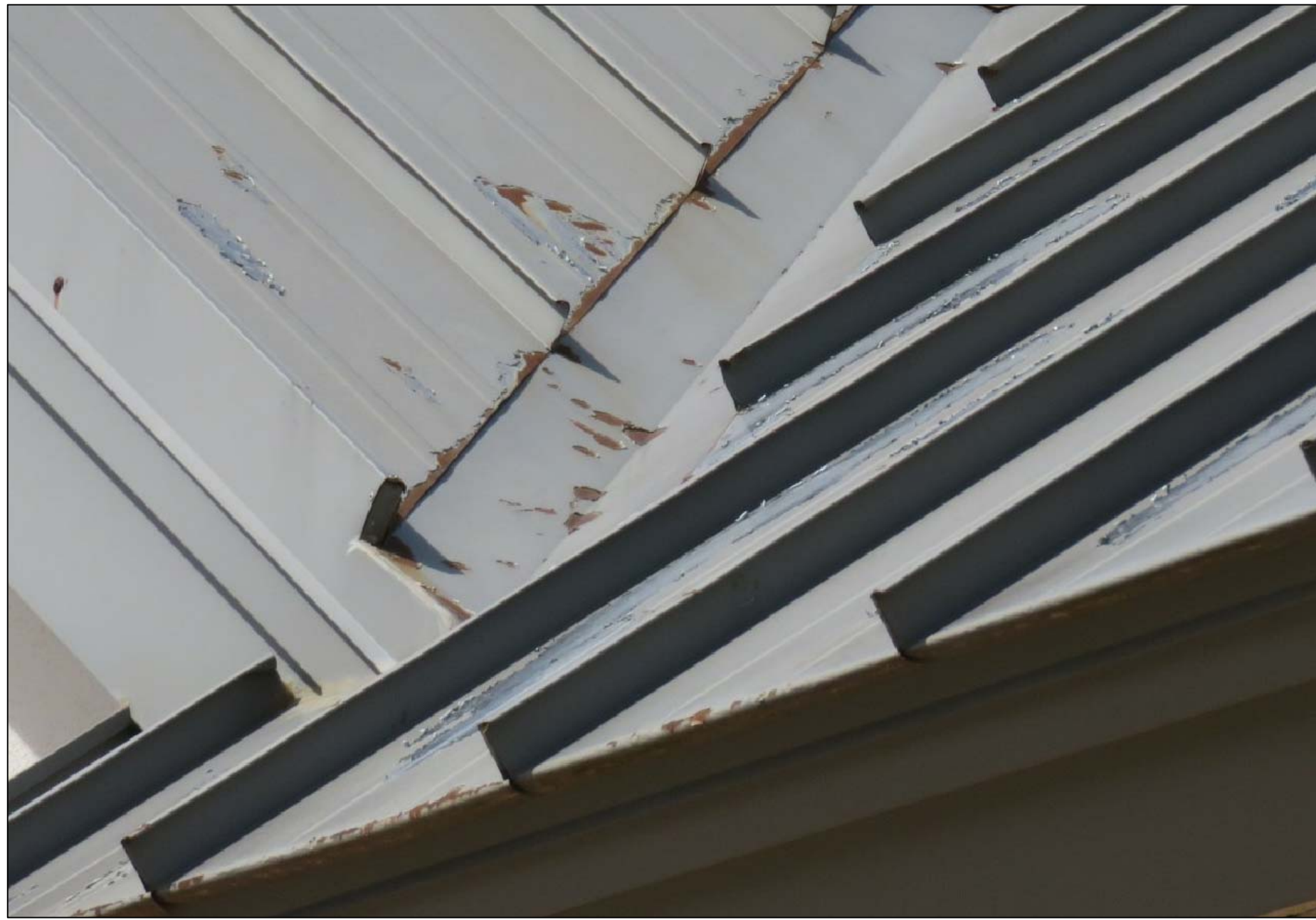
1B REFERENCE PHOTO L-2 EXISTING CONDITION - RUSTED AREAS ON METAL ROOF PANELS
