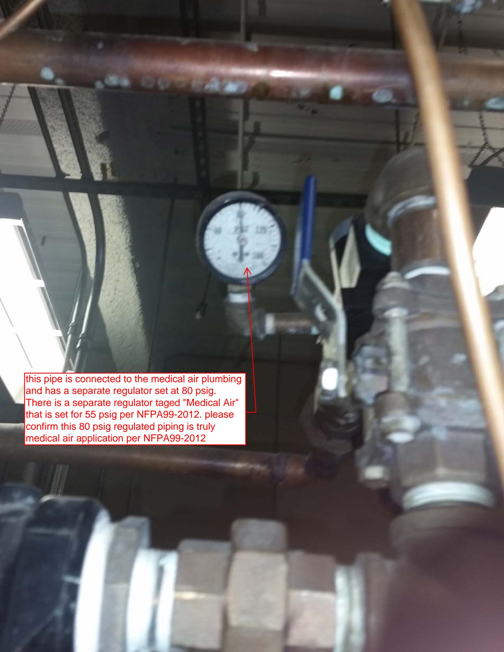
this pipe is connected to the medical air plumbing and has a separate regulator set at 80 psig. There is a separate regulator taged "Medical Air" that is set for 55 psig per NFPA99-2012. please confirm this 80 psig regulated piping is truly medical air application per NFPA99-2012
