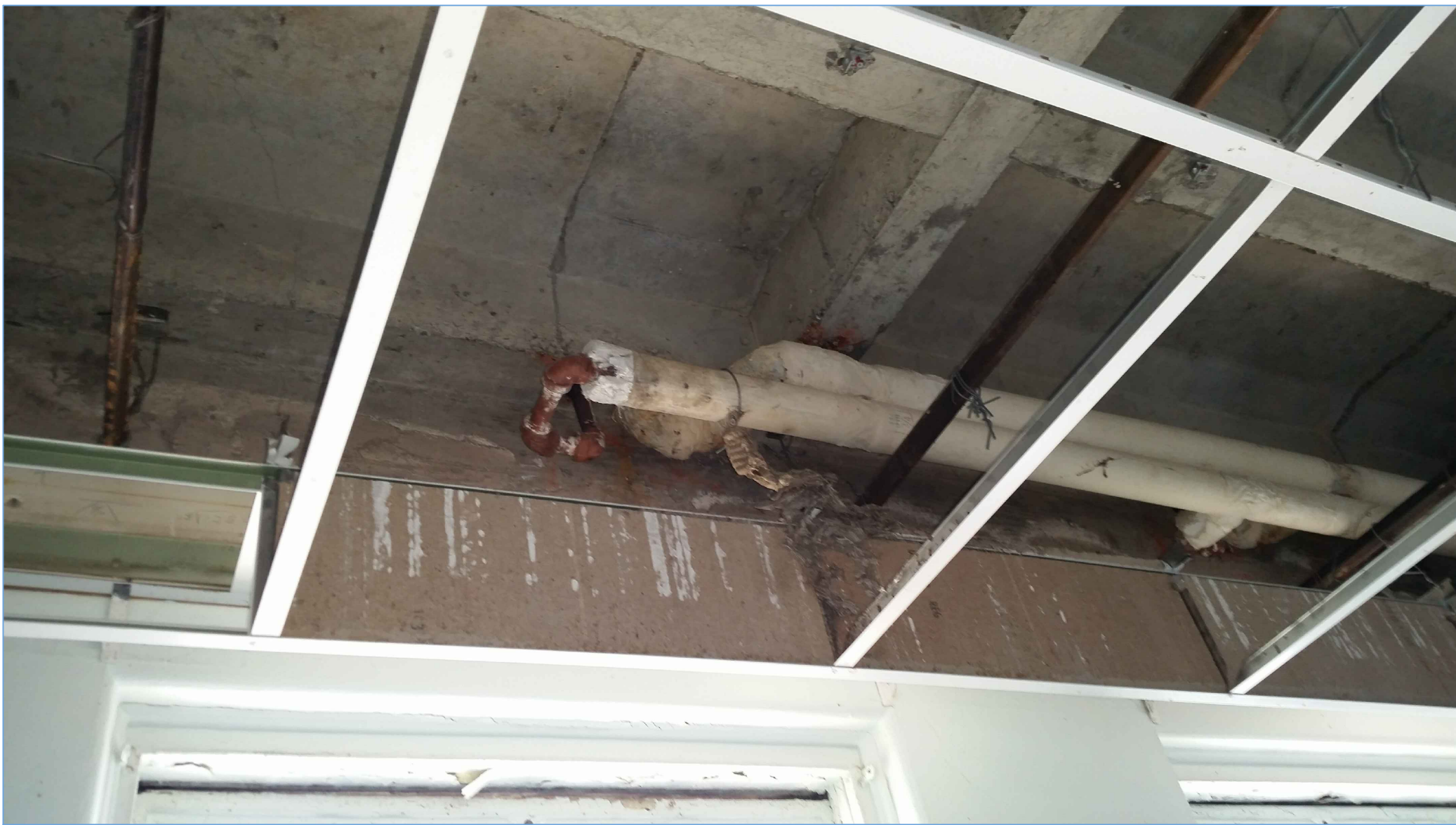
P3 NTS ACM PIPING SYSTEM ABOVE CEILING ON EXTERIOR WALL
