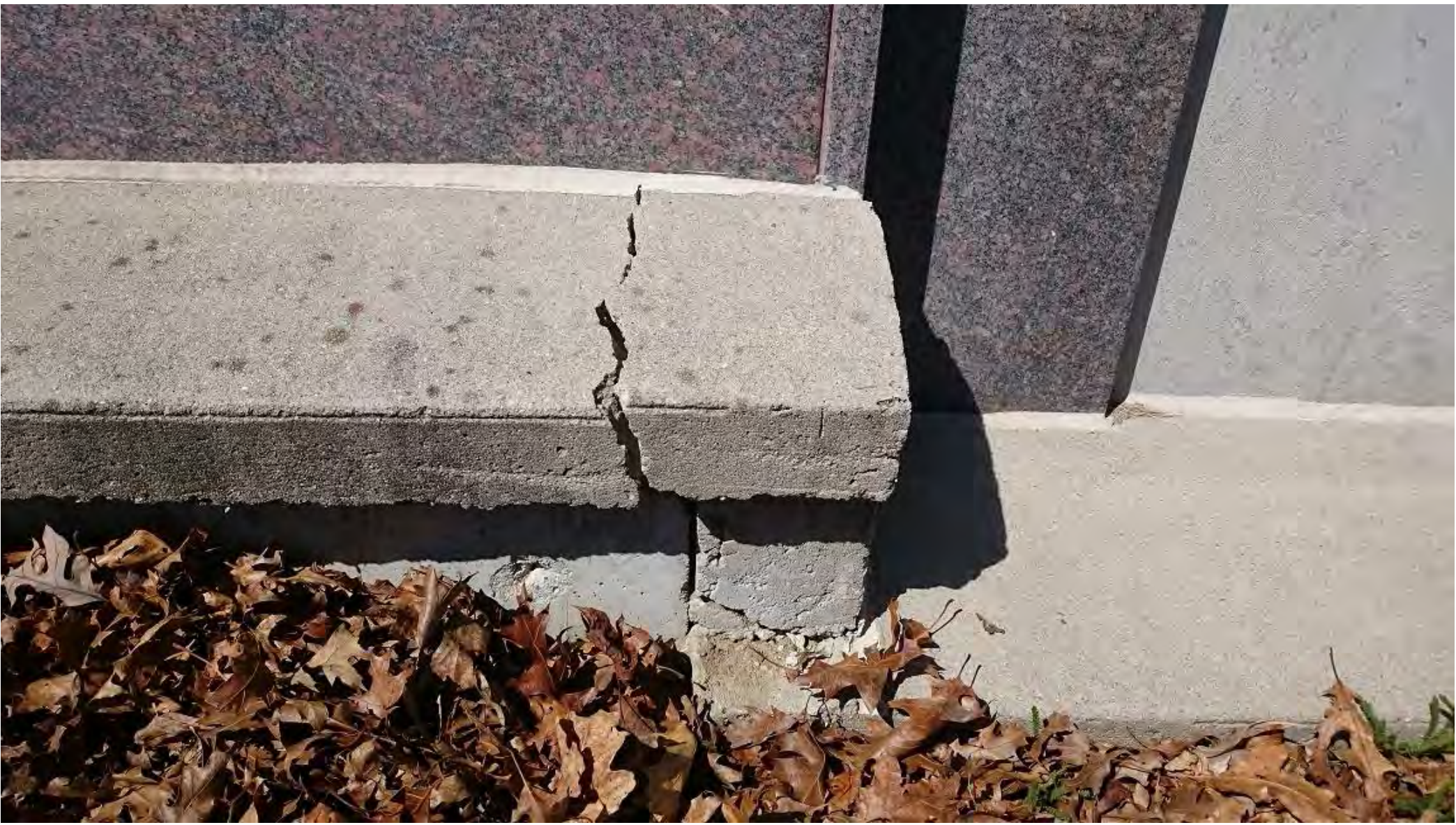
Detail 3: Demolish spalled concrete seen here, and reinstall. Dowel #4 rebar with epoxy into existing. Match color of existing. Caulk to match existing.
