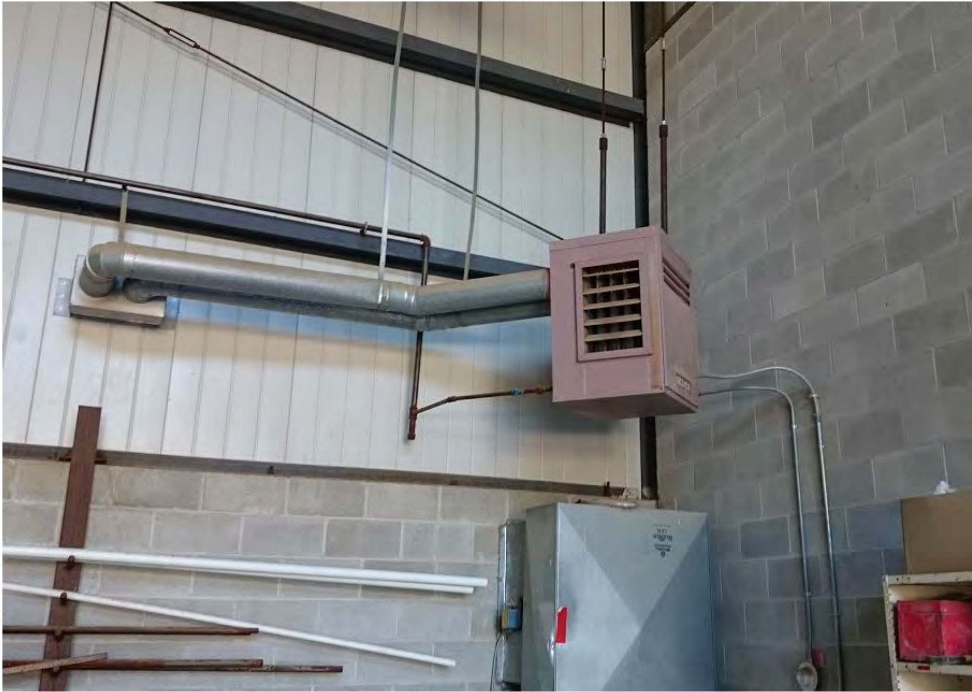
Detail 1: Demolish unit heater an all associated mechanical, electrical, and structural components.
