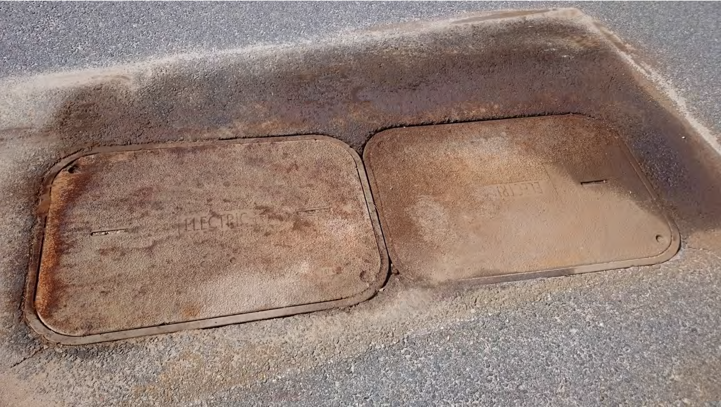
Detail 1: Remove existing electrical box covers and turn over to VA. Install new covers per specifications.
