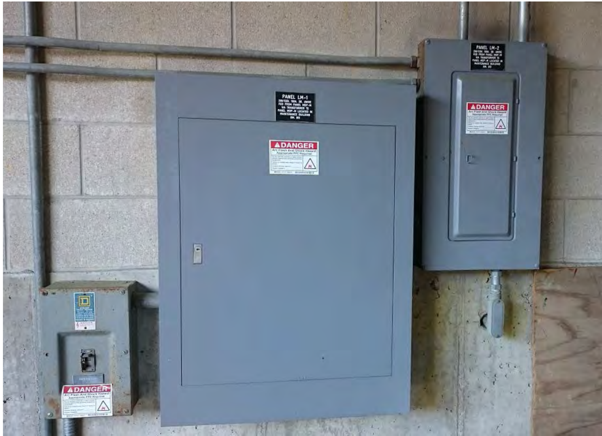
Detail 2. Project Engineer believes panel LM-2 is fed through LM-1. Contractor to verify and submit.
