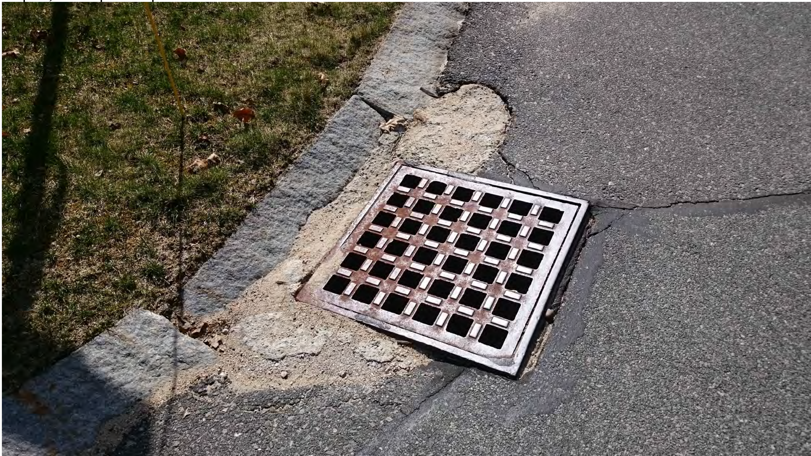
Detail 4 (above): Demolish failed manhole areas highlighted in red and replace with new. See specifications for more information. Note that precast concrete shall match the cast in place concrete specifications. Note also that existing manholes do not match this updated detail. Contractor shall bid for concrete and concrete block demolition work. New design build custom solution shall be enacted by the contractor which shall include a reinforced concrete solution per the design build detail. Detail 4 (below picture): Note typical failure which involves excavation, some concrete removal, infill, manhole/inlet repair, and asphalt repairs.
