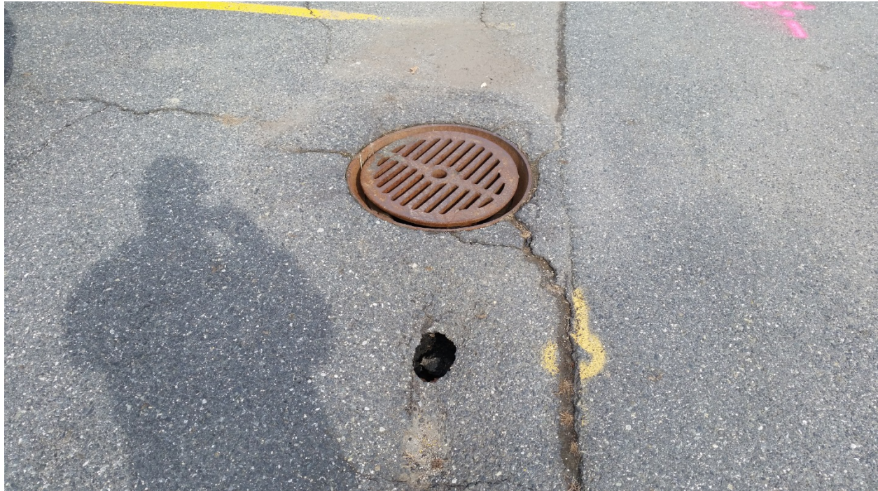
Photograph 2 – Cracking and Voids in Existing Parking Lot
