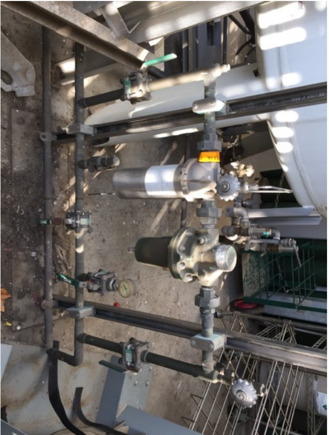
Pressure regulator, Output of Evaporator
