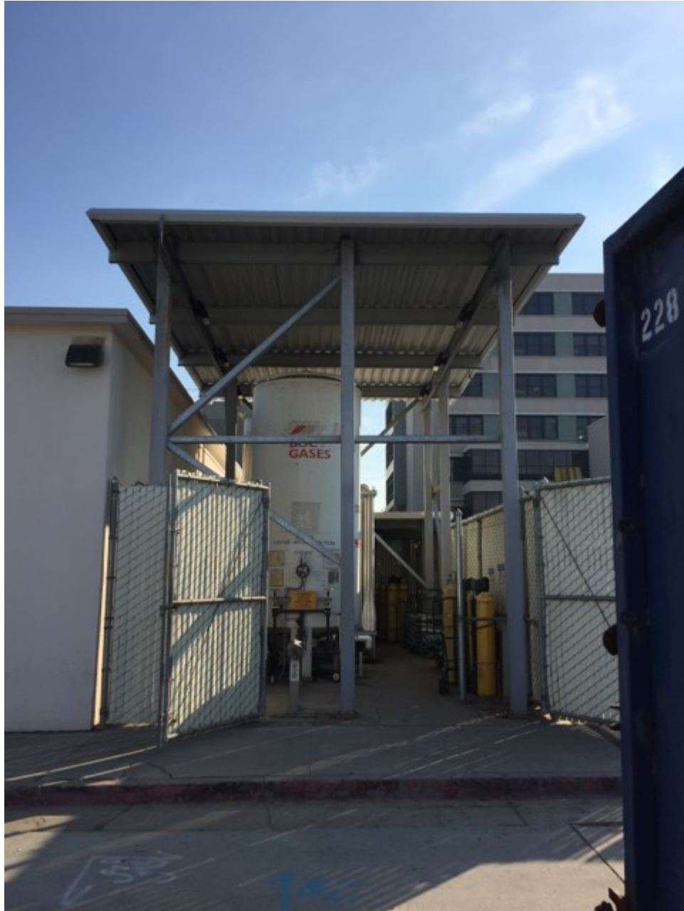
Liquid Oxygen Storage Area, North Side, Primary O2 Tank
