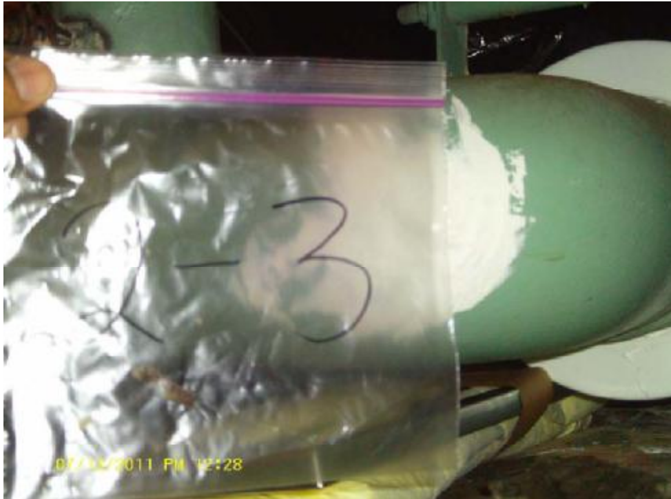
2-3 Joint insulation on green pipe 7% Chrysotile in dark brown sealant
