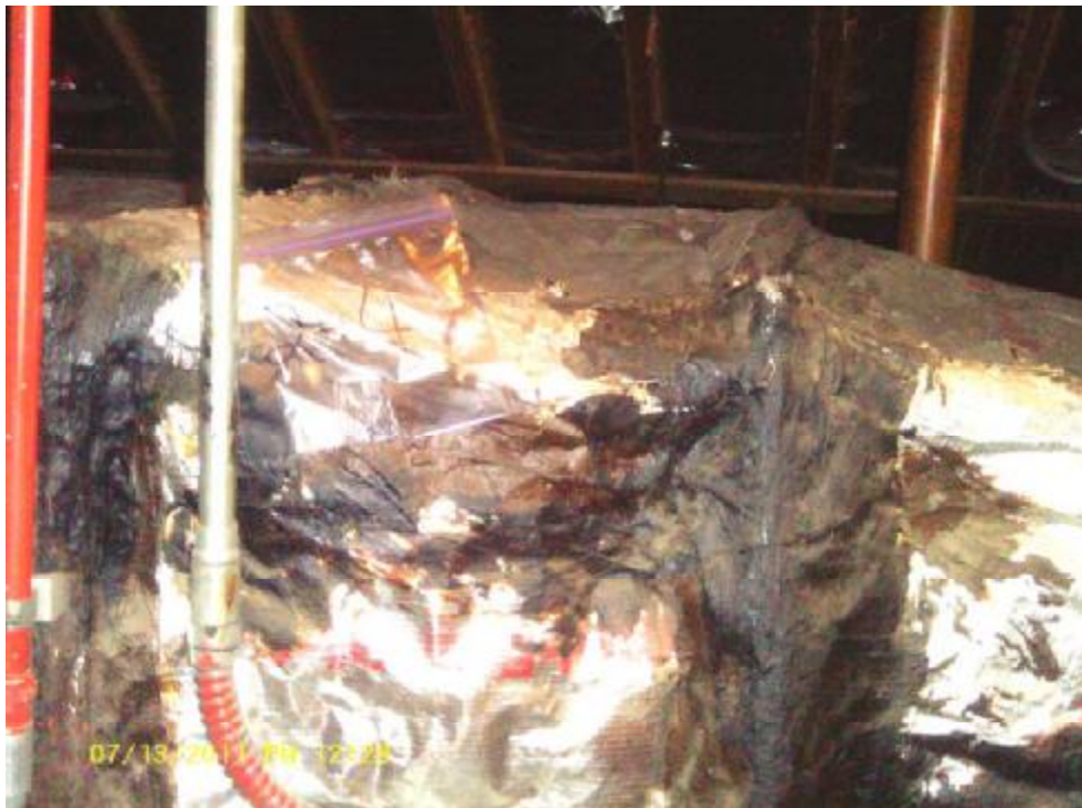
2-4 Mastic on square duct insulation – AHU 2 8% Chrysotile in dark brown sealant
