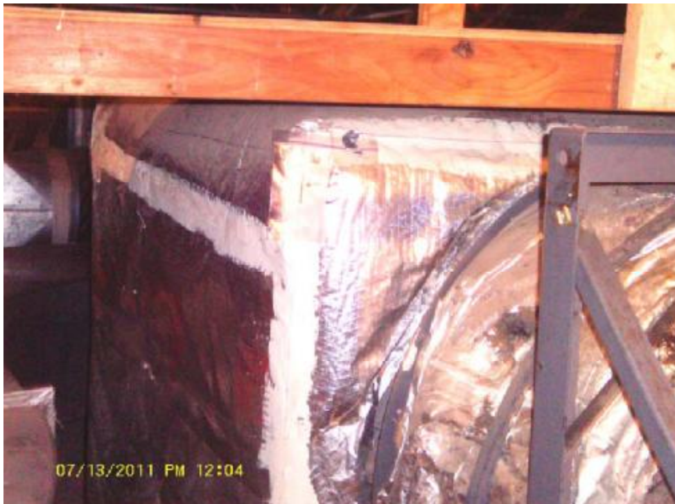
1-5 White mastic on AHU 1 duct – square None detected
