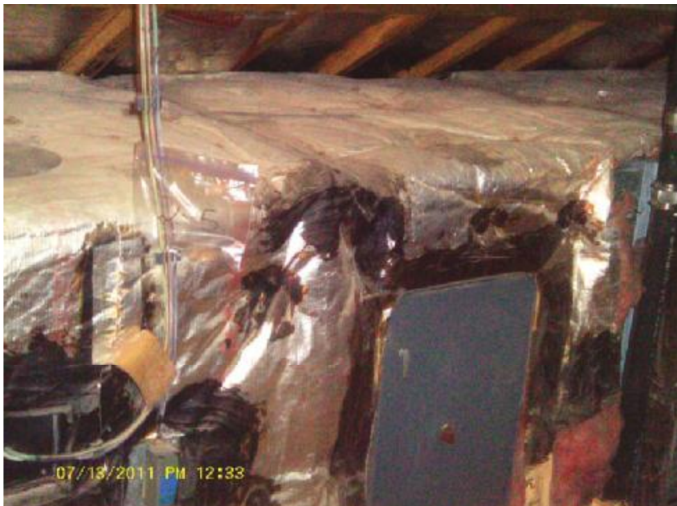
2-5 Mastic on square duct insulation – AHU 2 10% Chrysotile in dark brown sealant
