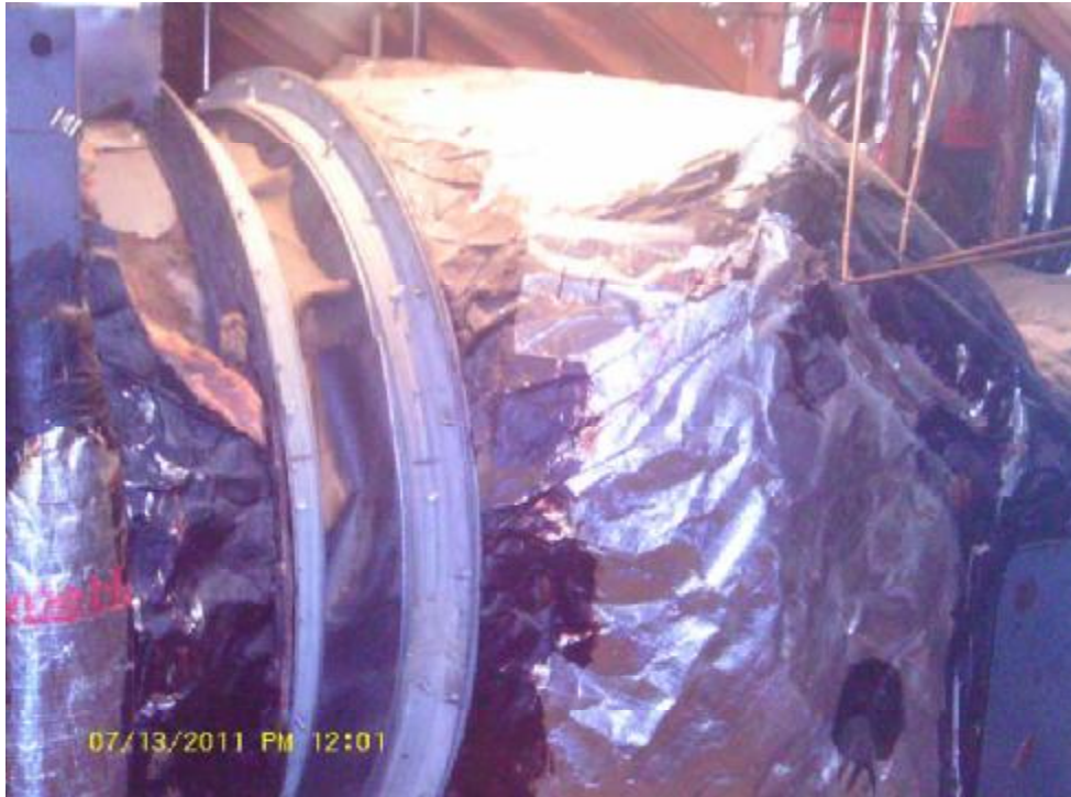
1-4 Black mastic on AHU 1 duct – round 5% Chrysotile in dark brown sealant
