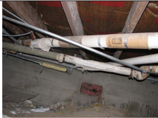
Photograph #1: Pipe insulation (assumed ACM) in crawlspace.
