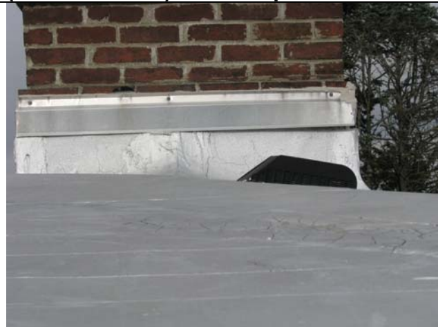
Photograph #3: Upper roof coating (Sample A-2).
