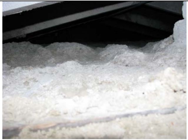
Photograph #2: Attic insulation (Sample A-1).
