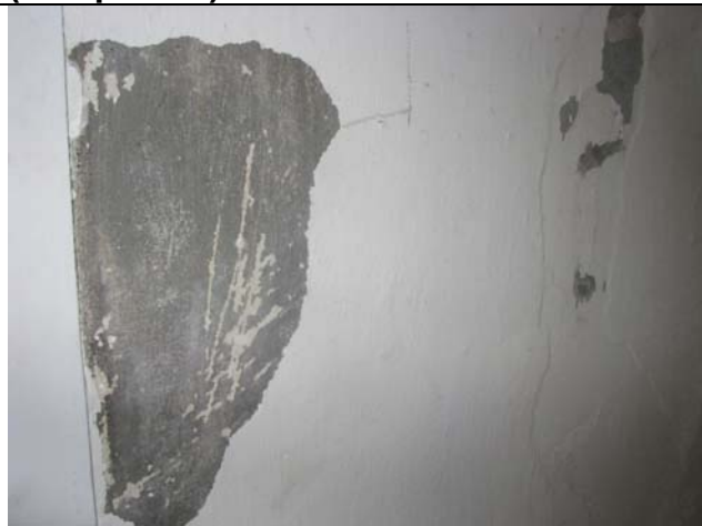
Photograph #9: Basement wall paint (Sample L-9).
