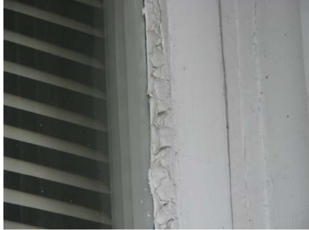
Photograph #7: Exterior window putty (Sample A-7).
