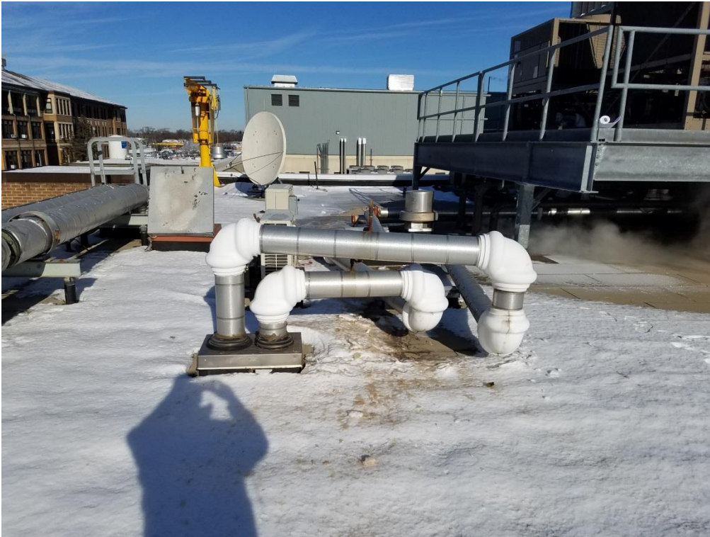
Roof top work site looking north
