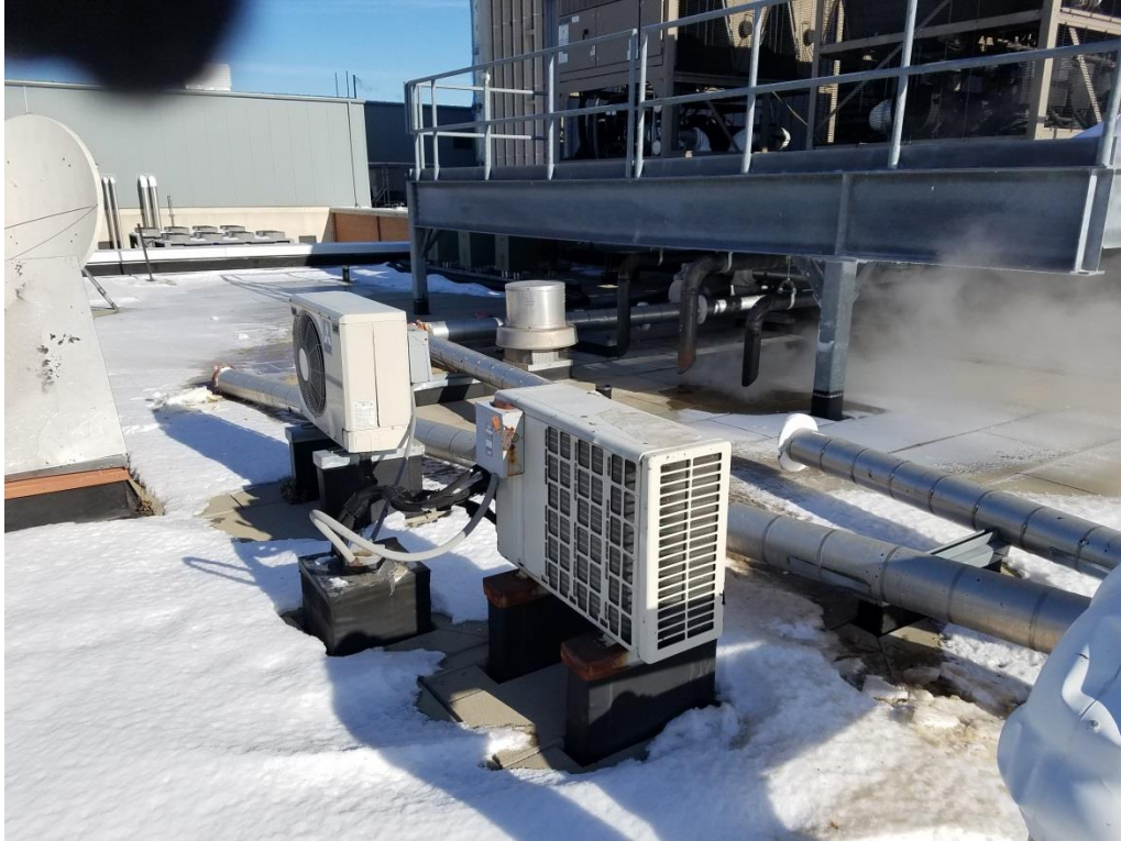
Roof top work site looking northeast
