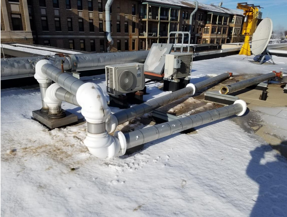
Roof top work site looking northwest
