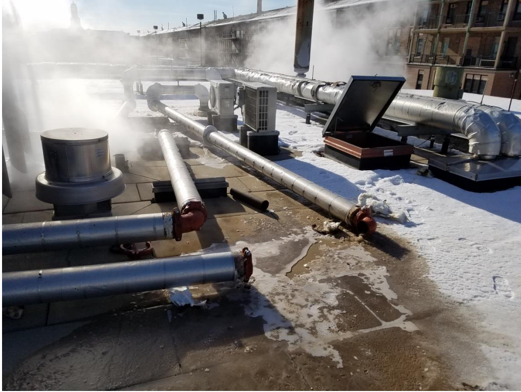
Roof top work site looking south
